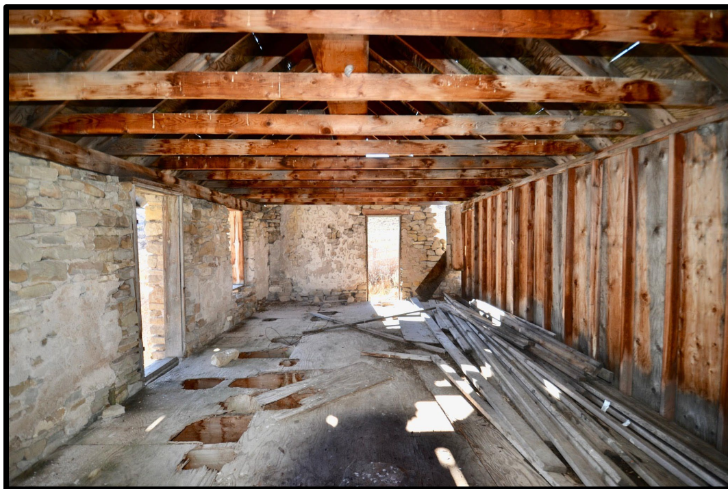
Photo 10: Interior of the Cabin, View to the South Current Photographs
