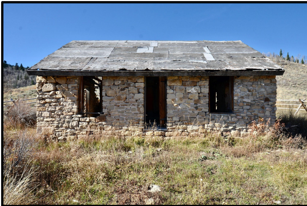
Photo 5: East Façade, View to the West
