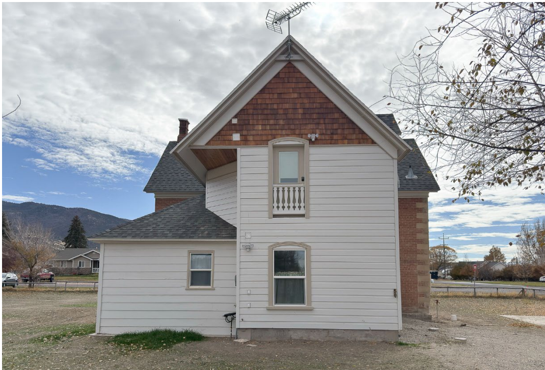
Photograph 8 North elevation of addition. Camera facing south.
