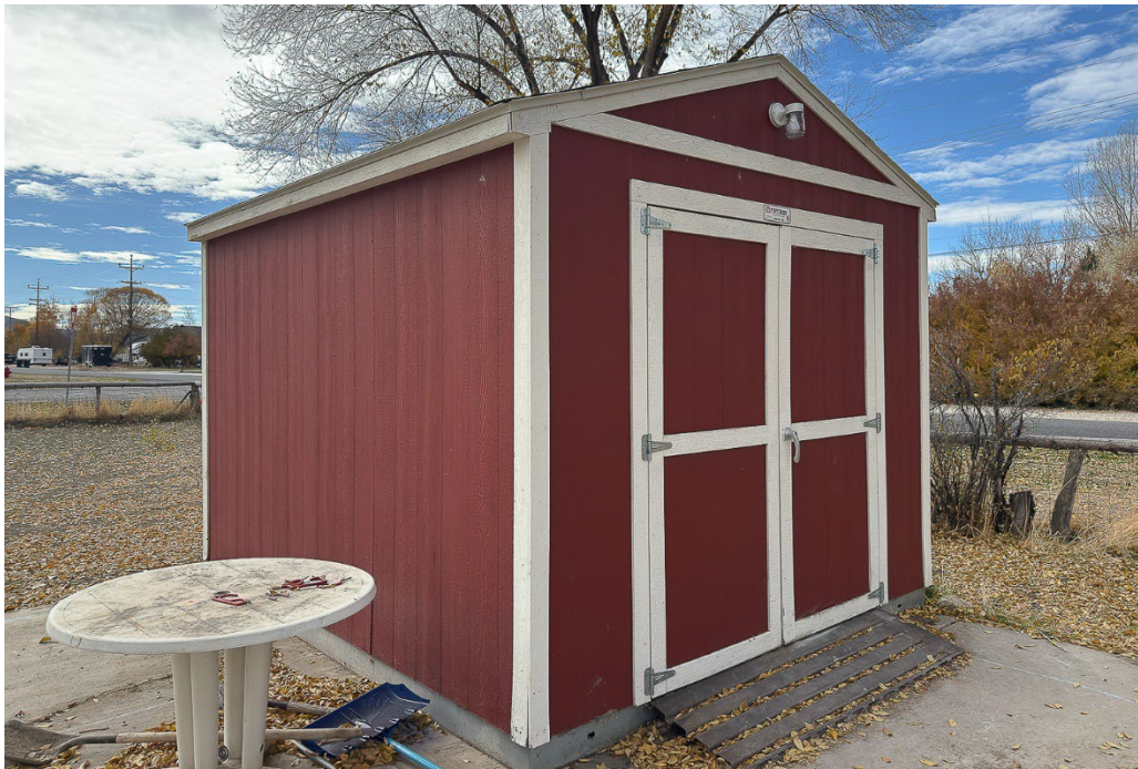
Photograph 16 Non-contributing prefabricated shed. Camera facing southwest.
