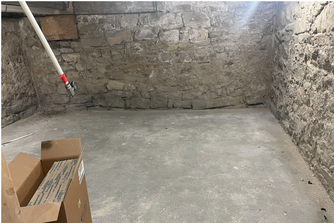
Photograph 13 Interior, basement. Camera facing east.
