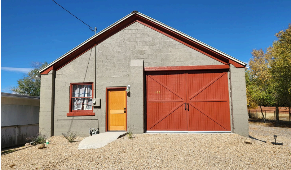
Photo 1 of 10. South elevation. Camera facing north.
