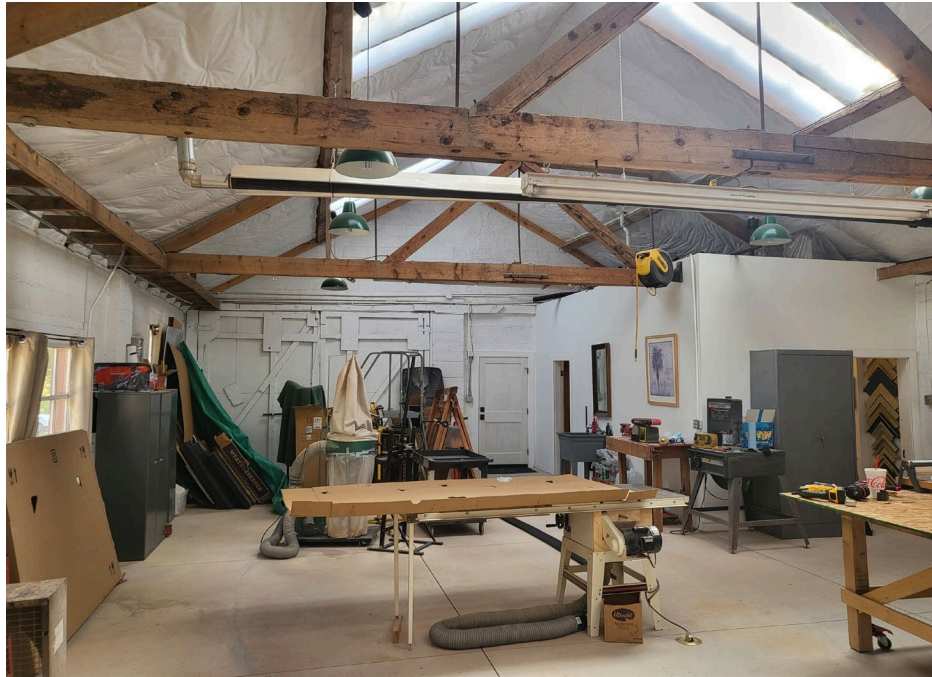
Photo 7 of 10. Frame/wood shop. Camera facing south. Restroom/storage enclosure on the right.
