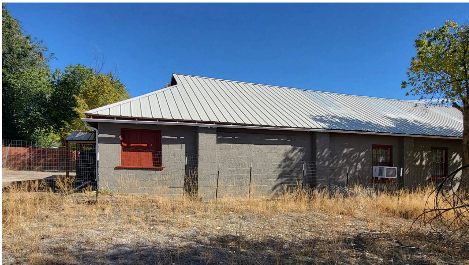
Photo 4 of 10. West elevation. Camera facing east.
