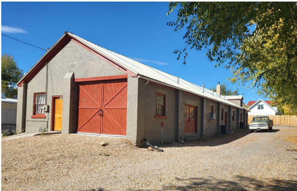
Photo 2 of 10. Southeast corner. Camera facing northwest.
