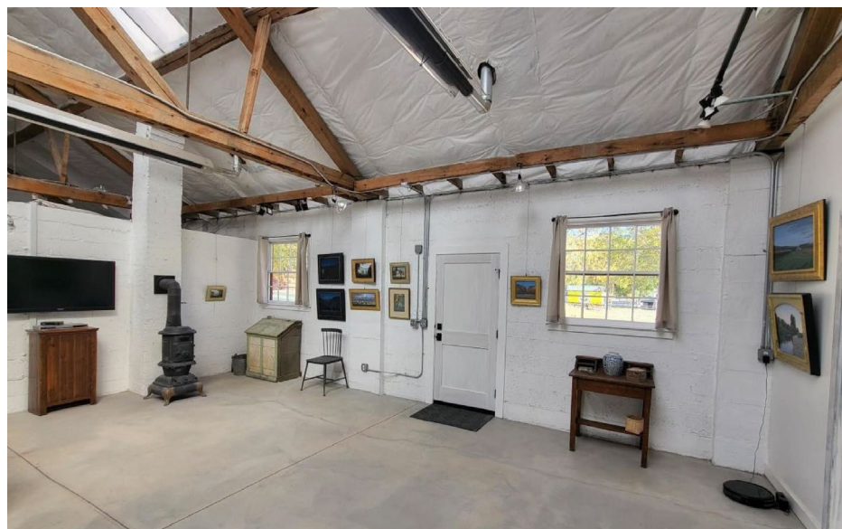
Photo 8 of 10. Art studio. Camera facing east/northeast.
