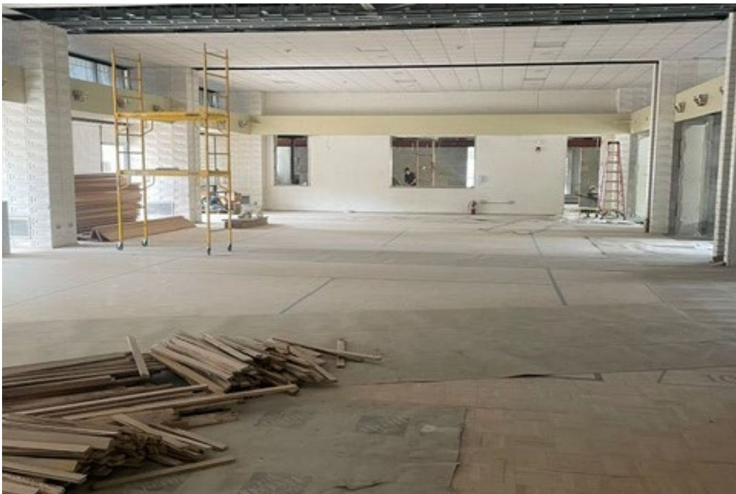
Photograph 30 Multipurpose room mid-construction with view of the kitchen. Camera facing south.
