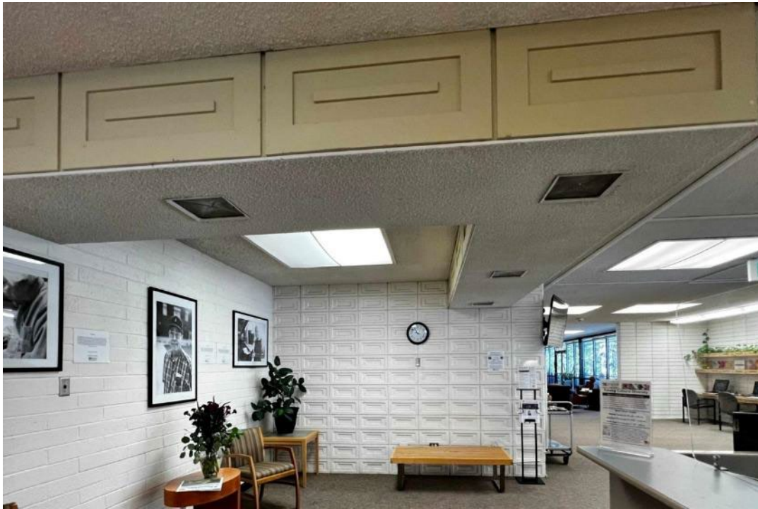
Figure 3 Front lobby pre-construction | July 11, 2023 | Ali Smith of Nexus Architecture
