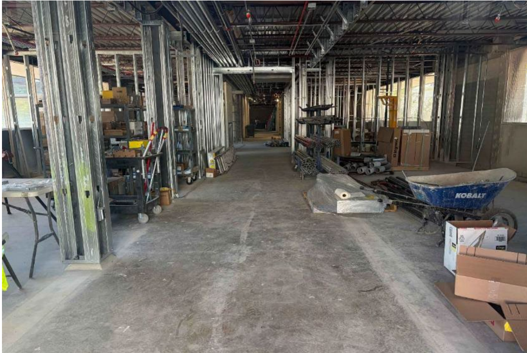
Photograph 31 Activity hallway mid-construction. Camera facing west.
