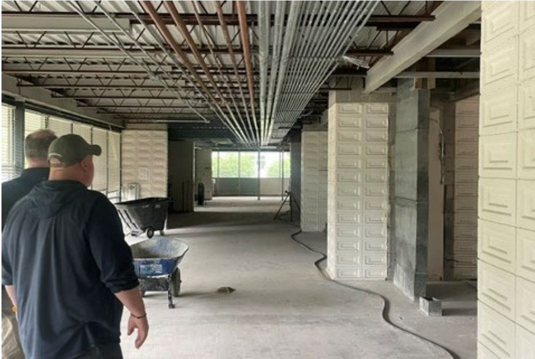
Photograph 29 Social commons mid-construction. Camera facing north.
