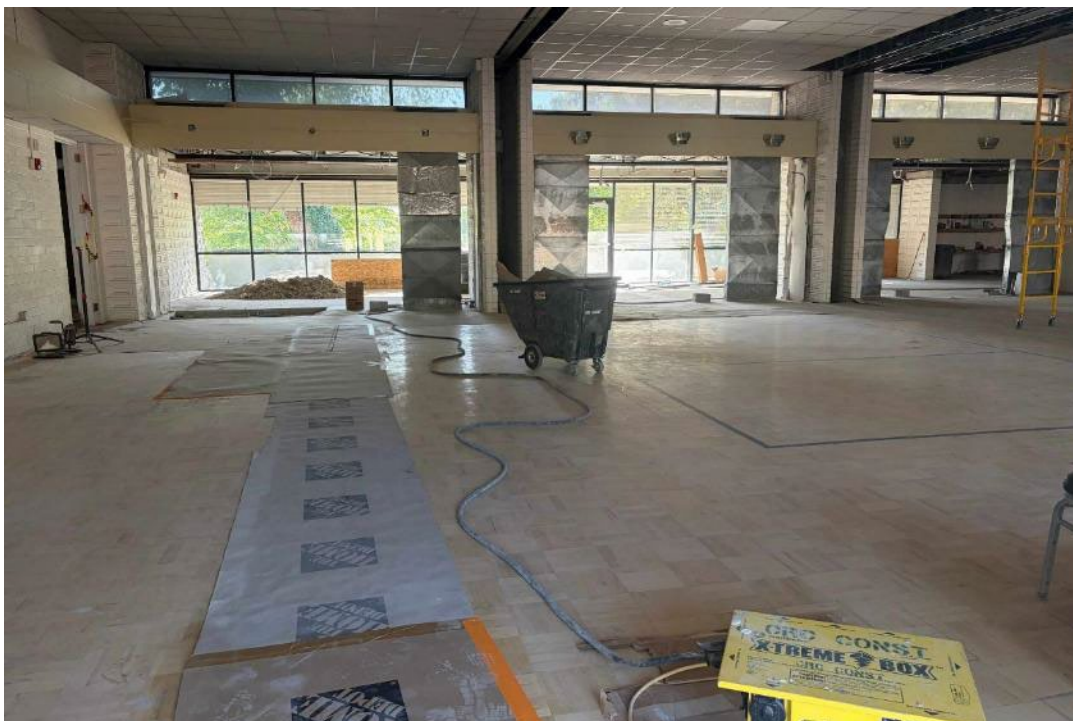
Photograph 32 Multipurpose room and clerestory windows. Camera facing west.
