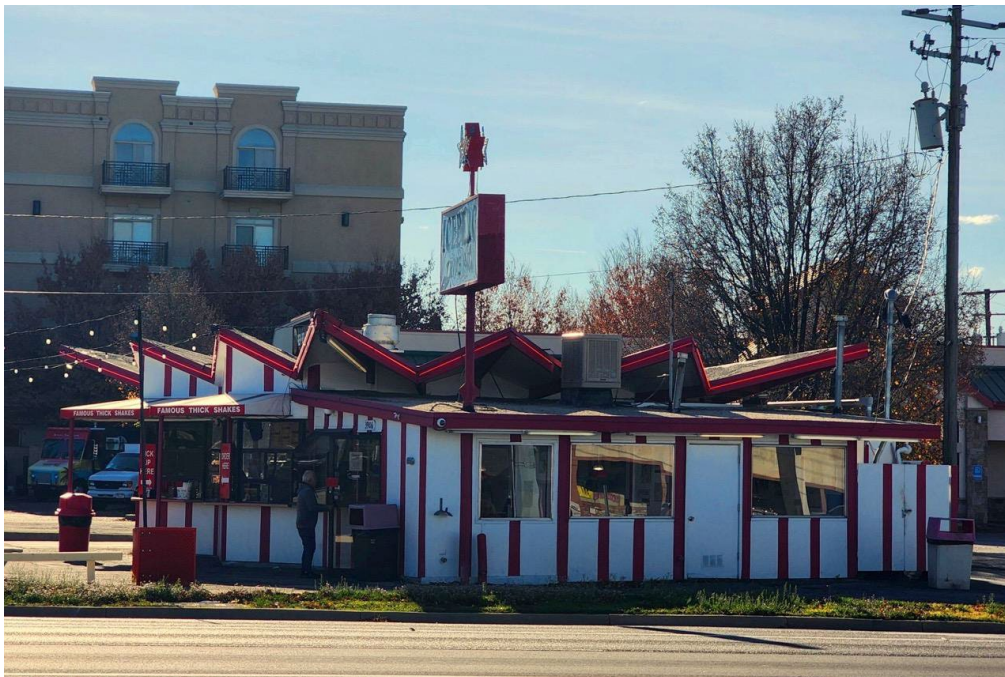
Photograph 2. Exterior, north façade. Camera facing southwest.
