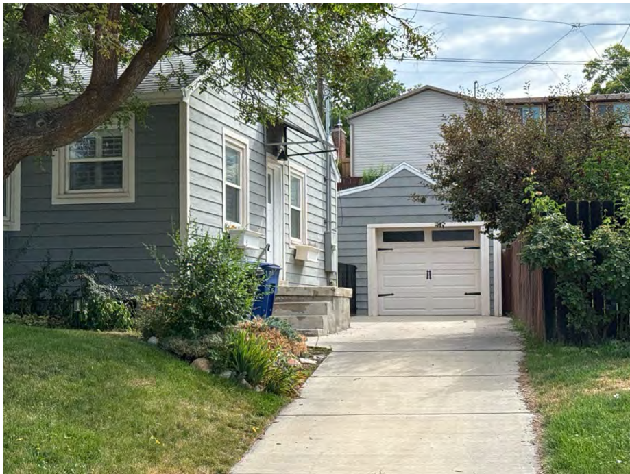
Photograph 48. 2819 S. Wainwright Dr. The main residence is contributing to the Historic District, and the garage unit is a contributing structure. Camera facing east.
