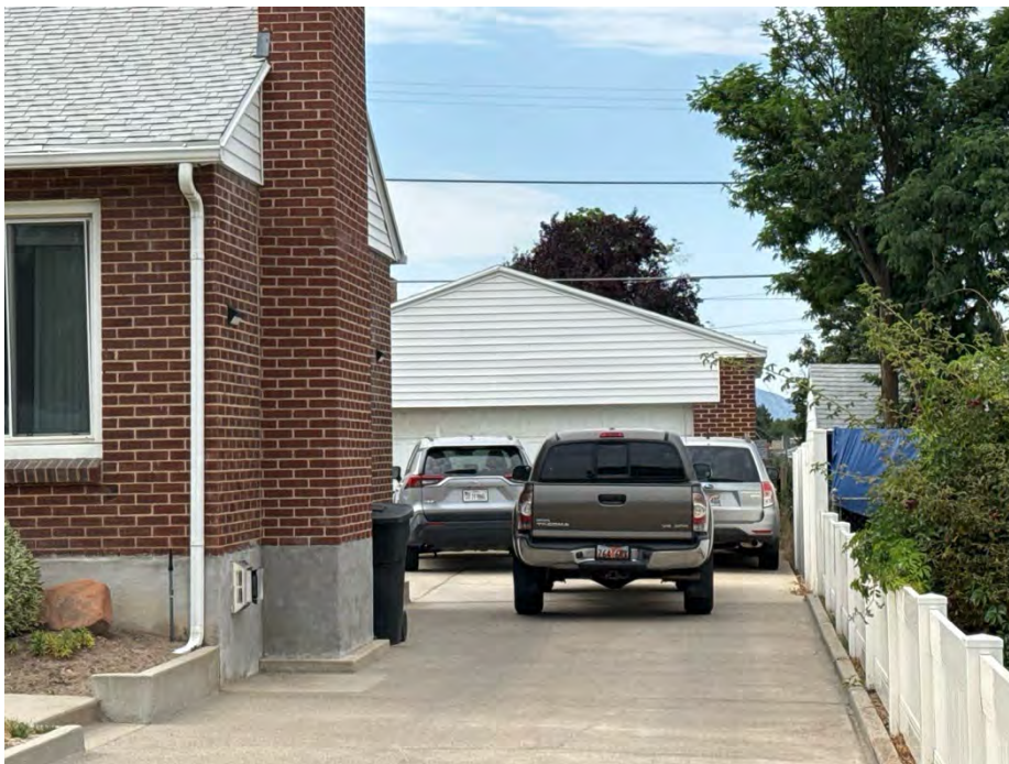
Photograph 46. 2540 E. 2900 S. The main residence is contributing to the Historic District, and the garage unit is a contributing structure. Camera facing south.
