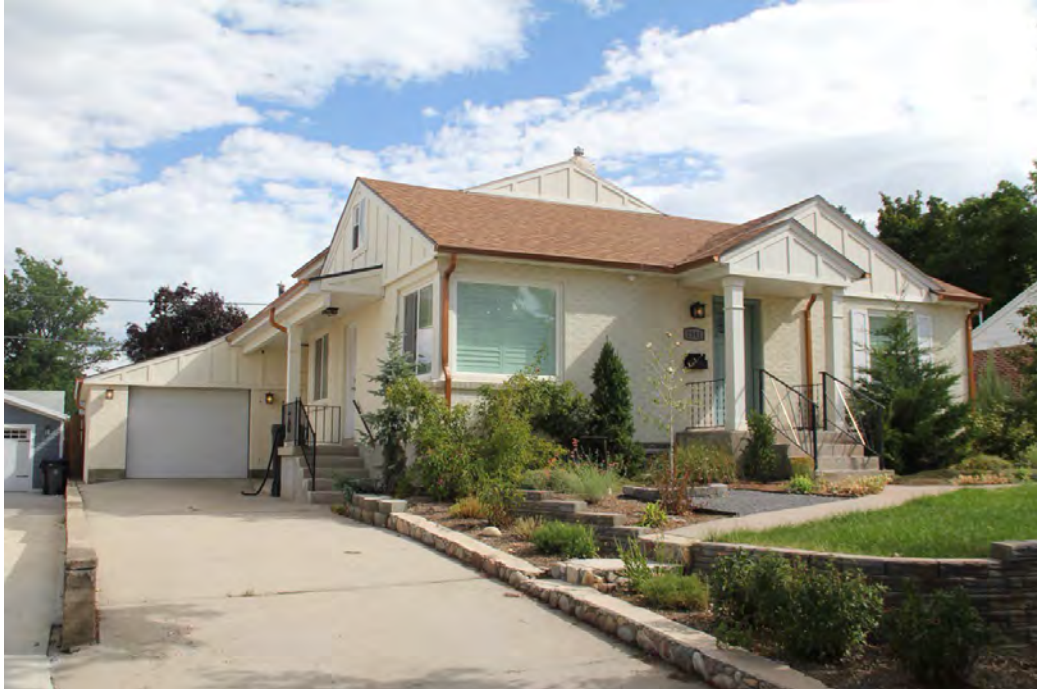
Photograph 41. 2541 E. 2940 S. Camera facing north. This building is non-contributing within the Historic District.
