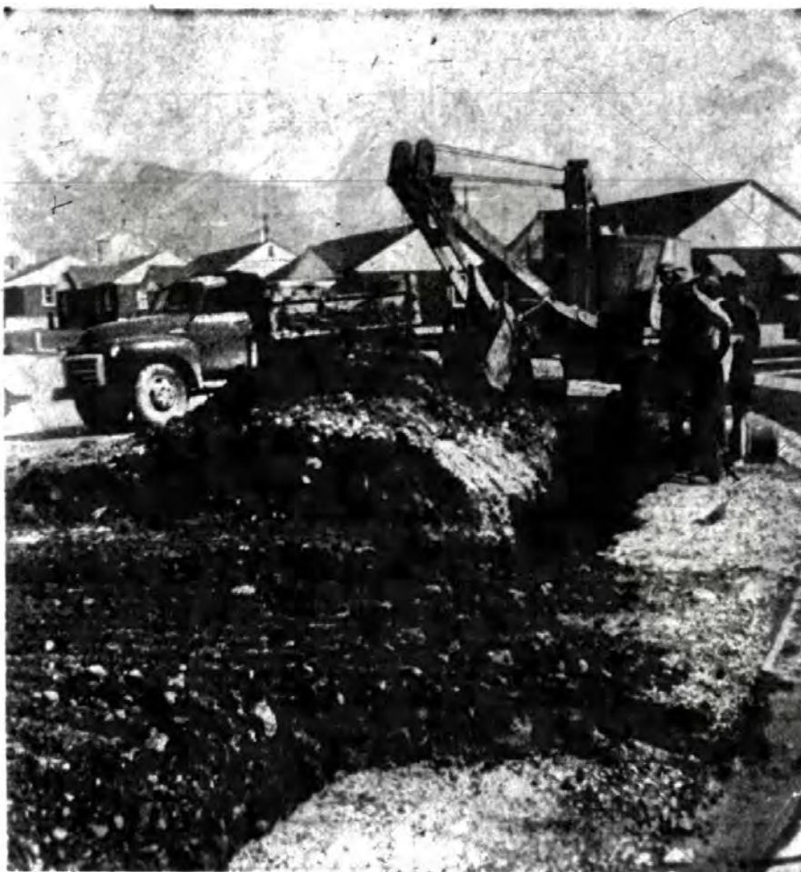
Work on the long-sought drainage project in the Veterans Heights area is well under way and "progressing nicely," County Commissioner Lamont B. Gunderson reported Thursday.
