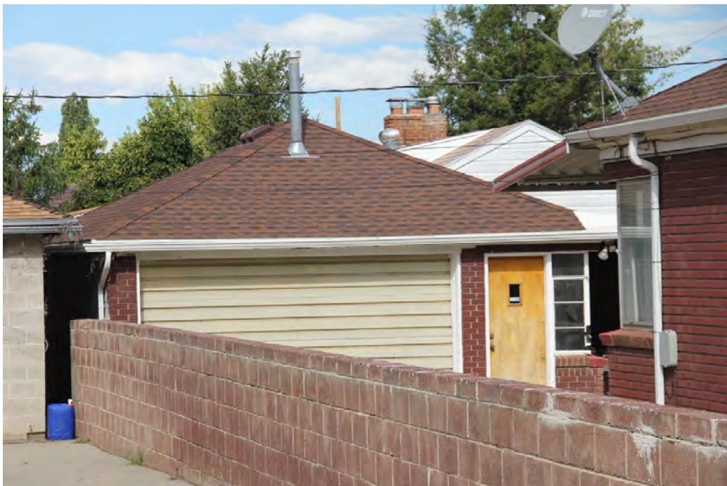
Photograph 42. 2768 S. 2700 E. Detached, contributing garage. Camera facing west. The building is contributing to the Historic District.
