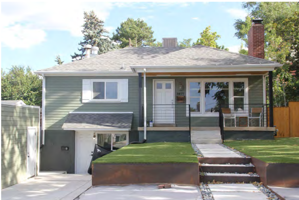
Photograph 18. 2677 E. 2900 S. Camera facing north. This building is non-contributing within the Historic District.
