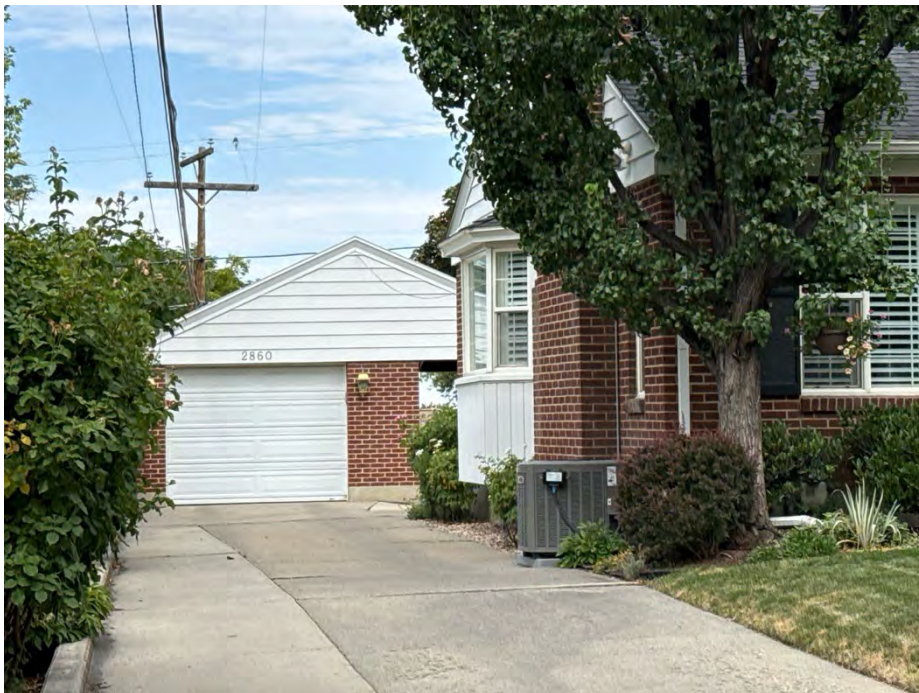
Photograph 52. 2860 S. Devereaux Way. The main residence is contributing to the Historic District, and the garage unit is a non-contributing structure. Camera facing west.
