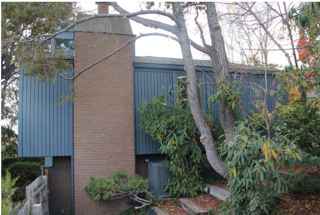
Photograph 6. Exterior, east façade. Camera facing west.
