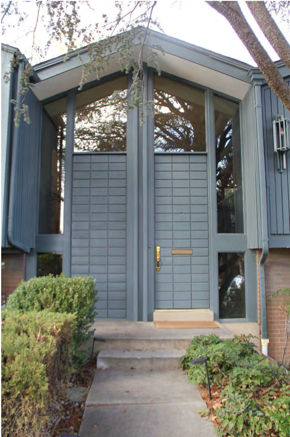
Photograph 13. Exterior, south (main) façade showing dummy leaf door, and trapezoidal transoms. Camera facing north.
