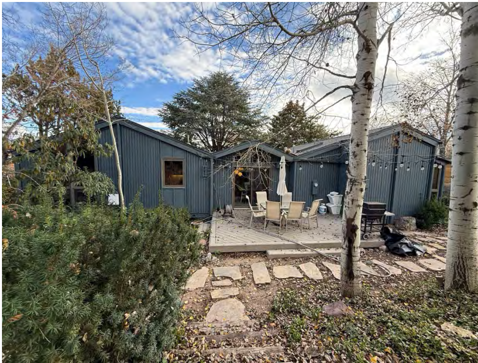
Photograph 9. Exterior, north façade. Camera facing south.
