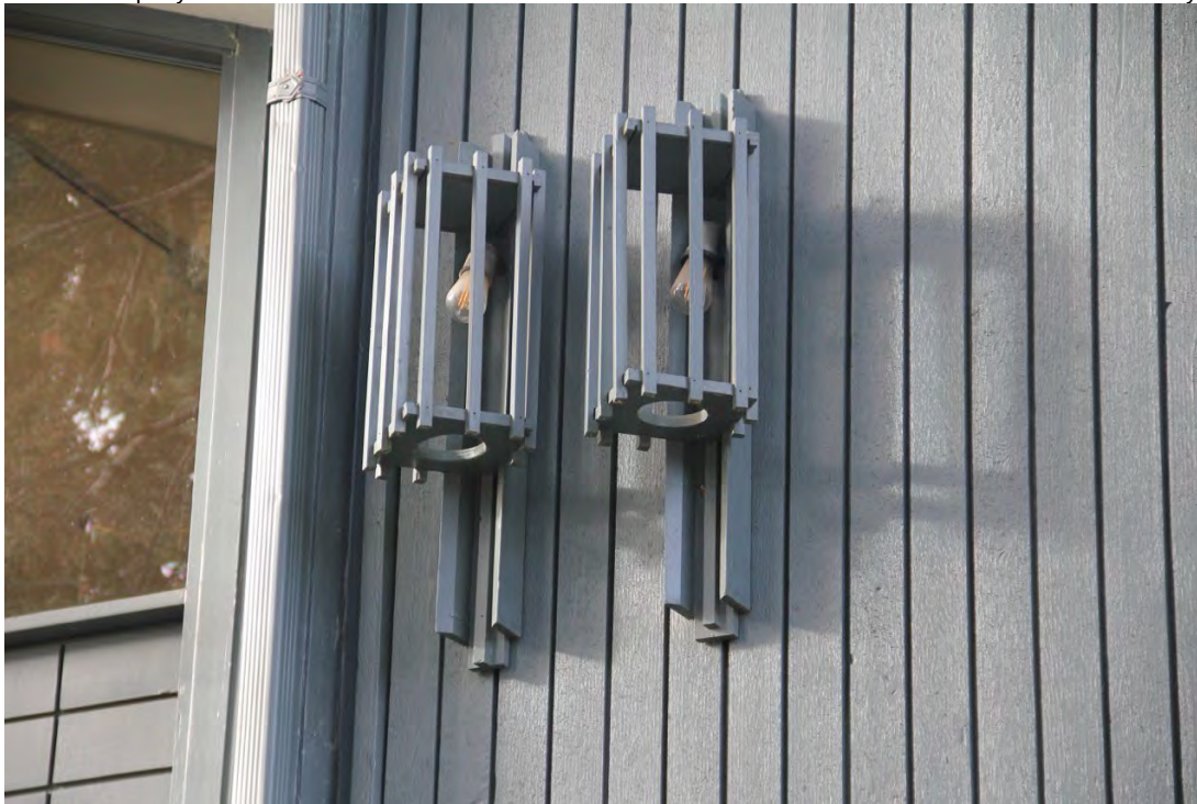
Photograph 14. Exterior, south (main) façade showing custom wood sconces for exterior lights. Camera facing north.
