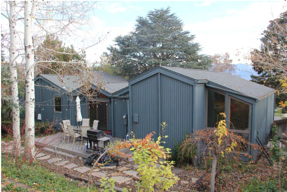
Photograph 10. Exterior, north façade. Camera facing southeast.
