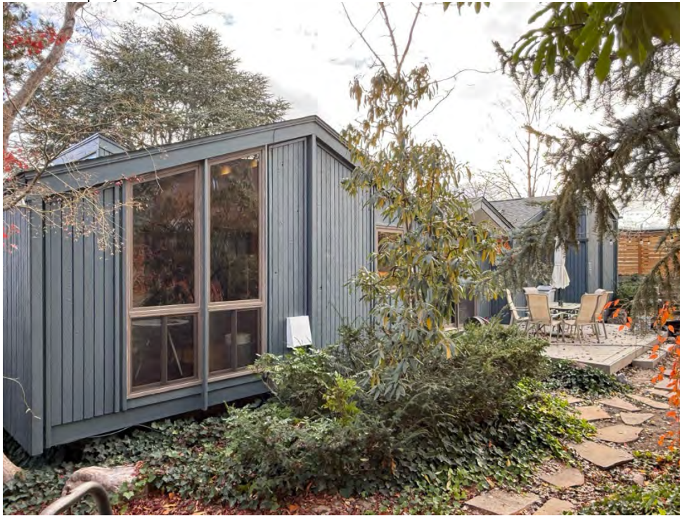
Photograph 8. Exterior, north façade. Camera facing southwest.
