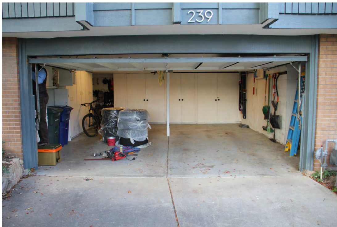
Photograph 38. Interior, garage area. Camera facing north.
