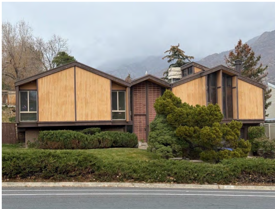
Figure 7. 3637 E Bengal Blvd in Salt Lake City was built in 1973. Photo taken in 2025. Credit: Kirk Huffaker.
