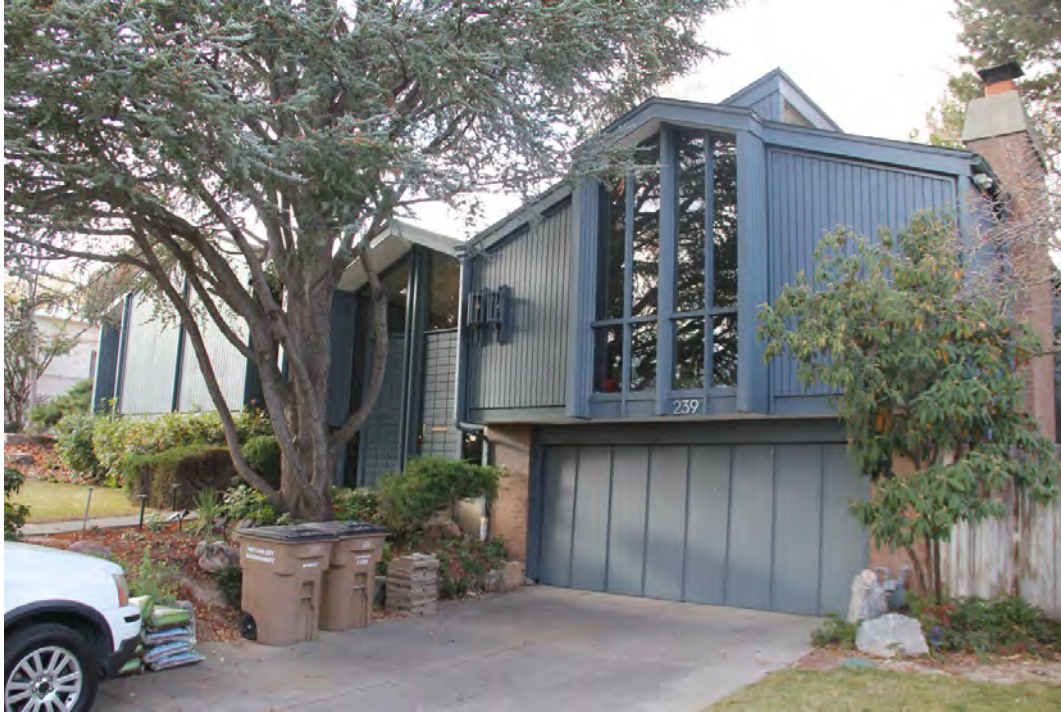
Photograph 1. Exterior, south (main) façade. Camera facing northwest.
