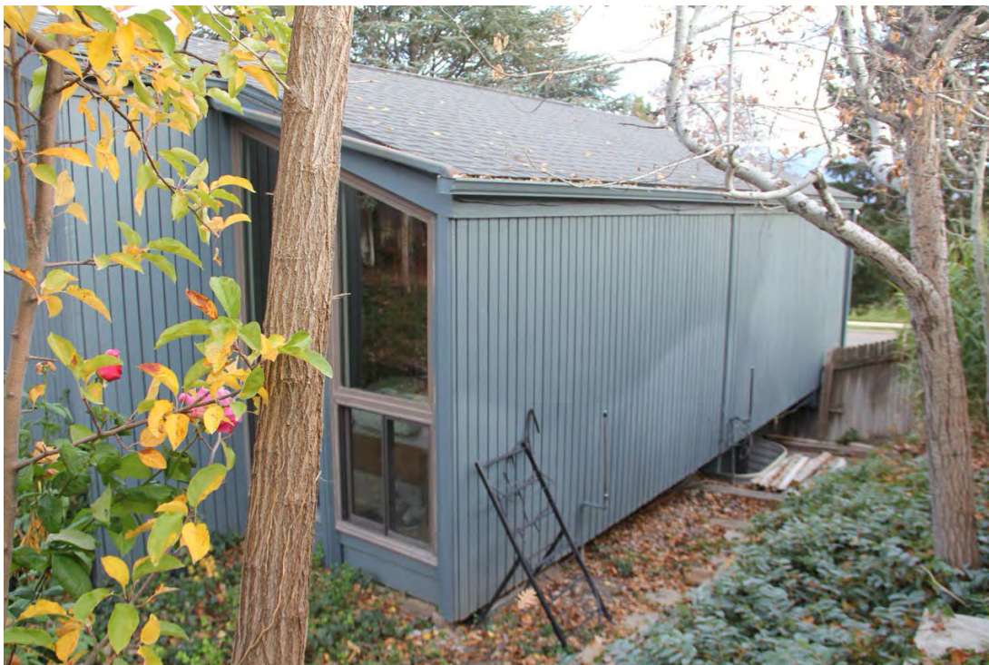
Photograph 11. Exterior, corner of north and west façade. Camera facing southeast.
