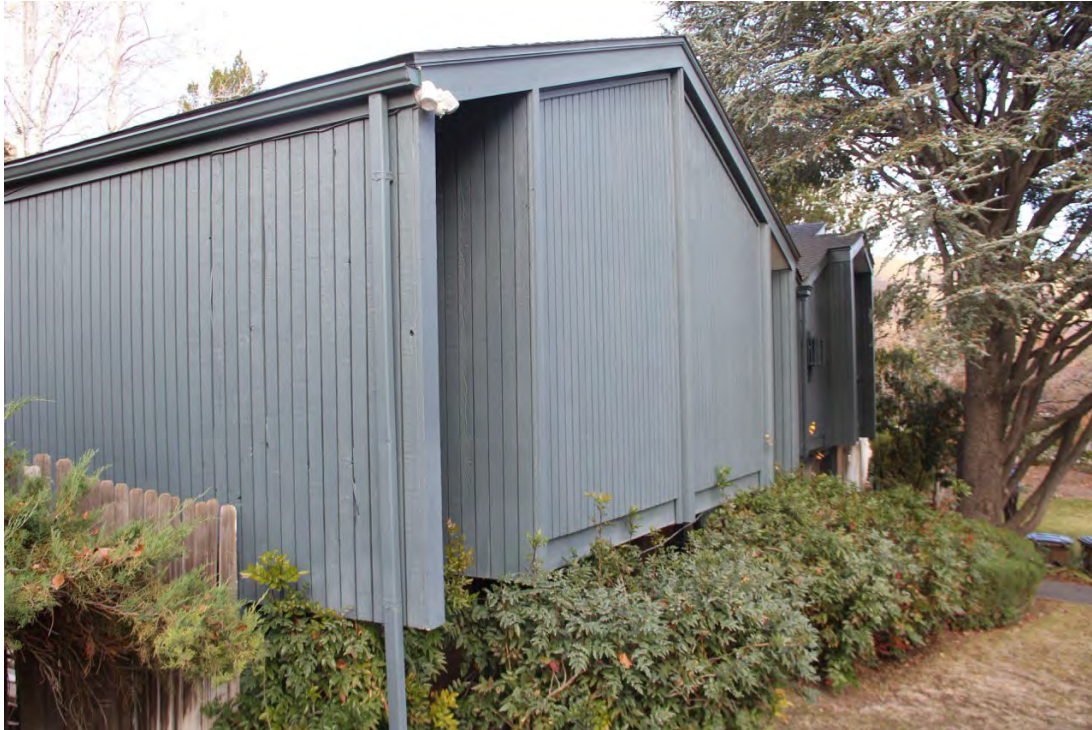
Photograph 3. Exterior, south (main) façade. Camera facing northeast.
