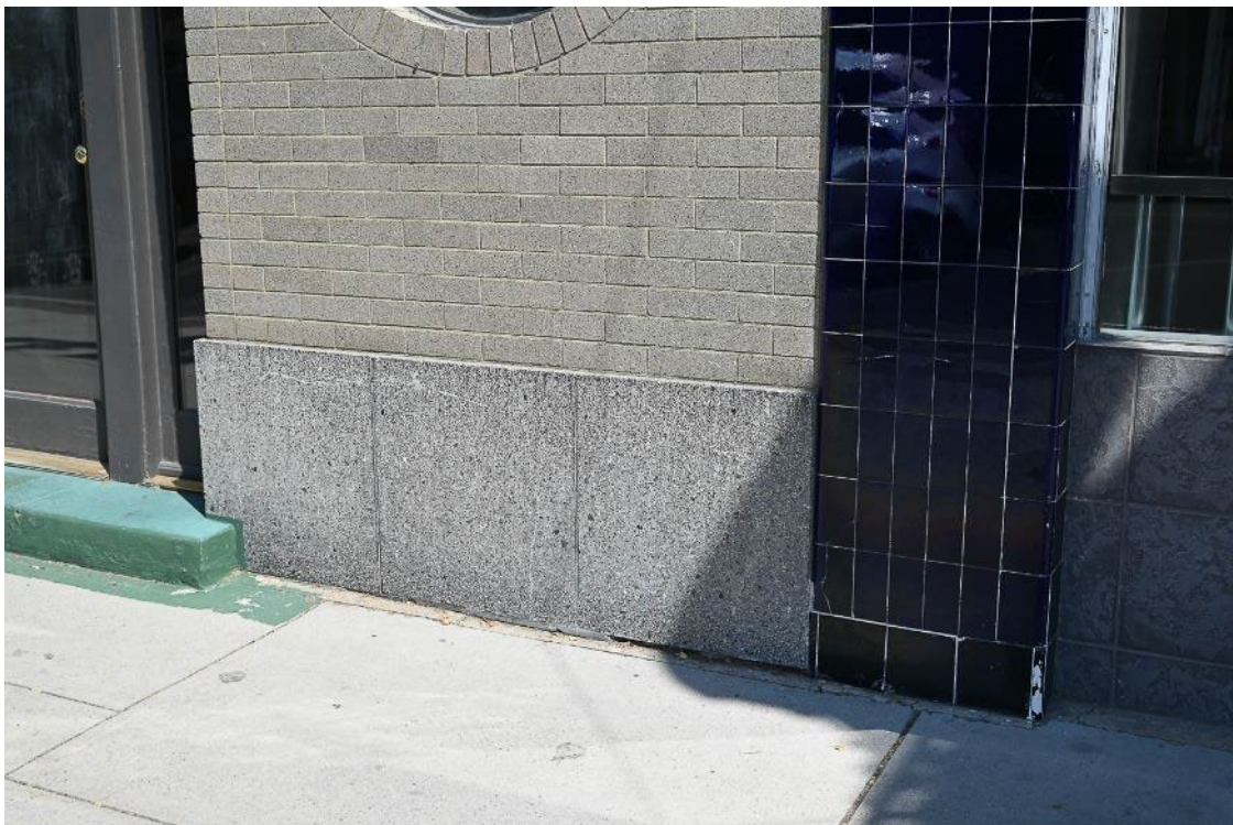
Photograph 6: South elevation (façade), window details. Camera facing north.
