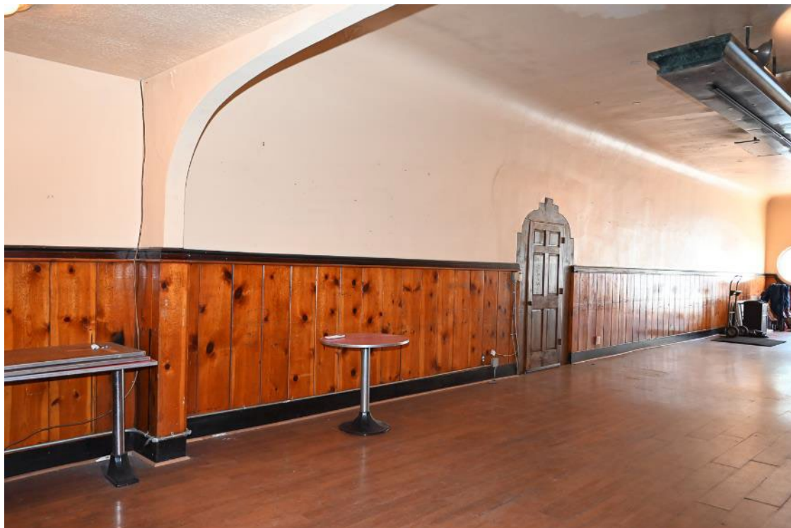
Photograph 14: Interior, main space, east wall and arch details. Camera facing southeast.
