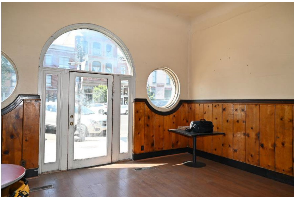
Photograph 10: Interior, southwest corner of main space. Camera facing southwest.
