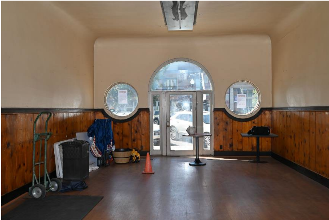
Photograph 9: Interior, main floor space, entry details. Camera facing south.
