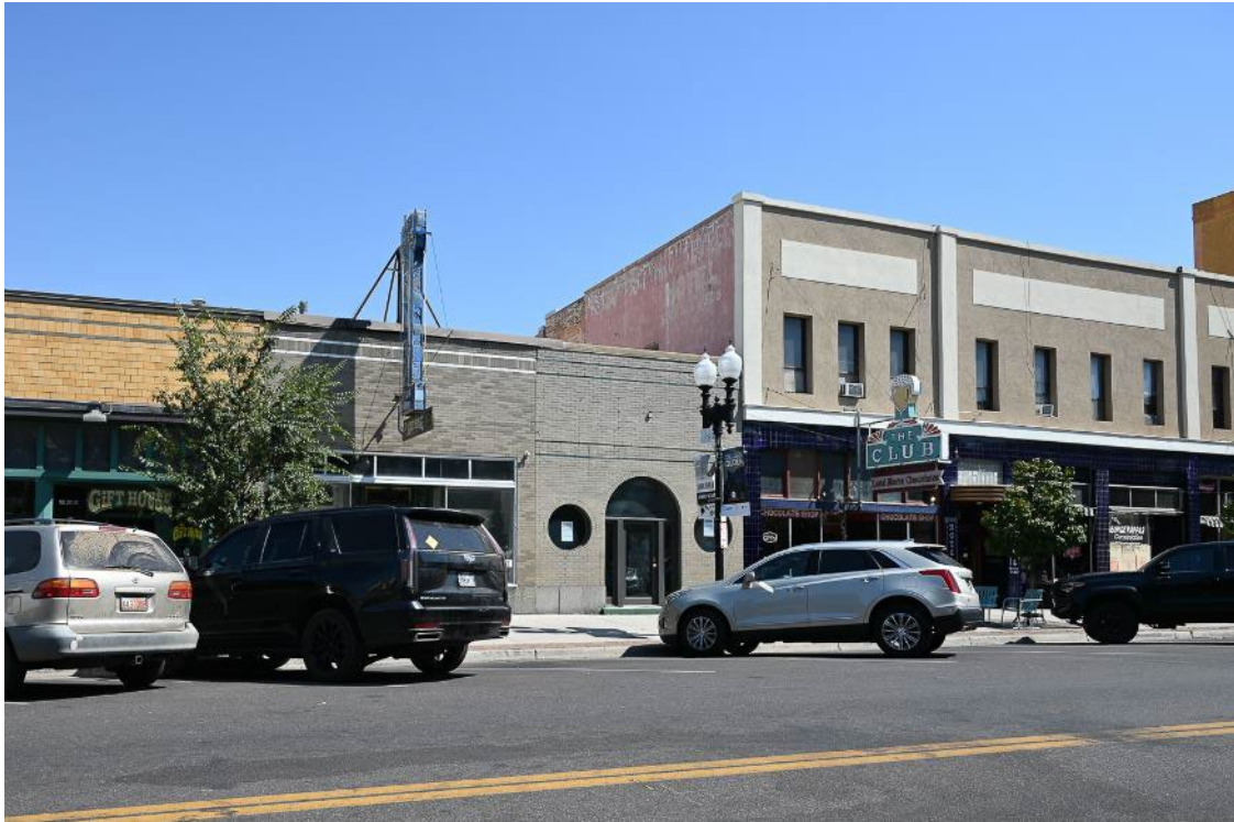
Photograph 1: Pearl Billiard Parlor/The Club in center of streetscape view of 25 th Street. Camera facing northeast.
