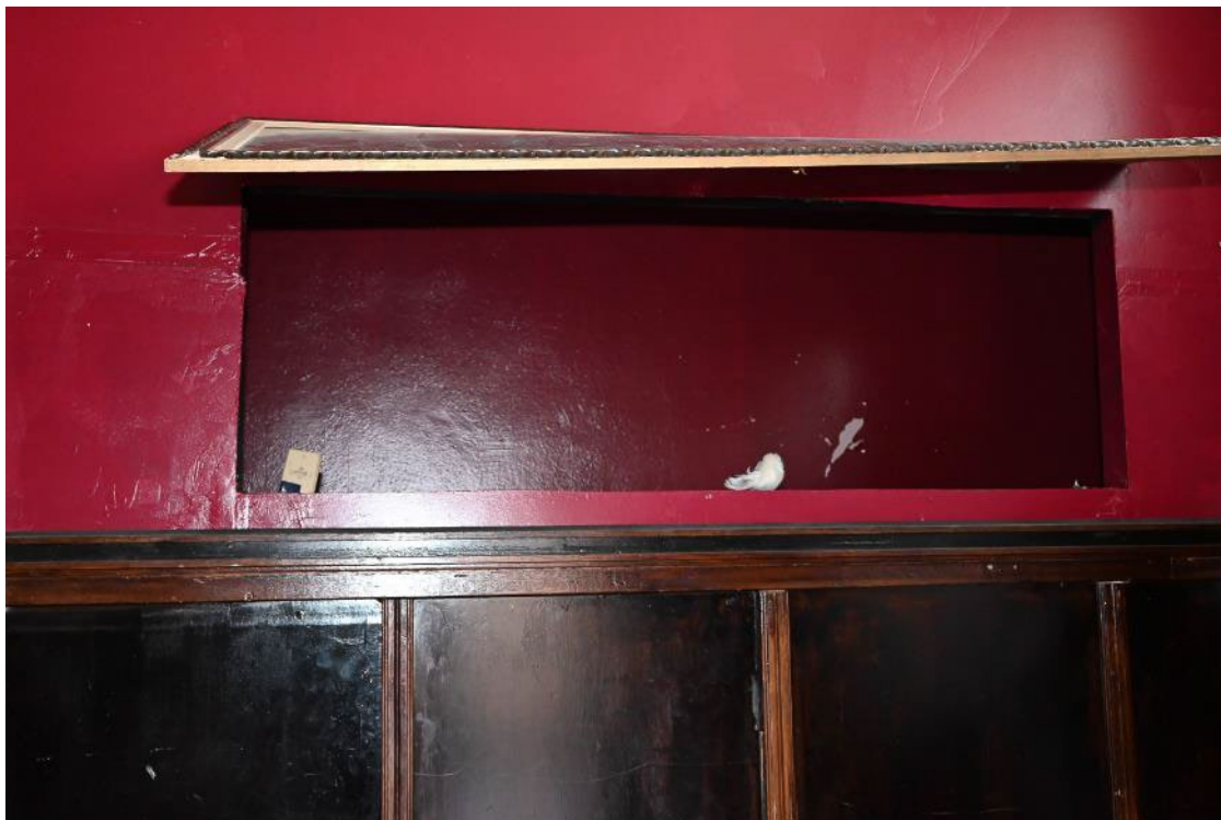
Photograph 20: Interior, back room (addition) and hidey hole details. Camera facing west.
