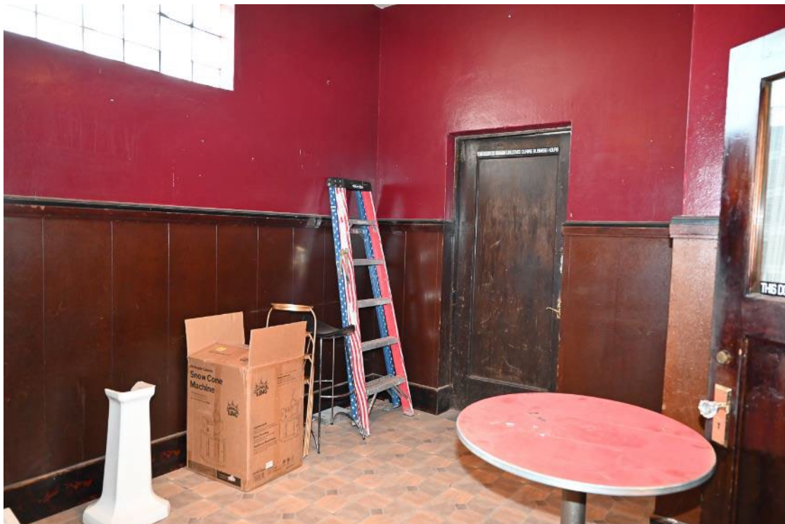
Photograph 18: Interior, back room (addition) and rear entry. Camera facing northeast.
