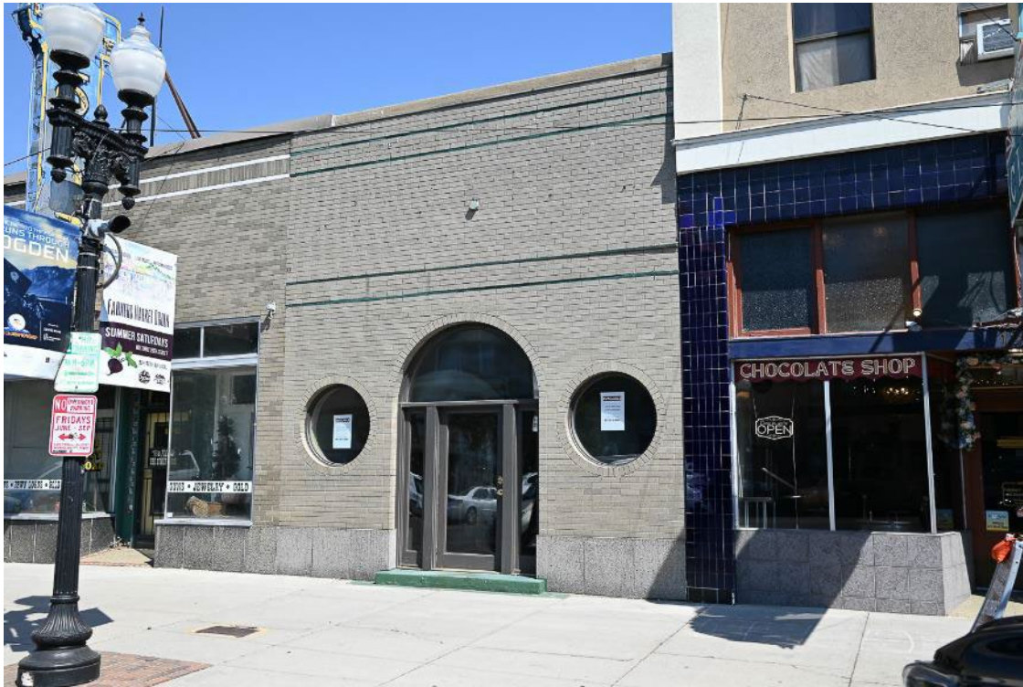
Photograph 3: South elevation (façade). Camera facing north.
