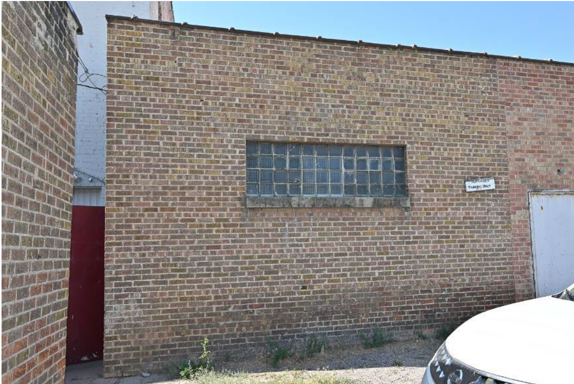
Photograph 7: North elevation (rear) addition. Camera facing south.
