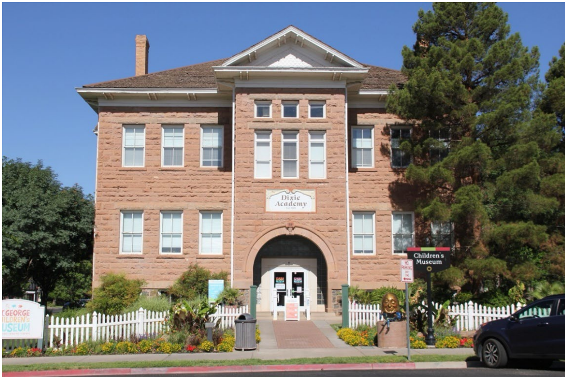
Photograph 21. Dixie Academy at 86 S. Main St. Contributing. Camera facing north
