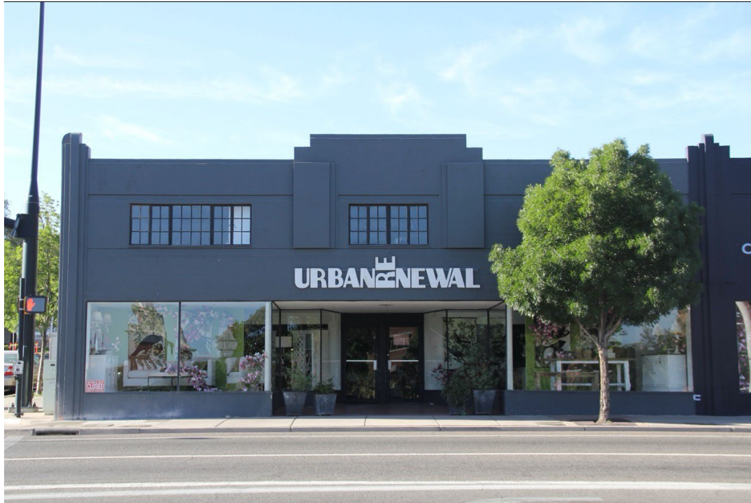
Photograph 32. J.C. Penney at 5 E. St. George Blvd. Contributing. Building has been repurposed but retains most of the original features. Camera facing north.
