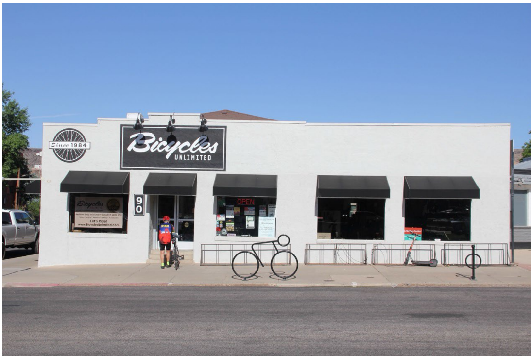
Photograph 56. Commercial building at 90 S 100 E. Noncontributing. Camera facing west.
