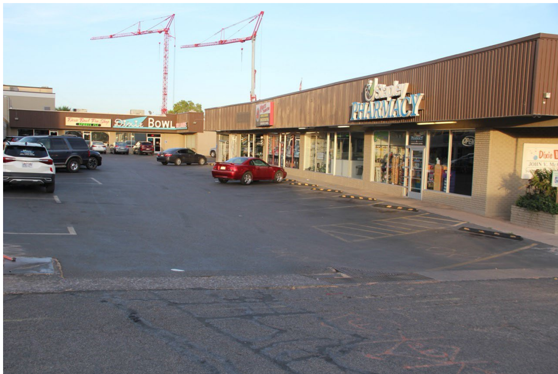
Photograph 33. Dixie Bowl and Billiards at 106 S. City Center Dr. Noncontributing. Camera facing east.
