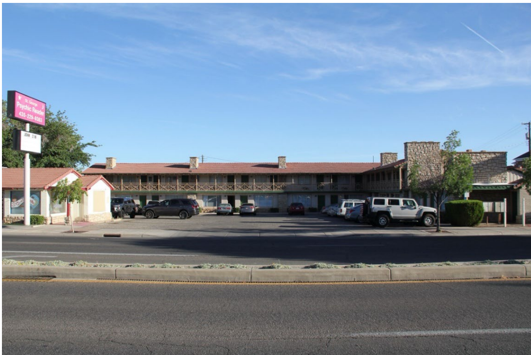
Photograph 35. Ranch Motel/El Pace'O Lodge/El Peso Motel at 111 W. St. George Blvd. Contributing. Camera facing south.
