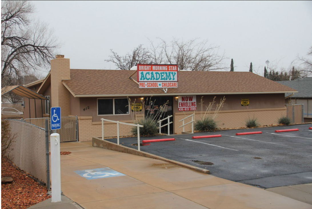
Photograph 59. Commercial building at 412 N 600 W. Noncontributing. Camera facing east.
