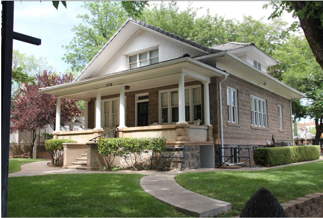
Photograph 63. The Joe Burgess House at 172 N 100 W is a fine example of the Bungalow/Craftsman style. Contributing. Camera facing east.
