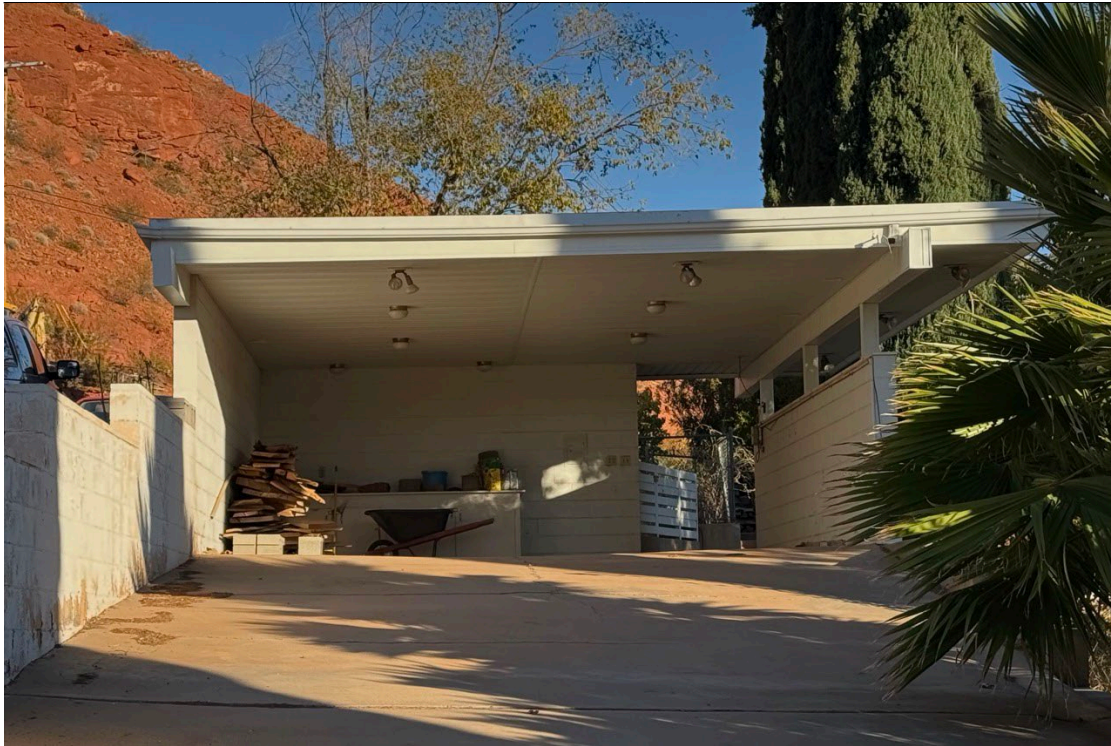
Photograph 48. Carport at 88 W 475 N Circle. Contributing. Camera facing east.
