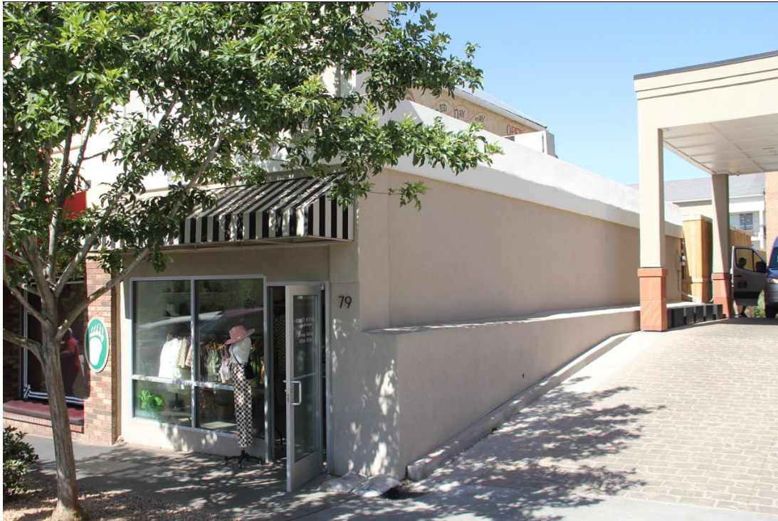
Photograph 55. Earliest extant commercial building in St. George (ca. 1880), located at 79 N. Main St. Noncontributing. Camera facing southwest.
