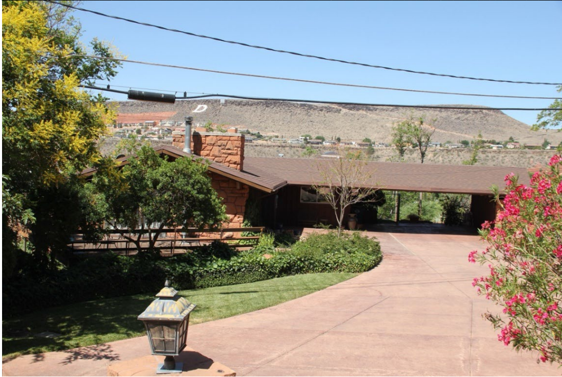
Photograph 38. Watson House at 335 N 100 W designed by L. Robert Gardner. Contributing. Camera facing west.
