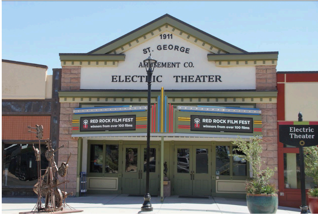
Photograph 22. Electric Theater at 70 E. Tabernacle St. Contributing. Camera facing south.
