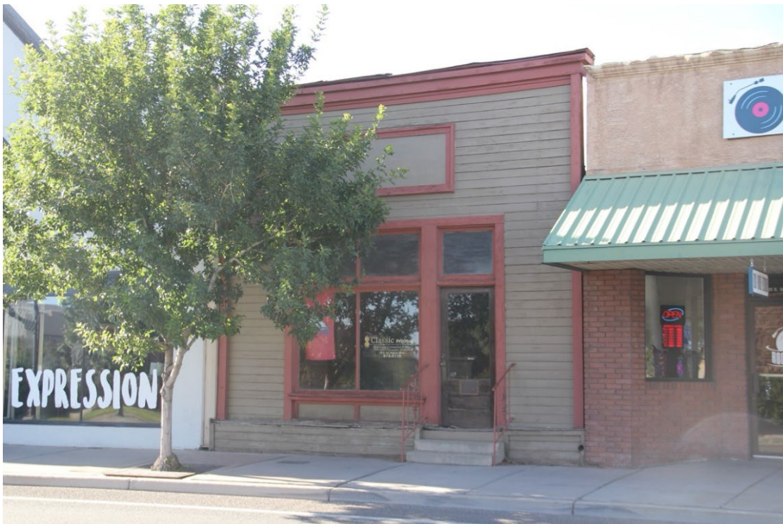
Photograph 16. Silver Reef Saloon/Washington County News at 23 E. St. George Blvd. Contributing. Camera facing north.
