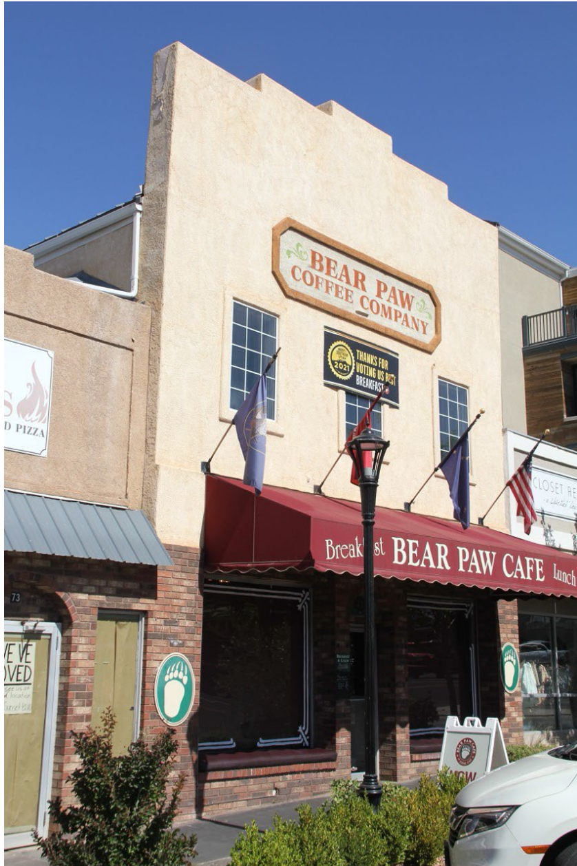
Photograph 19. St. George LDS Tithing Office at 75 N. Main St. Noncontributing. Camera facing west.
