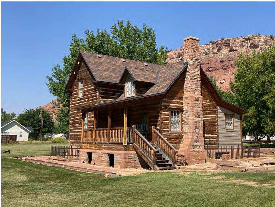
Photo 39. Residence at 10 South 140 West., Vernacular, ca. 1900; moved here in 1985, Noncontributing. Camera facing northwest.
