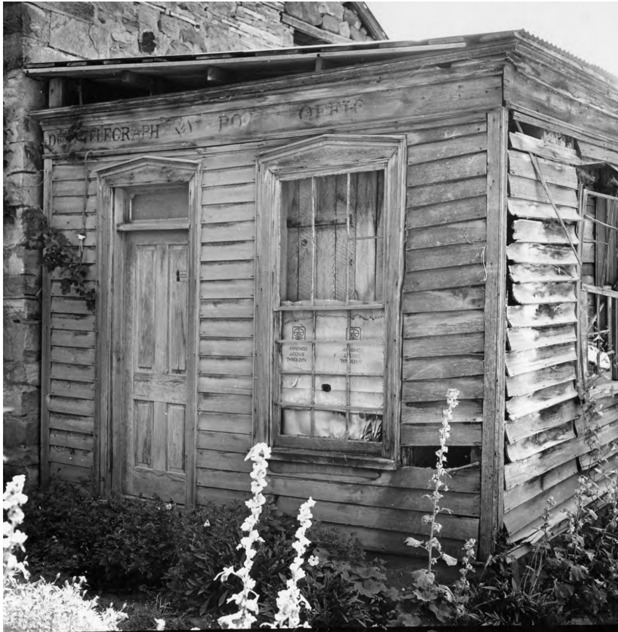
Figure 9. Close up view of the Deseret Telegraph addition to the Huber House at 91 W. Main St. Photo taken ca. 1940. Credit: Parker Hamilton. Source: Utah State Historical Society, Department of Cultural and Community Engagement.
