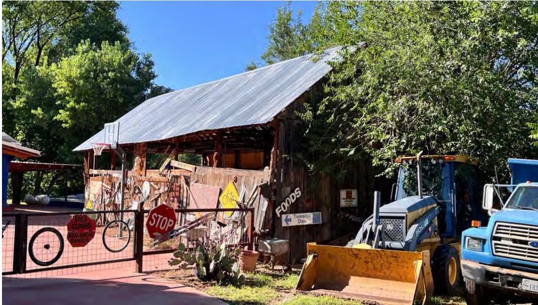
Photo 47. Example of a hay shed, repurposed for general storage. Located at 51 South 130 East. Contributing. Camera facing southeast.
