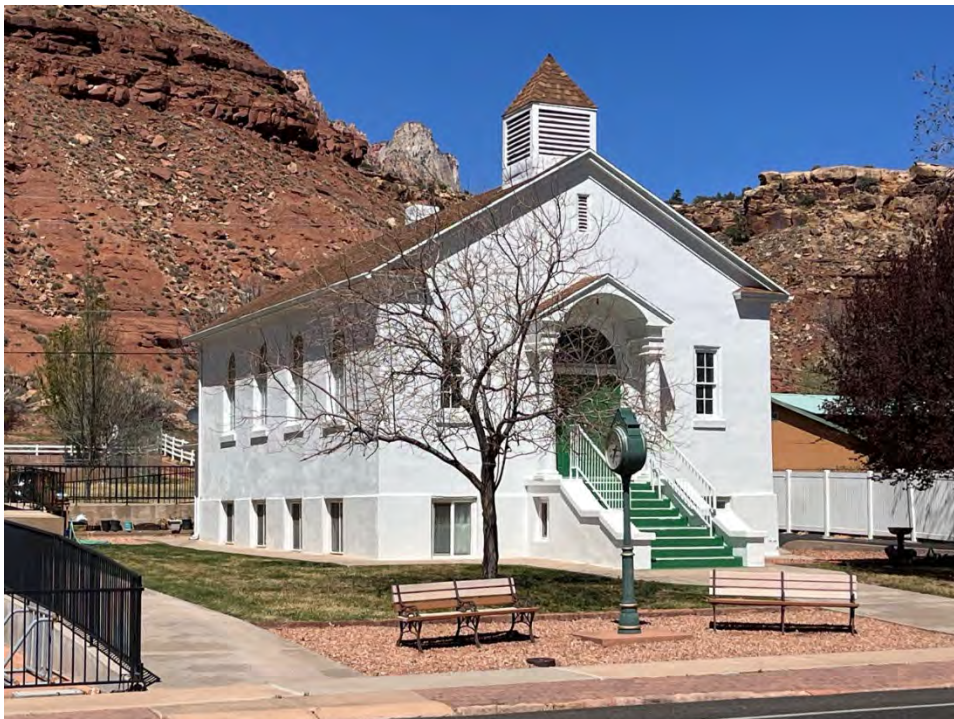
Photo 50. The Rockville LDS Chapel at 53 E. Main St. is the one example of the vernacular Neoclassical style in the district. Contributing. Camera facing northeast.
