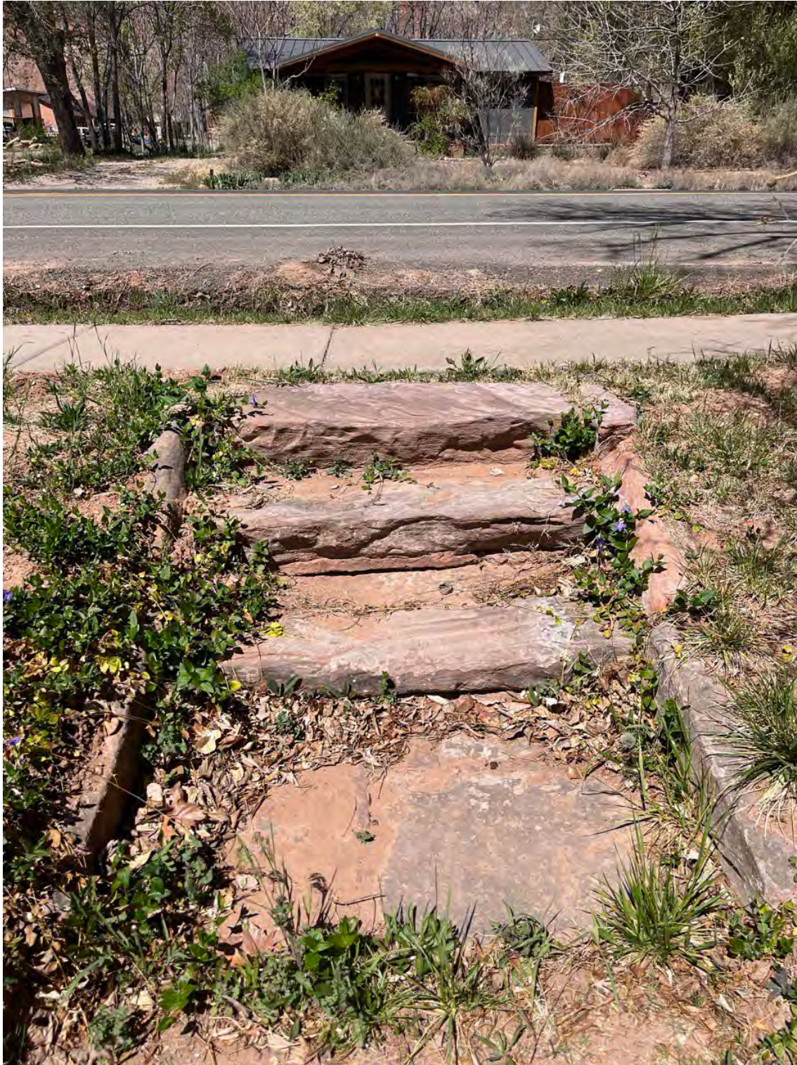
Photo 15. Landscape. Sandstone steps (Contributing as part of the irrigation system construction) constructed by the WPA on the south side of Main Street. Camera facing north.
