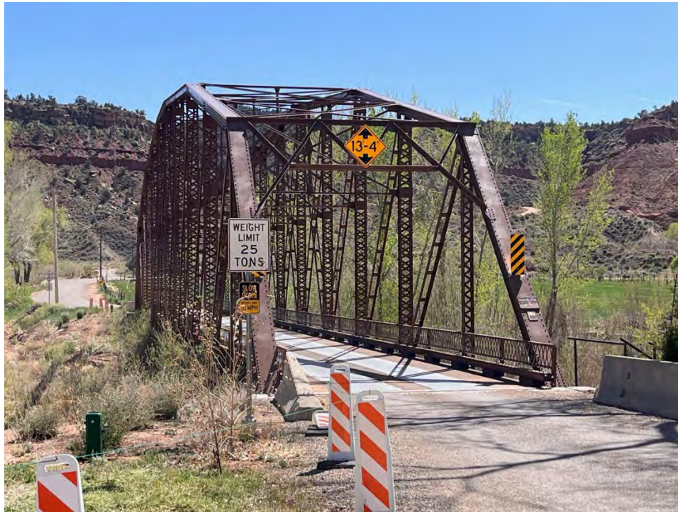
Photo 27. The Rockville Bridge was completed in 1924, listed in the NRHP in 1995, and rehabilitation completed in 2019. Camera facing north.
