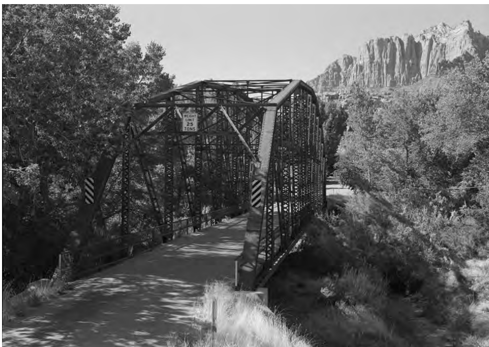
Figure 5. The Rockville Bridge was completed in 1924. Funded by the National Park Service, it served as the first connection between Zion National Park and the Grand Canyon, allowing tourists to reach both parks easily by automobile. Credit: Brian C. Grogan. Source: Library of Congress, HAER-UT-74.
