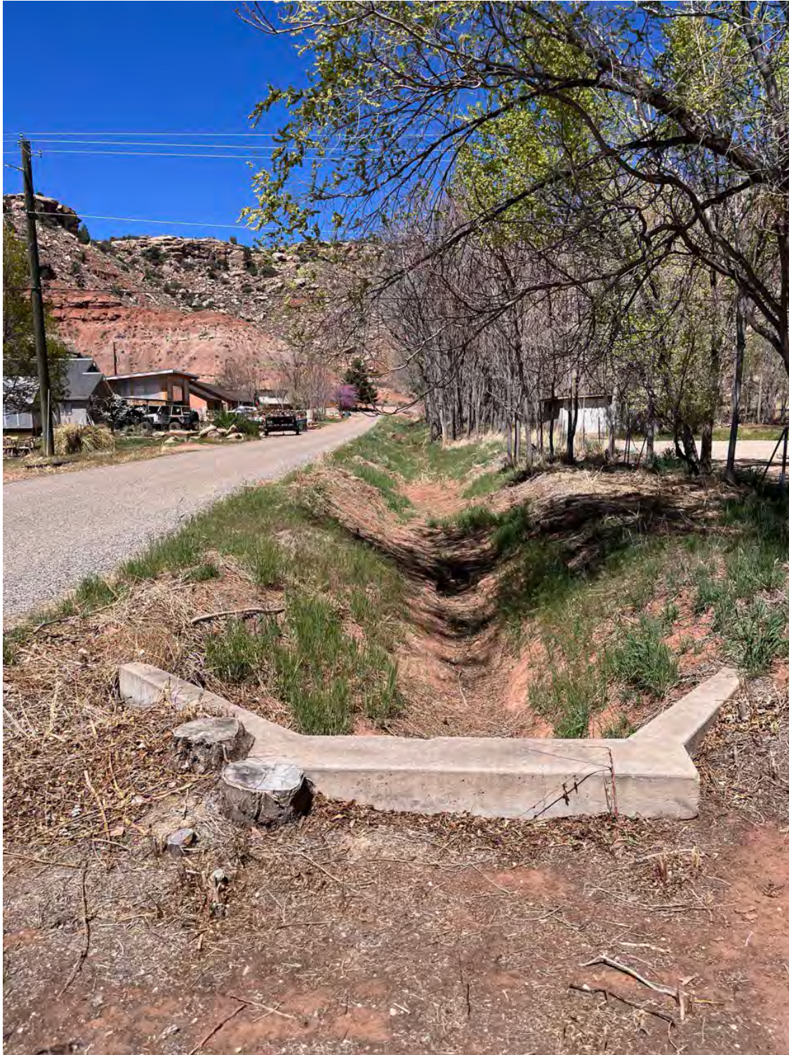
Photo 9. Landscape. The west irrigation ditch (Contributing) as it flows into the concrete culvert that carries the water under Main Street toward the Virgin River. Camera facing north.
