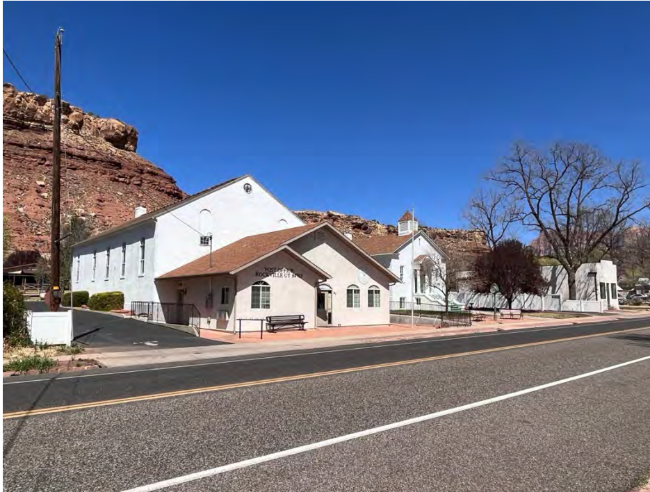
Photo 29. LDS Amusement Hall (Rockville Town Hall), left, 1934, Period Revival: Other, Noncontributing. LDS Chapel (Rockville Community Center), right, 1932, Neoclassical, Contributing. Camera facing northeast.
