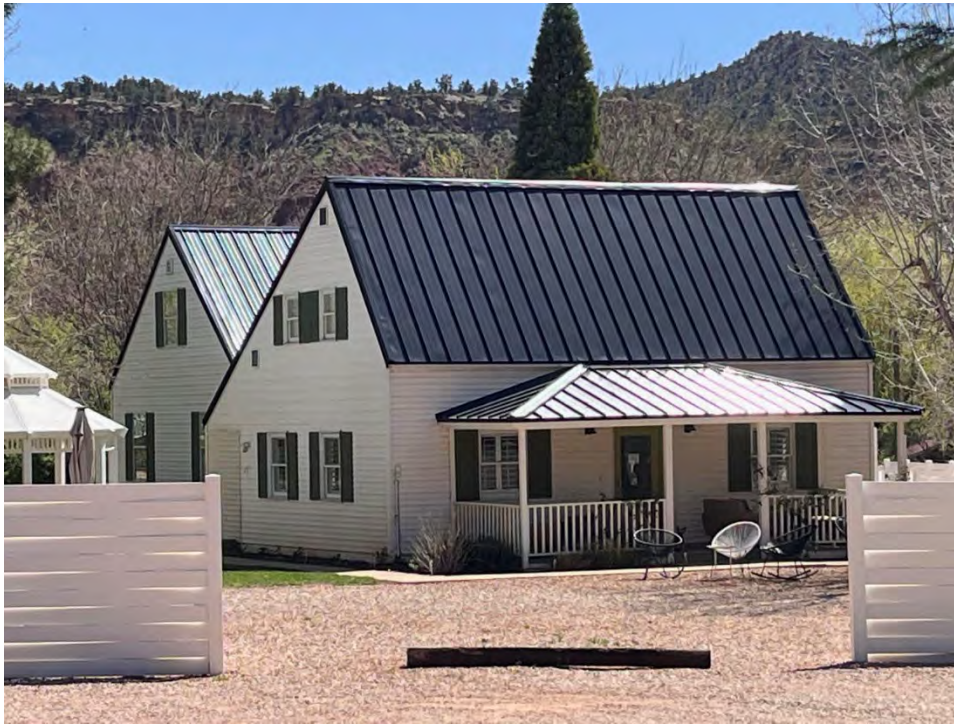
Photo 38. Heller House Inn at 225 E. Main St., 1984, Neo-Colonial, Noncontributing. Camera facing south.
