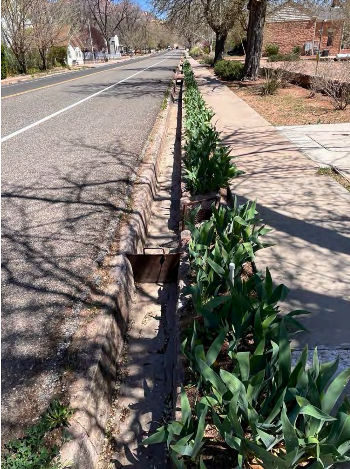
Photo 14. Landscape. The small u-shaped sandstone irrigation ditch on the south side of Main Street showing culvert-type bridges and an original control gate. Contributing. Camera facing east.
