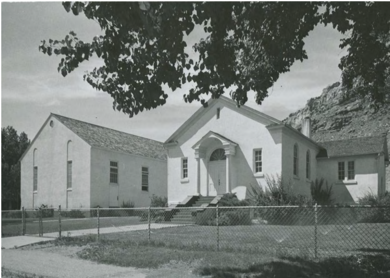
Figure 11. Rockville Ward LDS Chapel (right) and Amusement Hall (left) in 1958. The Amusement Hall has been adaptively used as the town hall while the chapel serves as a community meeting space that is owned and operated by the Town of Rockville. Source: Church History Library, The Church of Jesus Christ of Latter-day Saints.
