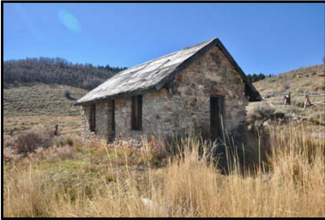
Photo 9: East and North Walls, View to the Southwest
