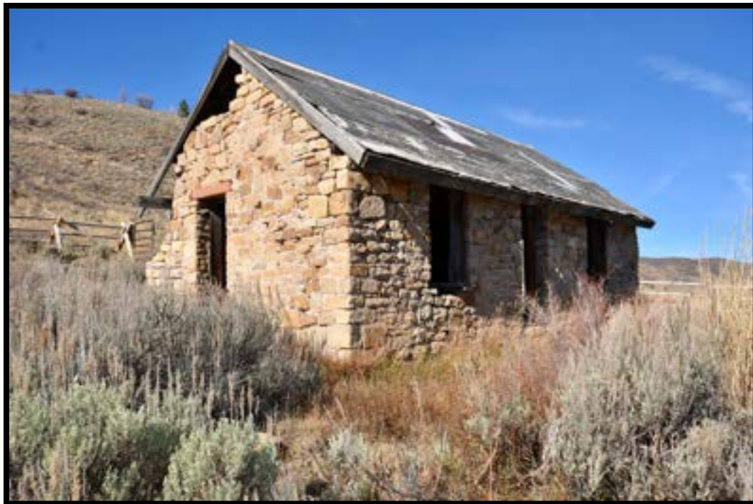
Photo 6: South and East Walls, View to the Northwest
