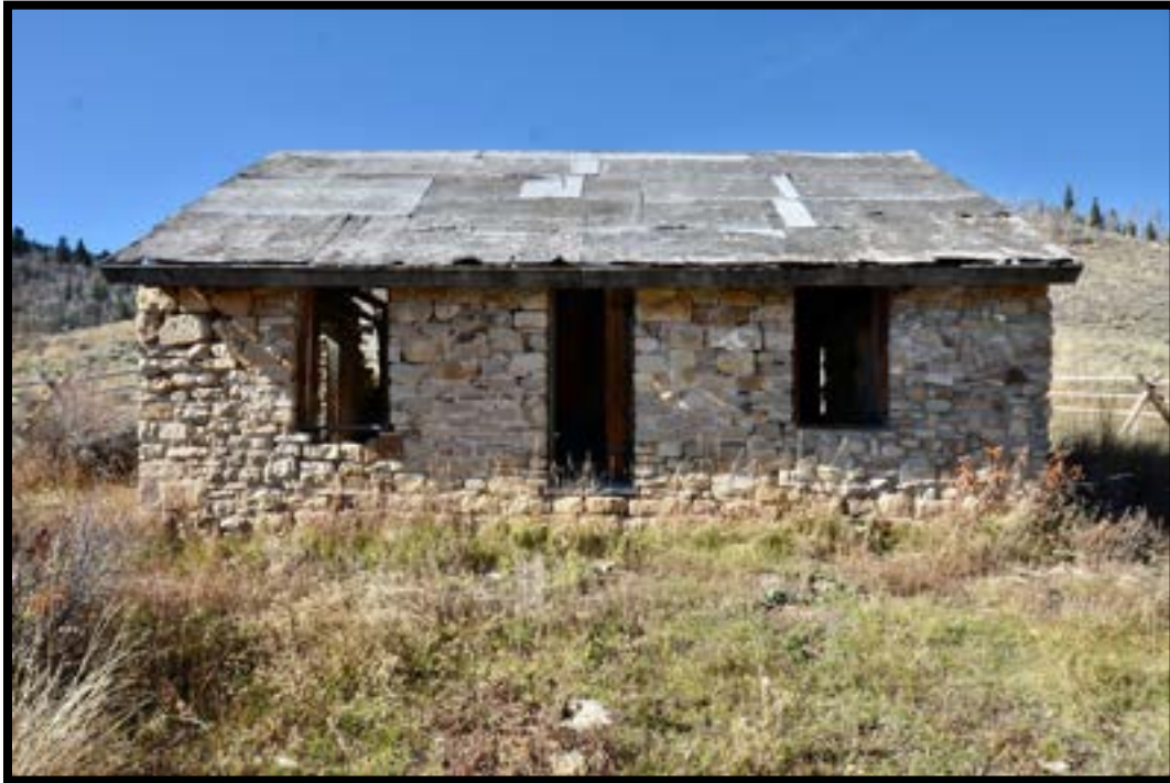
Photo 5: East Façade, View to the West
