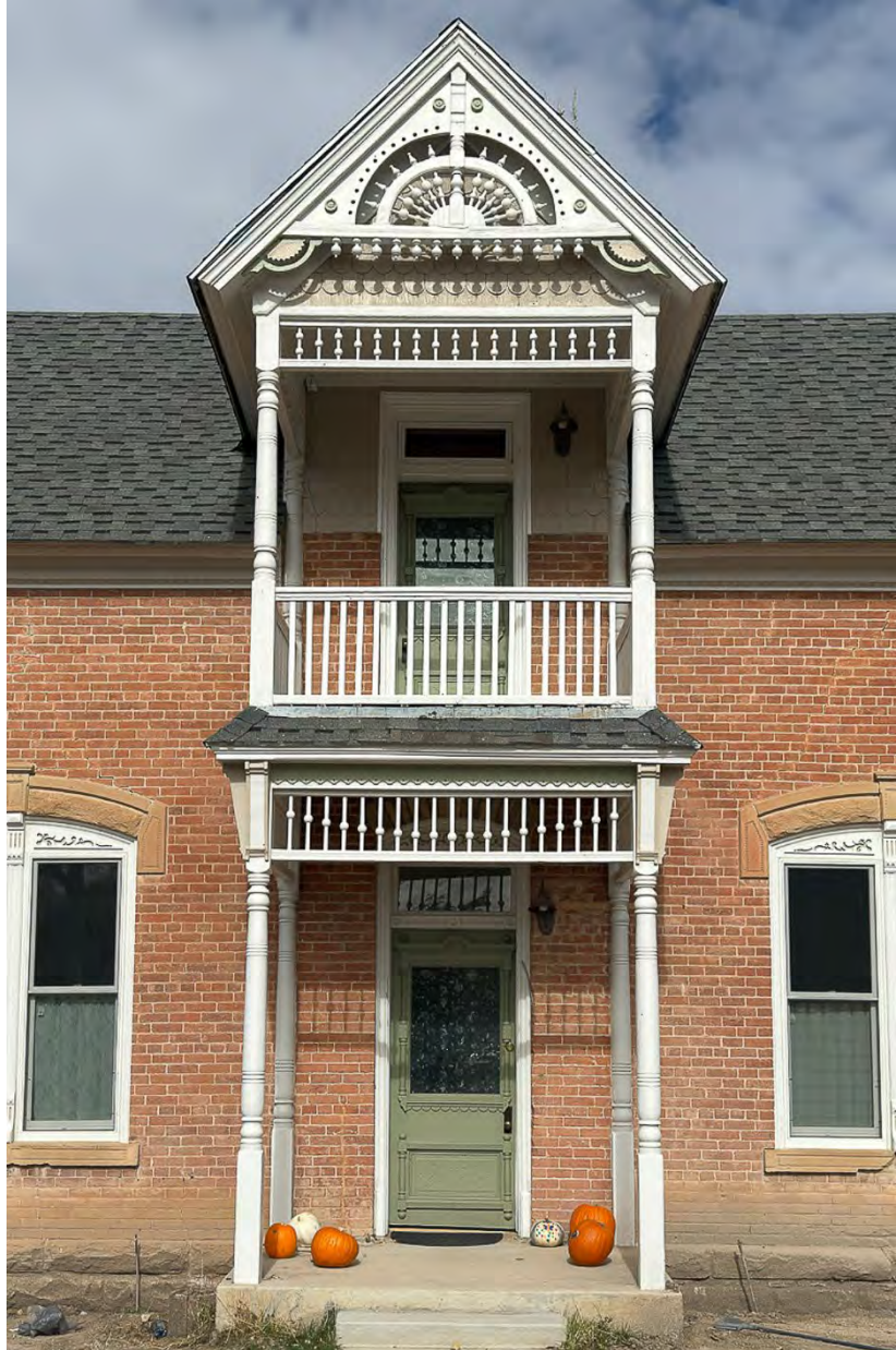
Photograph 3 South elevation, details of porch and balcony. Camera facing north.
