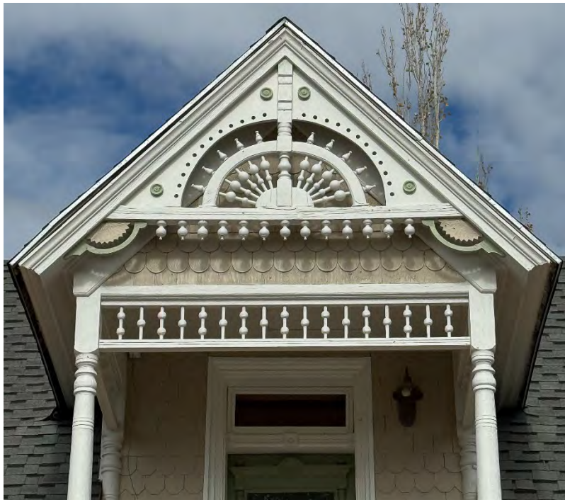
Photograph 5 South elevation, balcony ornamentation details. Camera facing north.
