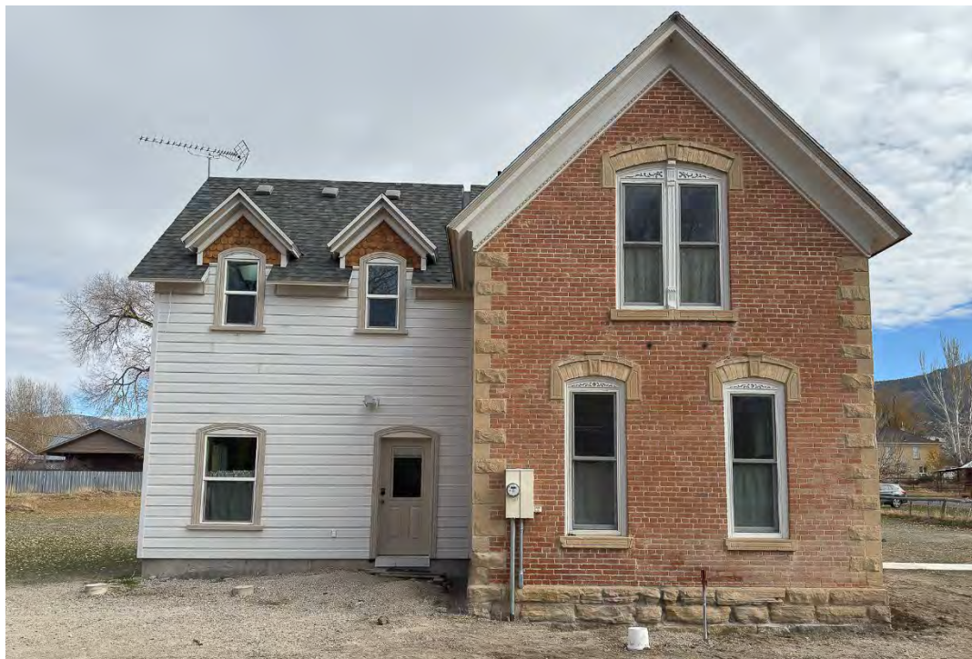
Photograph 7 West elevation of house and addition. Camera facing east.
