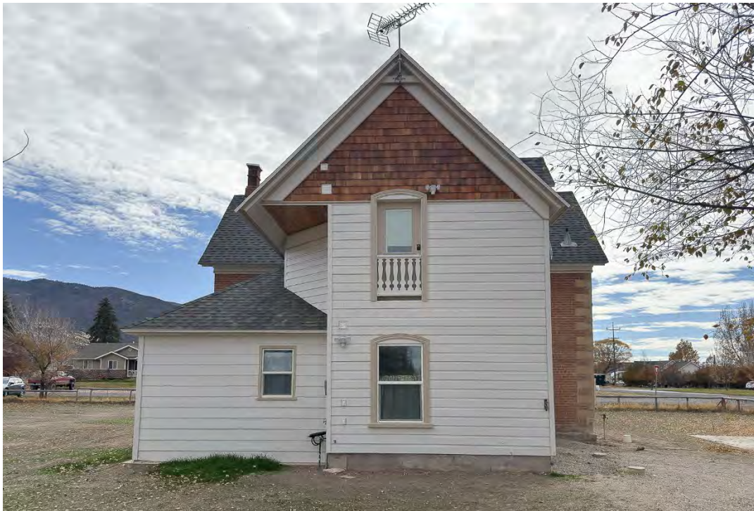
Photograph 8 North elevation of addition. Camera facing south.
