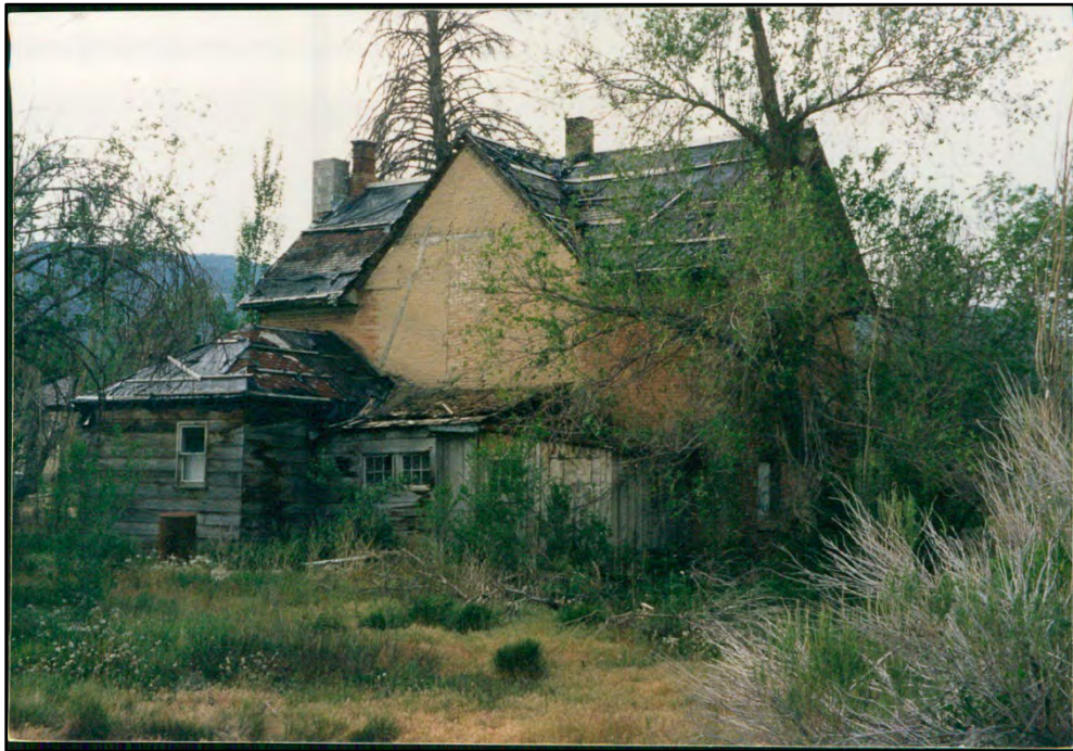
Figure 6 North elevation (circa 1994). Camera facing southeast.
