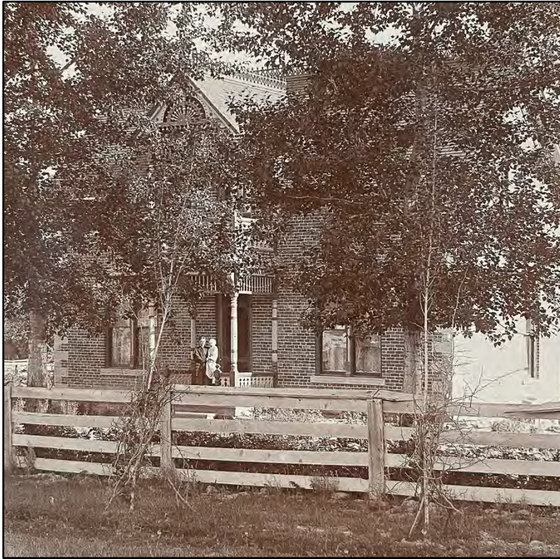
Figure 1 South and west elevations (circa 1900). Camera facing northwest.
