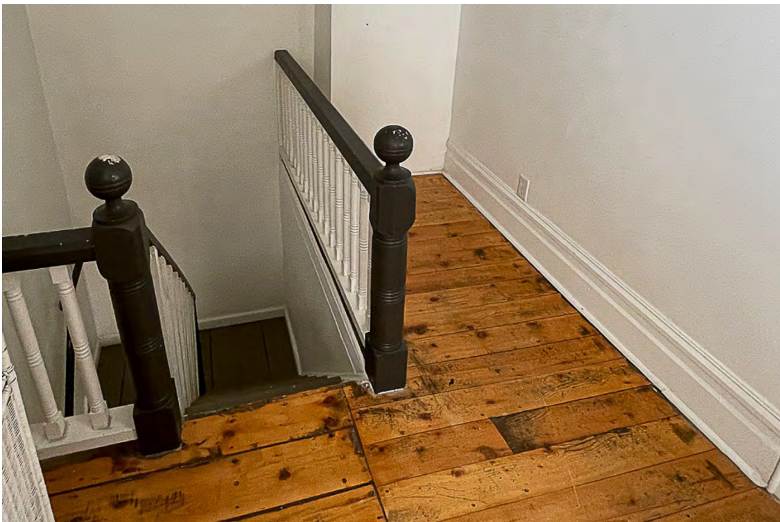
Photograph 14 Interior, second floor, landing and stairs. Camera facing northeast.
