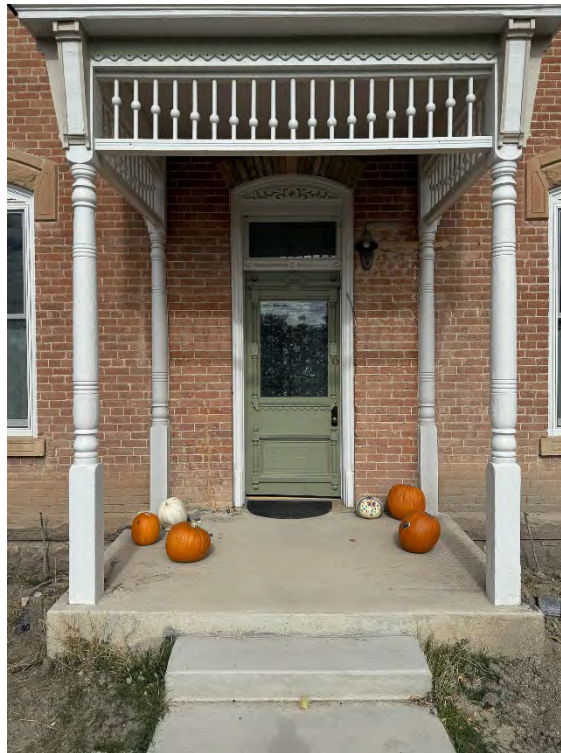
Photograph 4 South elevation, porch and door details. Camera facing north.
