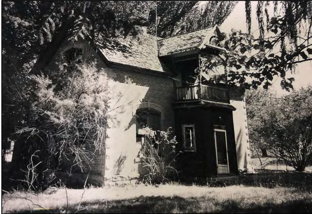
Figure 4 South and west elevations (circa 1980). Camera facing northeast.
