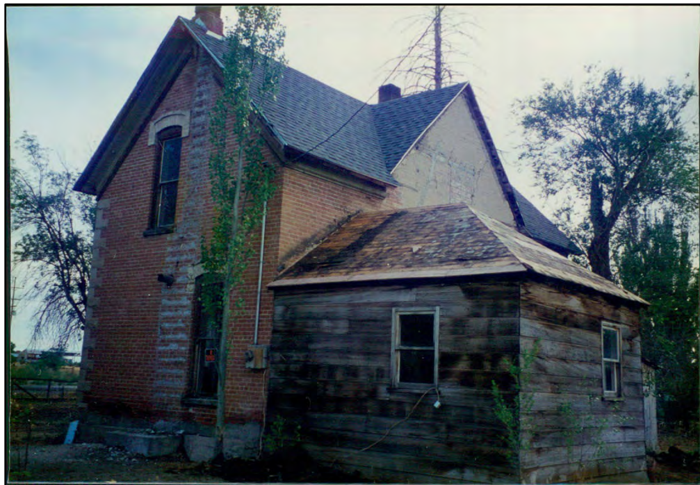
Figure 7 East and north elevations (circa 1995). Camera facing southwest.
