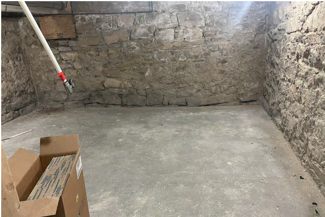
Photograph 13 Interior, basement. Camera facing east.
