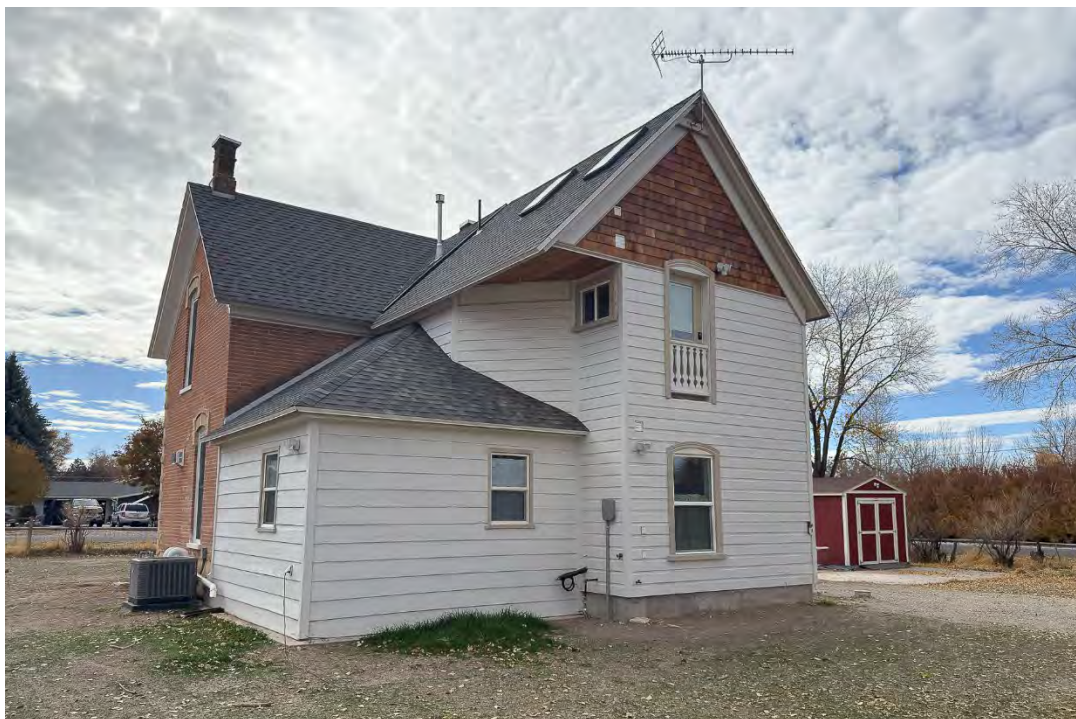
Photograph 9 North and east elevations of addition. Camera facing southwest.
