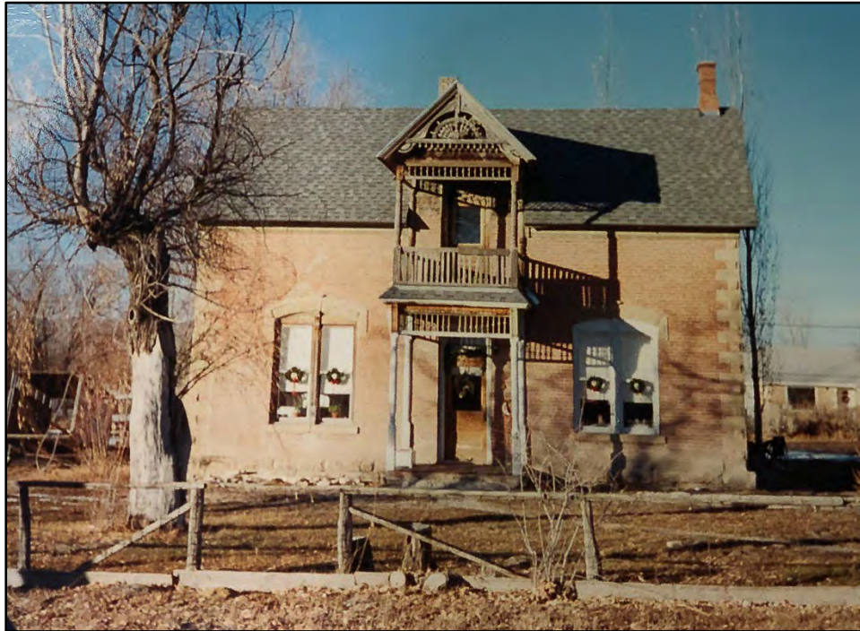
Figure 8 South elevation (circa 1995). Camera facing north.
