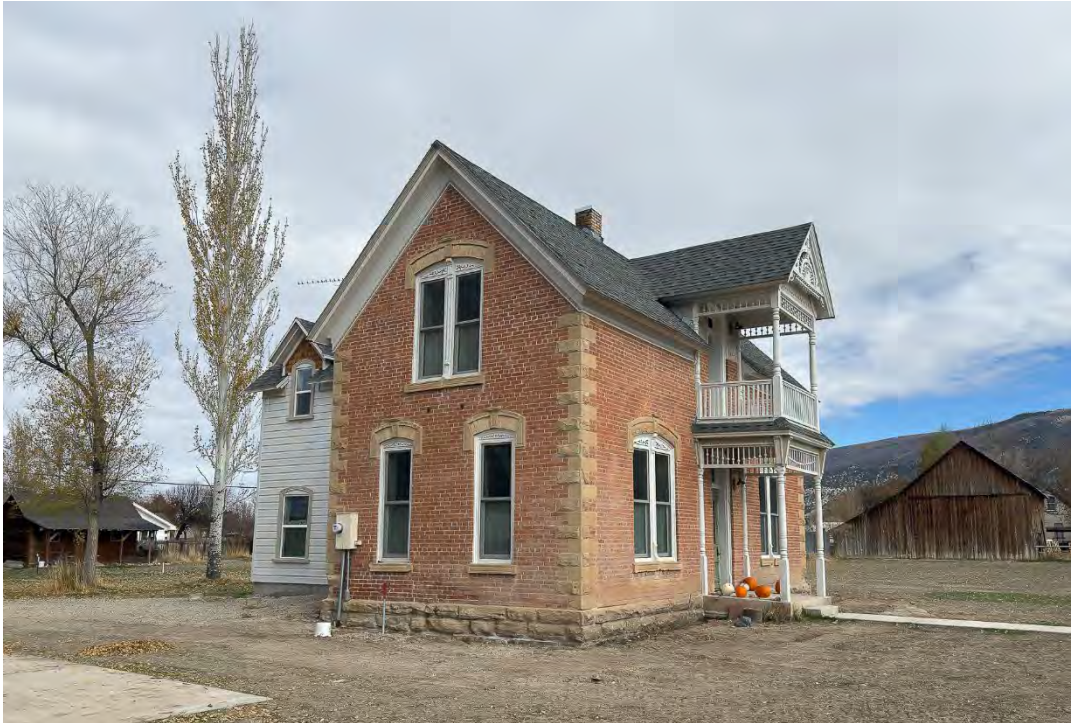
Photograph 6 South and west elevations of house. Camera facing northeast.
