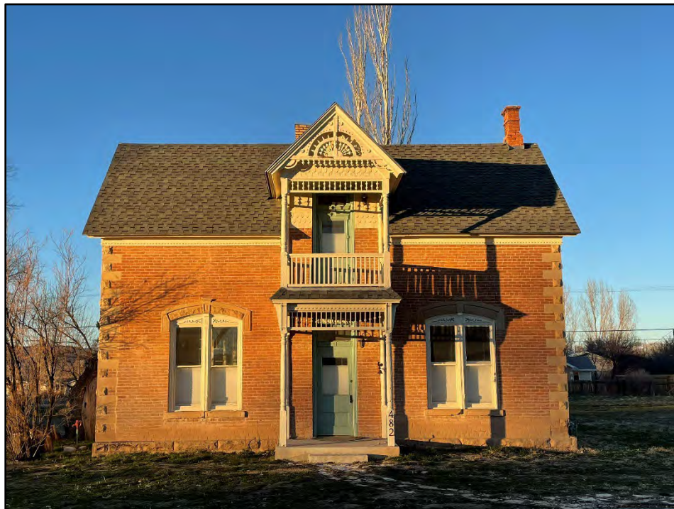
Figure 9 South elevation (2021). Camera facing north.
