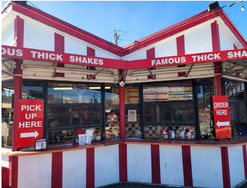
Photograph 8. Exterior, east (main) façade detail of walk-up windows. Camera facing west.
