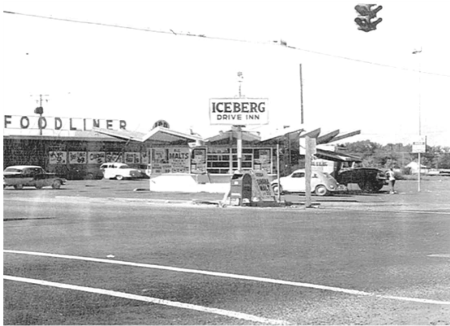
Figure 1. Photograph of the Iceberg Drive-Inn circa 1962. Note the IGA Foodliner to the left. Camera is facing southwest. Credit: Iceberg Drive-Inn.
