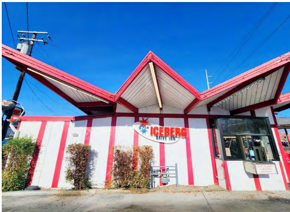
Photograph 9. Exterior, south façade detail of drive-thru. Camera facing north.
