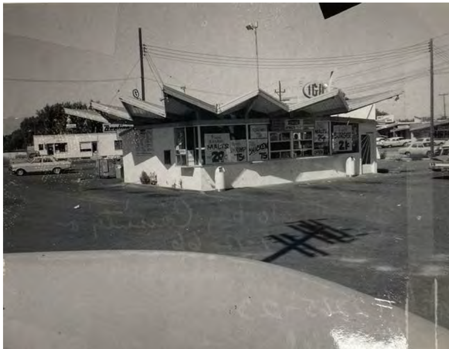
Figure 2. Photograph of the Iceberg Drive-Inn, 1966. Note the east façade door to the dining room addition visible at the far right. Camera is facing northwest. Credit: Salt Lake County Archives.
