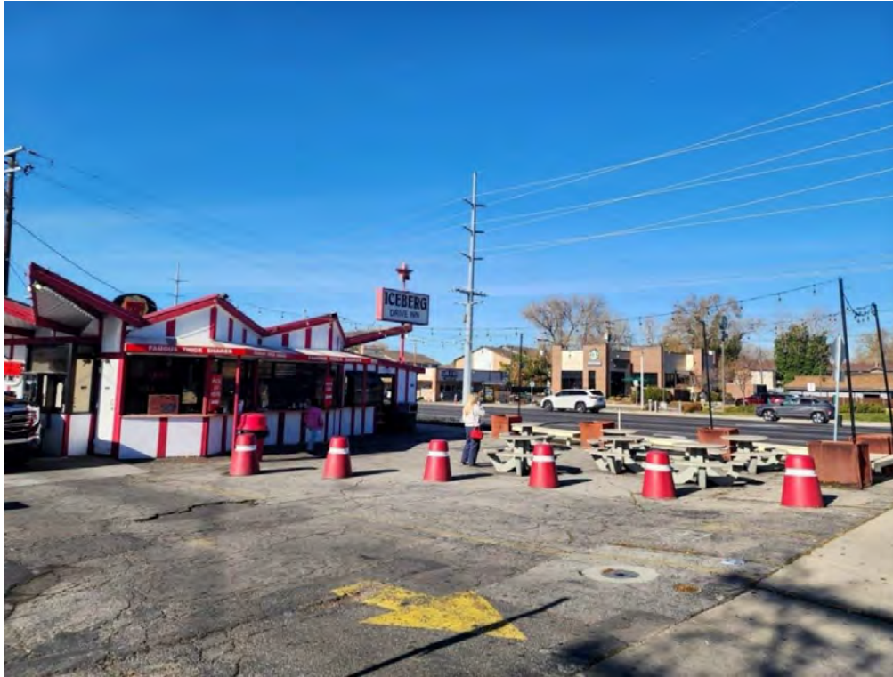
Photograph 5. Exterior, east (main) façade and surrounding area. Camera facing northwest.
