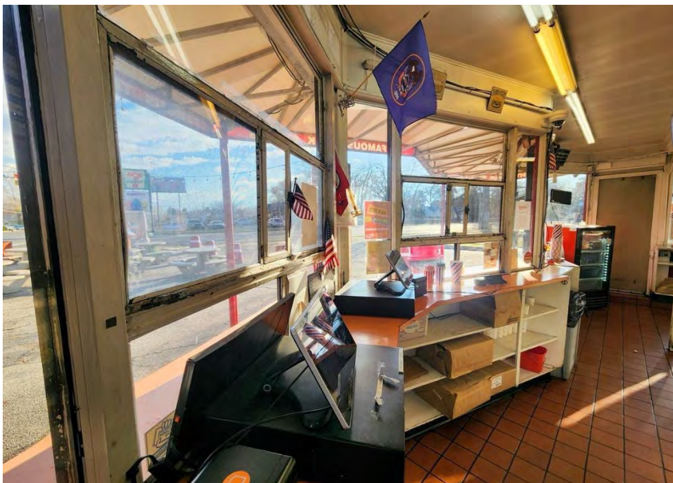
Photograph 15. Interior, detail of sliding order and pick-up windows. Camera facing southeast.
