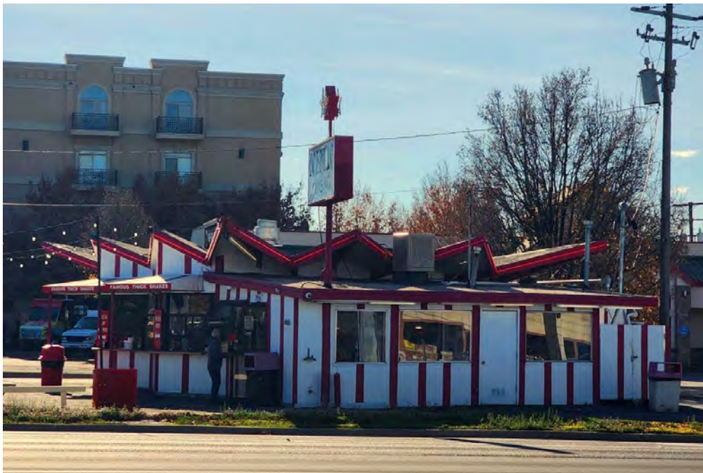
Photograph 2. Exterior, north façade. Camera facing southwest.
