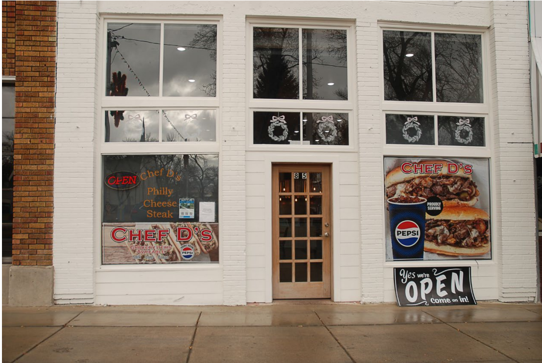
Photograph 3: South elevation of building, storefront entrance. Camera facing north.
