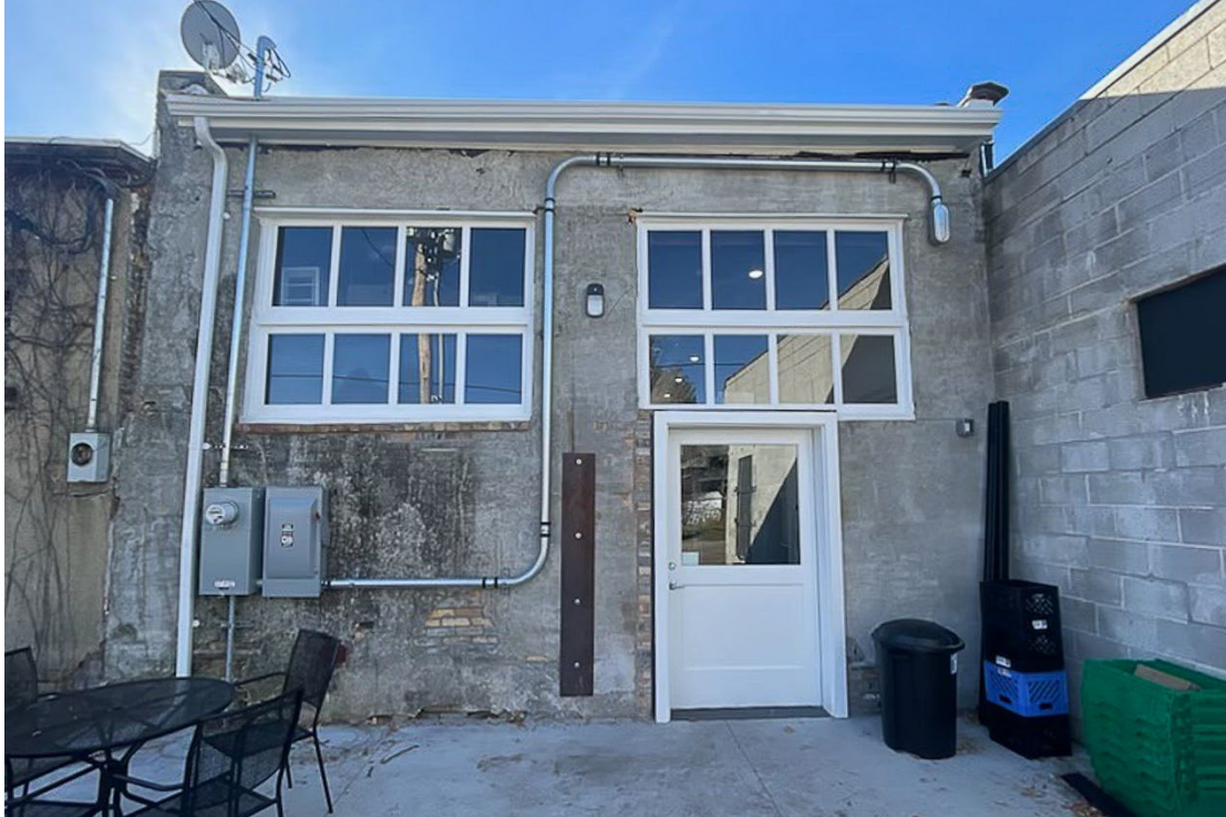
Photograph 5: North (rear) elevation. Camera facing south.
