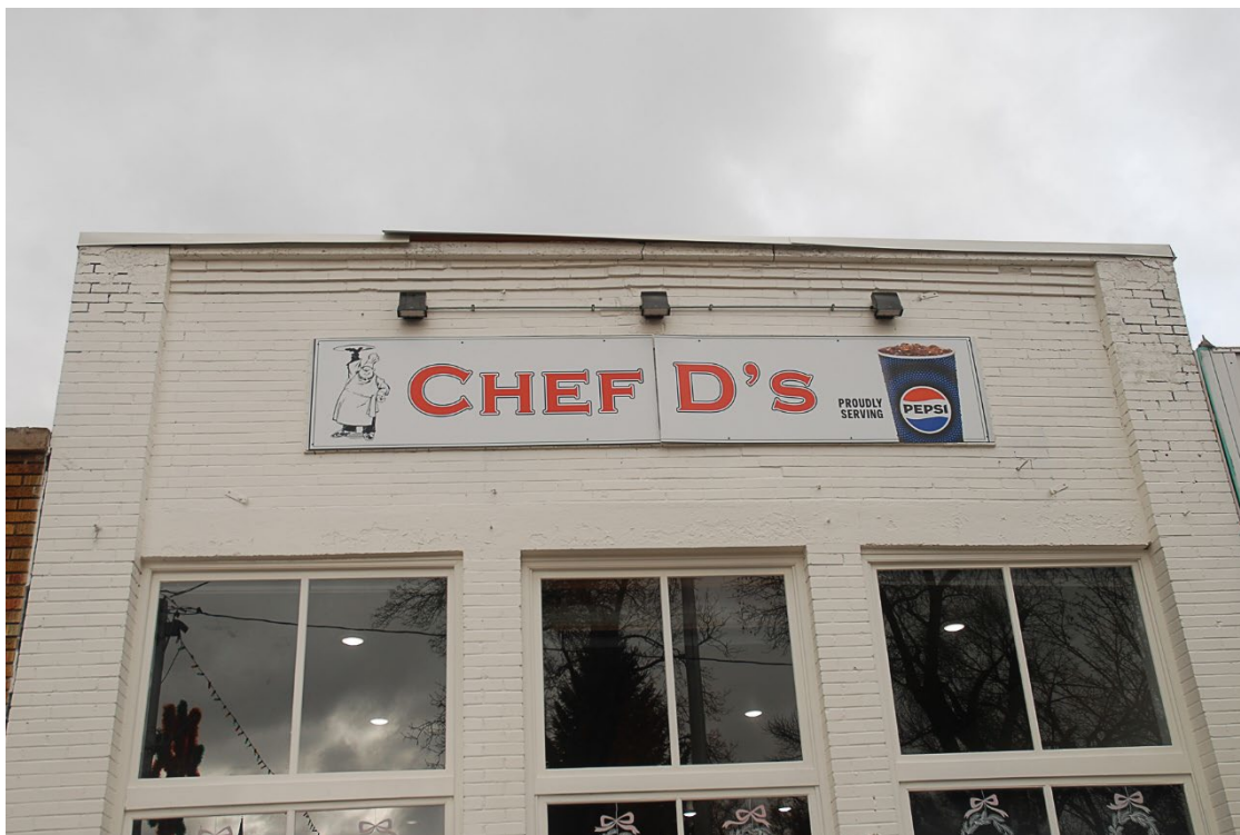
Photograph 4: South elevation, window and parapet details. Camera facing north.
