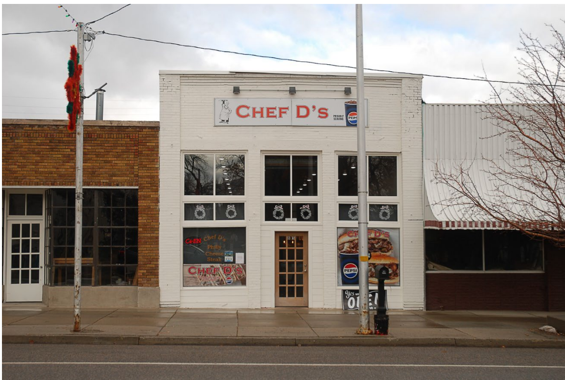
Photograph 2: South elevation of building. Camera facing north.
