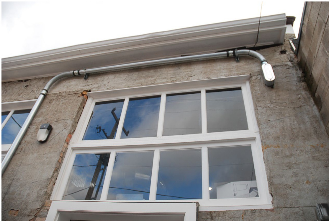
Photograph 6: North (rear) elevation, window detail. Camera facing south.
