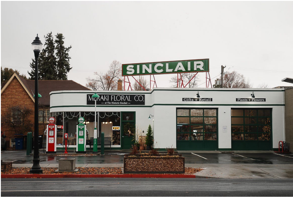
Photograph 2 North elevations of Dale's Sinclair Service Station. Camera facing south.
