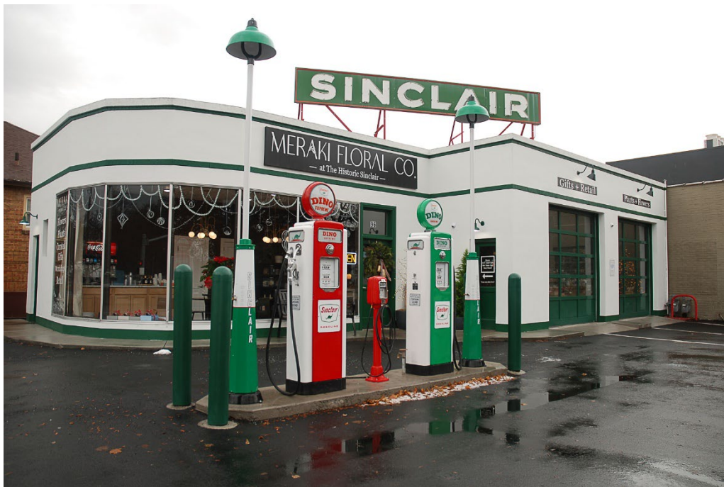
Photograph 3 North and east elevations of Dale's Sinclair Service Station. Camera facing southwest.
