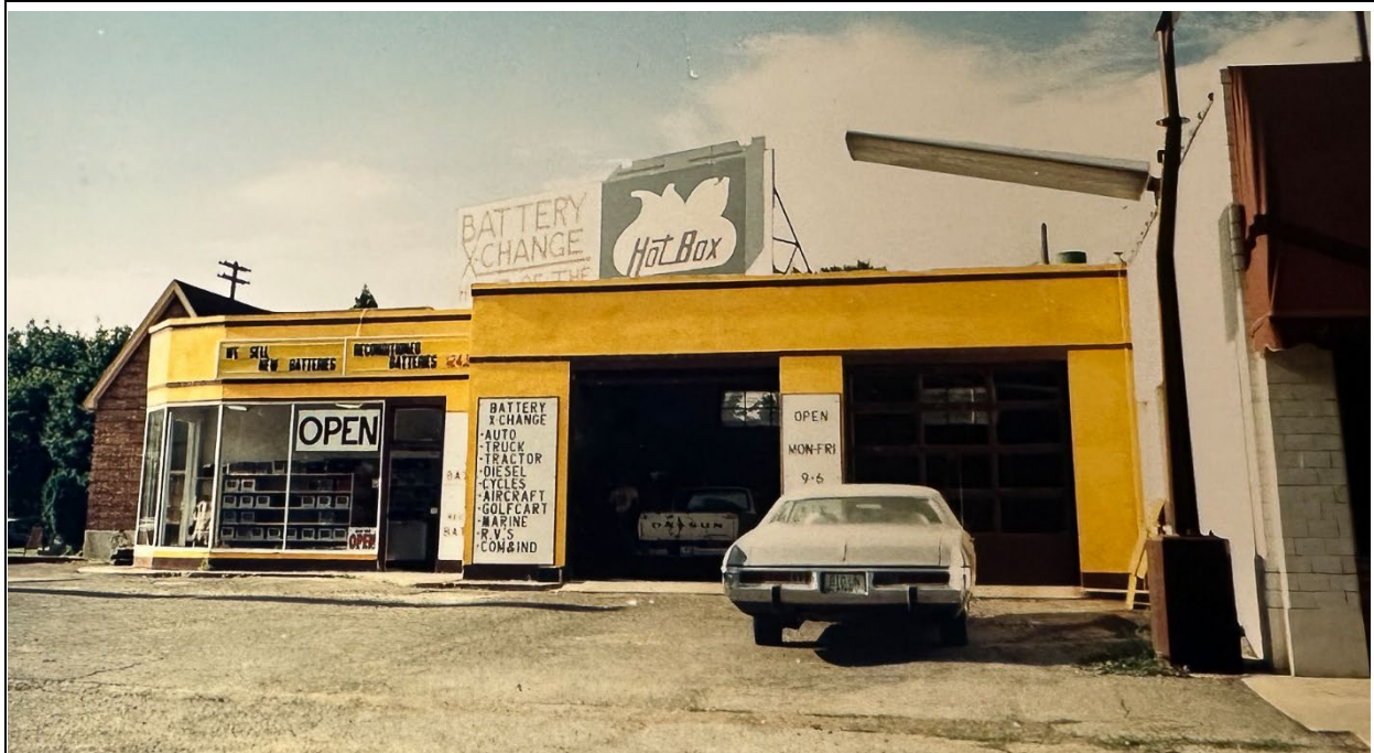
Figure 3 Dale's Sinclair Service Station, photographed circa 1984. Courtesy Cache County Tax Assessor's Office.
