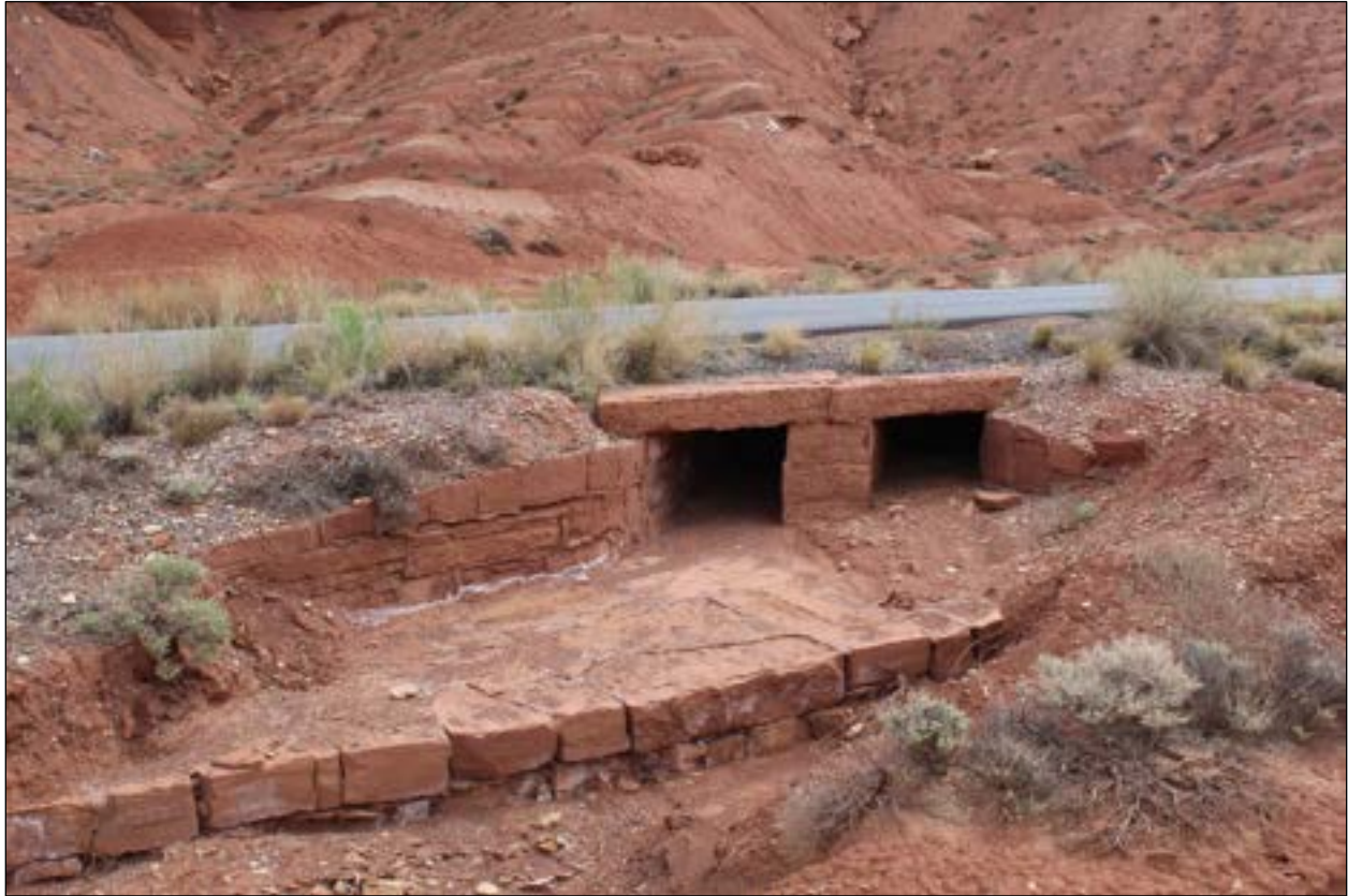
Photo 007. The CCC-constructed culvert at milepost 2.26 has a double box culvert with sandstone inlet and outlet basins. The culverts feature large, coursed, squared sandstone blocks. View to the east-southeast.
