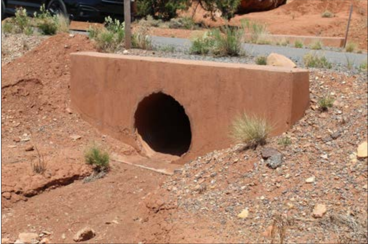
Photo 018. After the period of significance, culverts with poured concrete headwalls were constructed along Scenic Drive. View to the northeast of the culvert near milepost 6.90.
