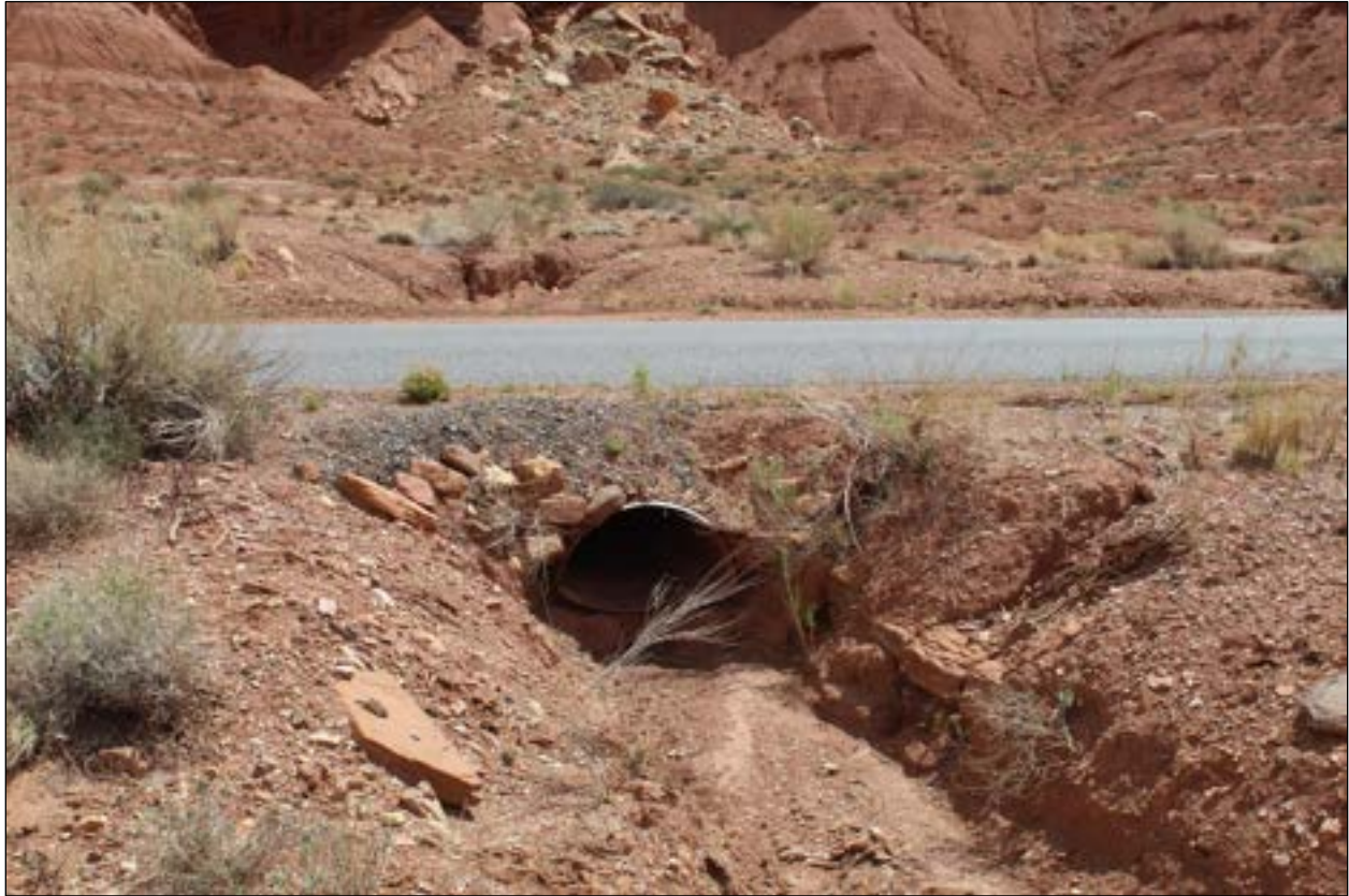
Photo 019. This culvert near milepost 1.90 was likely built by the CCC, indicated by the large sandstone blocks used for the headwall, but its condition has deteriorated to the point that it no longer retains historic integrity. View to the east.
