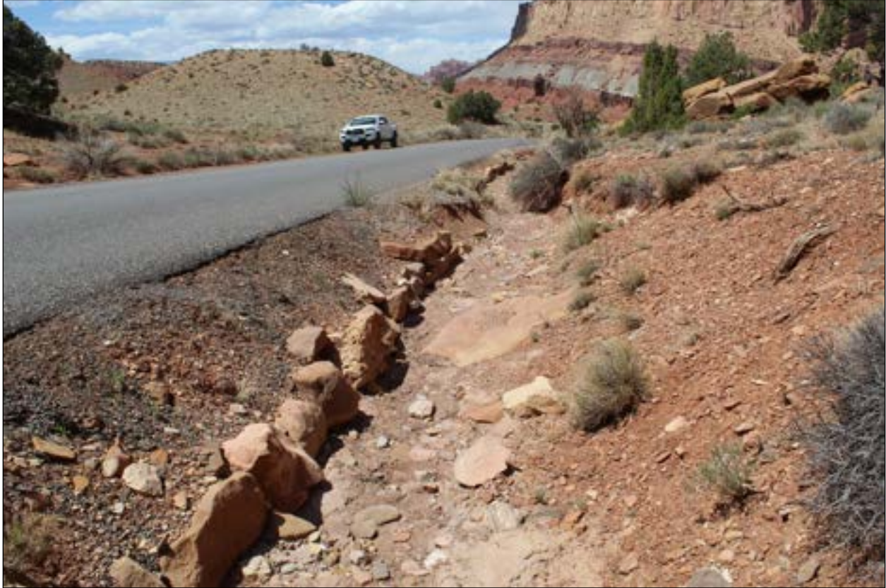
Photo 021. Ditches line many sections of Scenic Drive to carry water toward the washes. However, because they have been excavated repeatedly over decades, it is not known which may be historic. View to the north.
