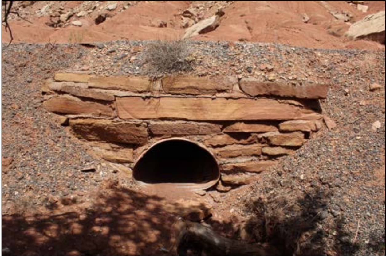
Photo 009. Culverts built during the Mission 66 era feature headwalls with roughly squared and coursed sandstone blocks, all of which are smaller than the blocks used by the CCC/WPA. View to the east of the culvert at milepost 6.75.
