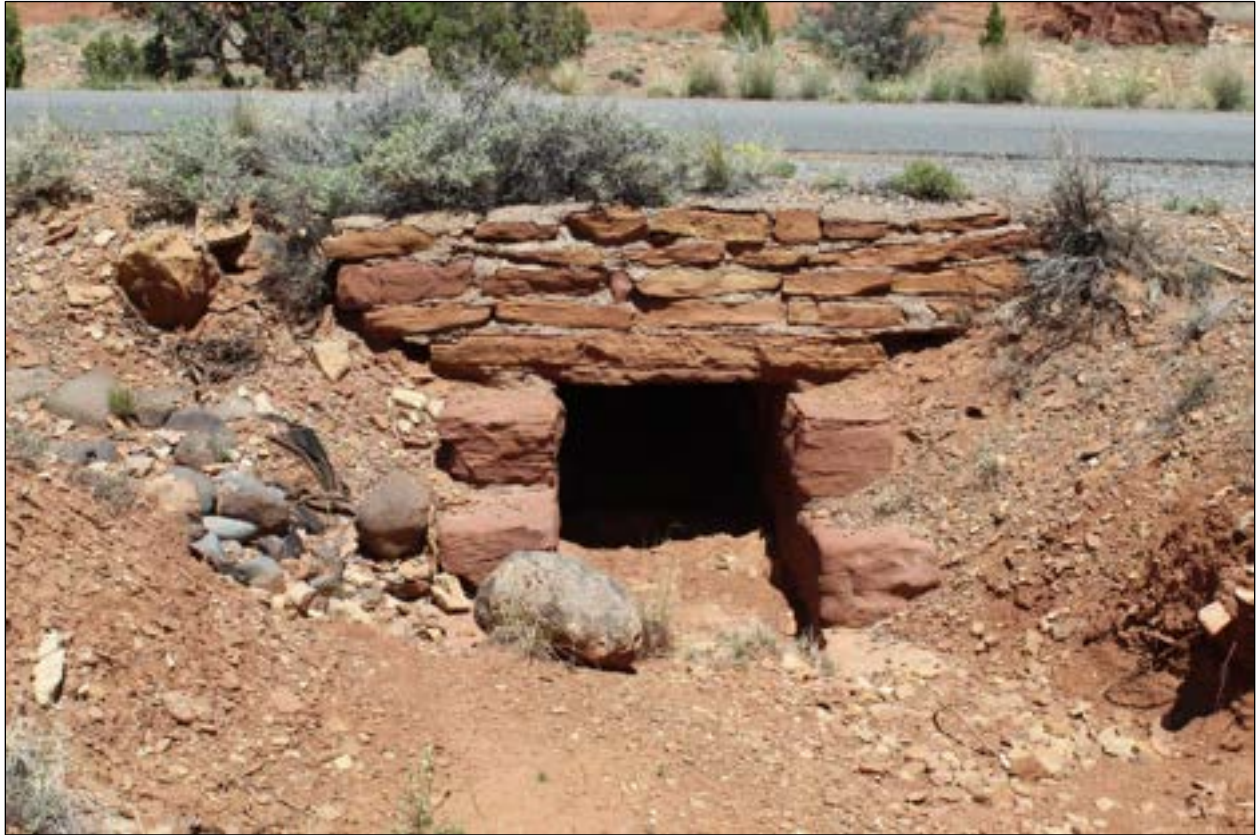
Photo 008. Some culverts appear to have been originally built during the WPA era but rebuilt during the Mission 66 era, such as this one at milepost 3.30. Its headwall's lower courses are large, squared sandstone blocks characteristic of the CCC and WPA work, whereas the upper courses are smaller and more roughly squared, indicative of Mission 66 construction. View to the east.
