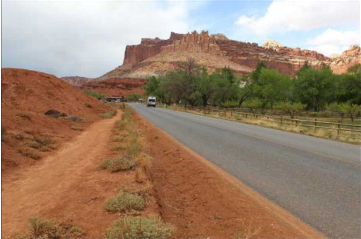
Photo 001. At its northern end, Scenic Drive passes through the Fruita Rural Historic District, where it is a two-lane, asphalt-paved road with a painted centerline. View to the north-northwest.
