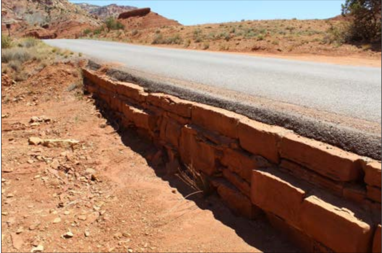
Photo 010. Three low-water crossings along Scenic Drive were likely built by the CCC or WPA. These crossings are constructed of large, squared sandstone blocks similar to those used for the box culverts and culvert headwalls. View to the southwest of the low-water crossing at milepost 3.33.
