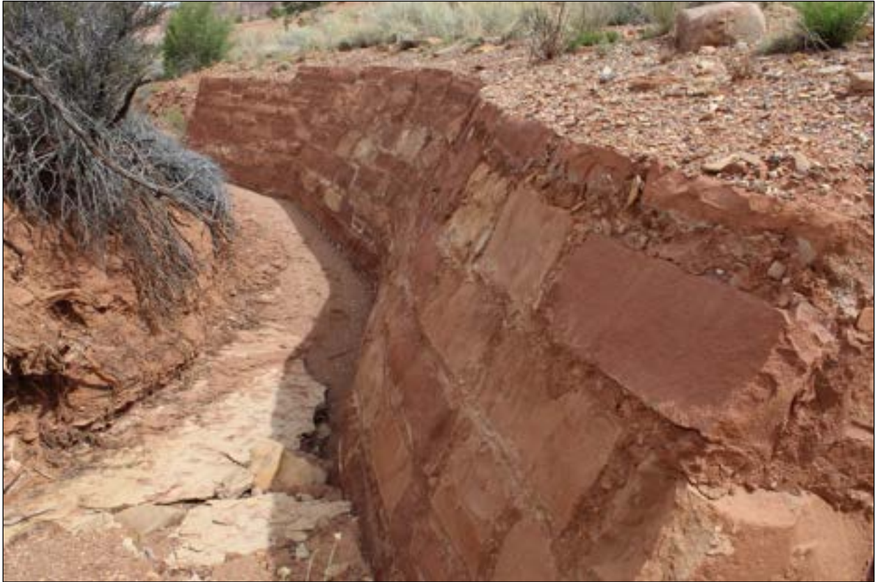
Photo 011. Four sandstone retaining walls that line Scenic Drive were built in 2010-2011 as part of the rock embankment project. View to the northeast of the retaining wall at milepost 5.69.
