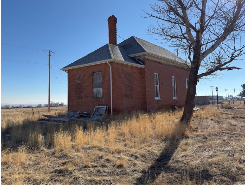
Photograph 7 of 19. Exterior, north and west facades. Camera facing southeast.
