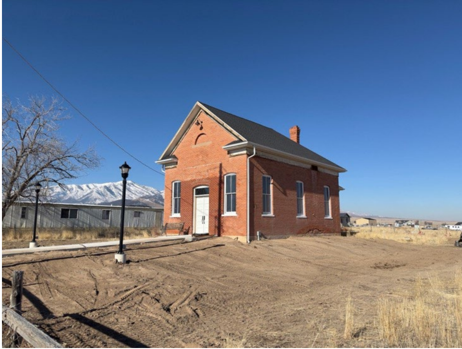
Photograph 3 of 19. Exterior, east and south (main) façades. Camera facing northwest.
