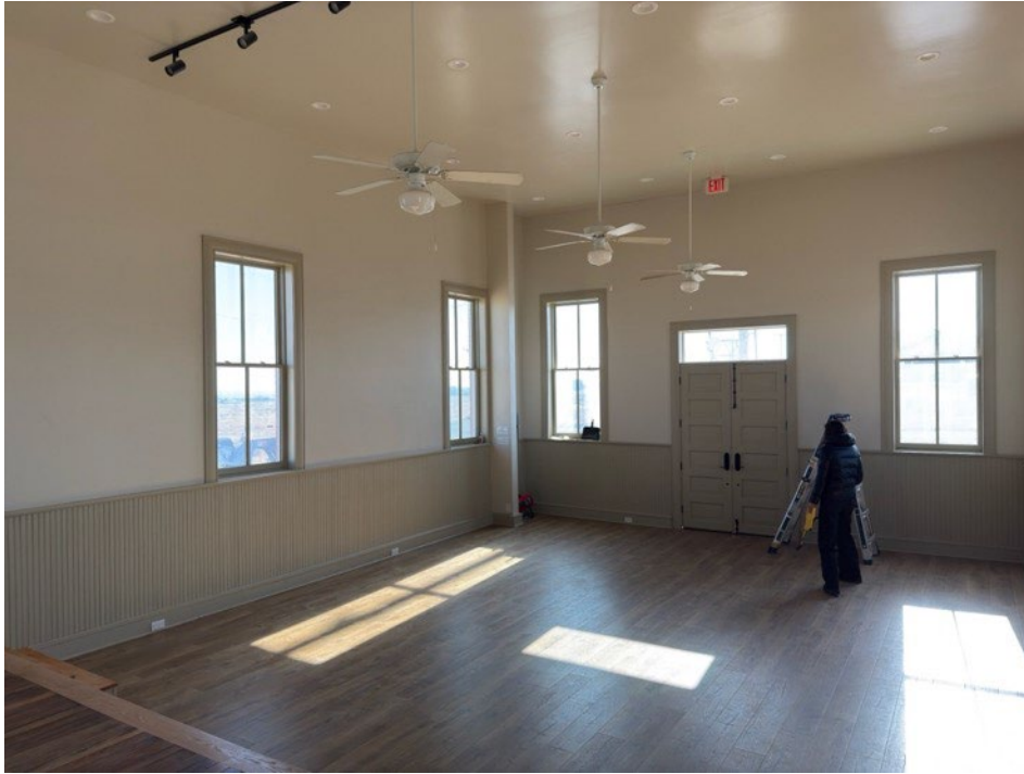
Photograph 15 of 19. Interior, showing lighting and replaced windows. Camera facing southeast.
