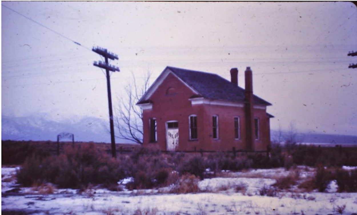
Figure 4 of 14. Clover Meetinghouse, ca. 1960. Note the power lines, replaced entryway doors, and removal of the bell tower. Camera facing northwest. Source: John Cluff.
