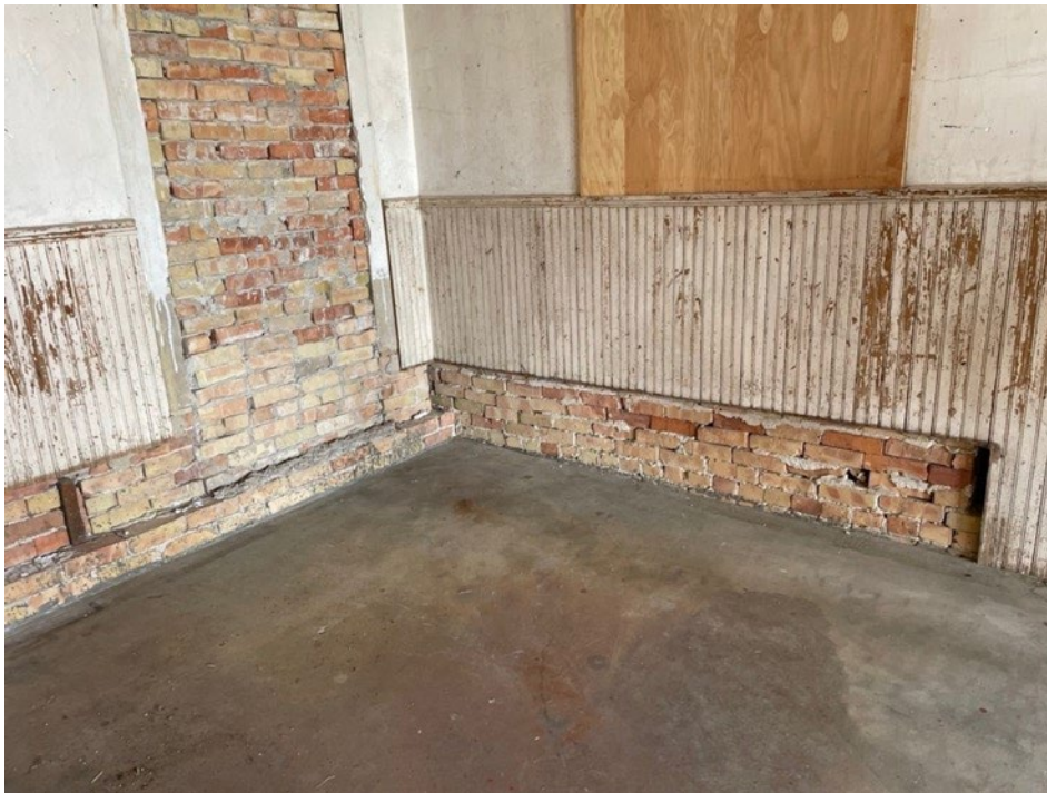
Figure 12 of 14. Photograph of the stage area prior to reconstruction, ca. 2022. Note the extant “ghost lines” of the original stage and the bricked doorway. Camera facing northeast. Source: Clover Church Restoration Committee.
