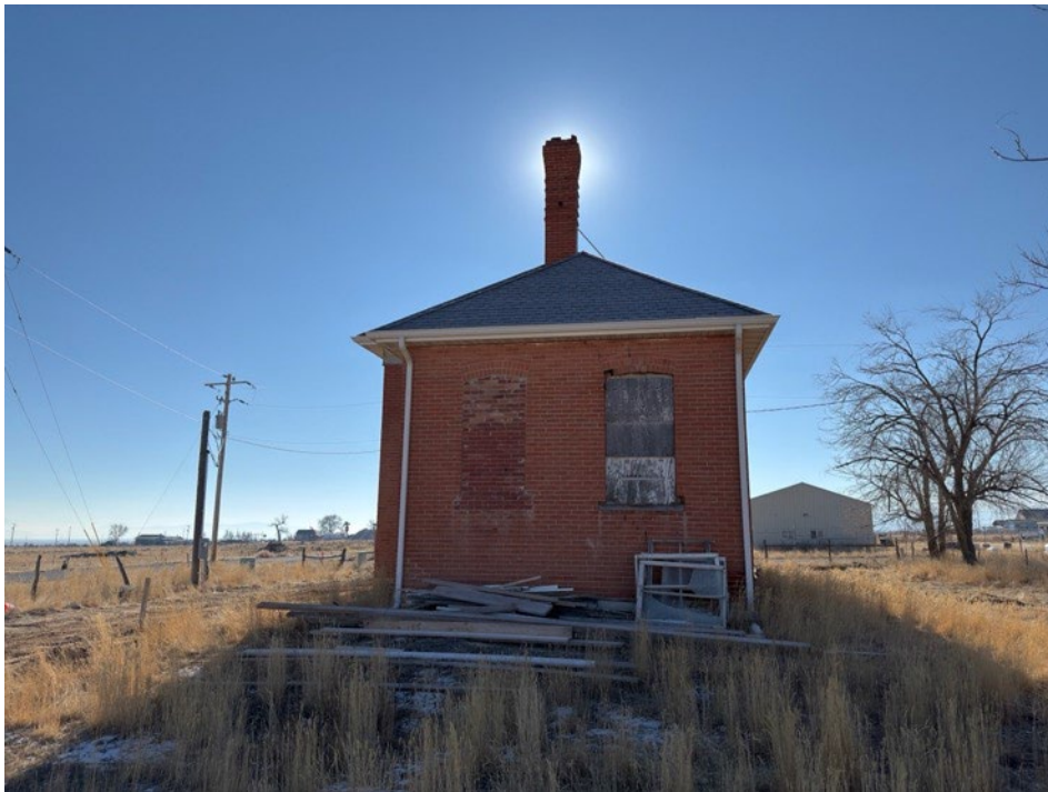
Photograph 8 of 19. Exterior, north facade. Camera facing south.
