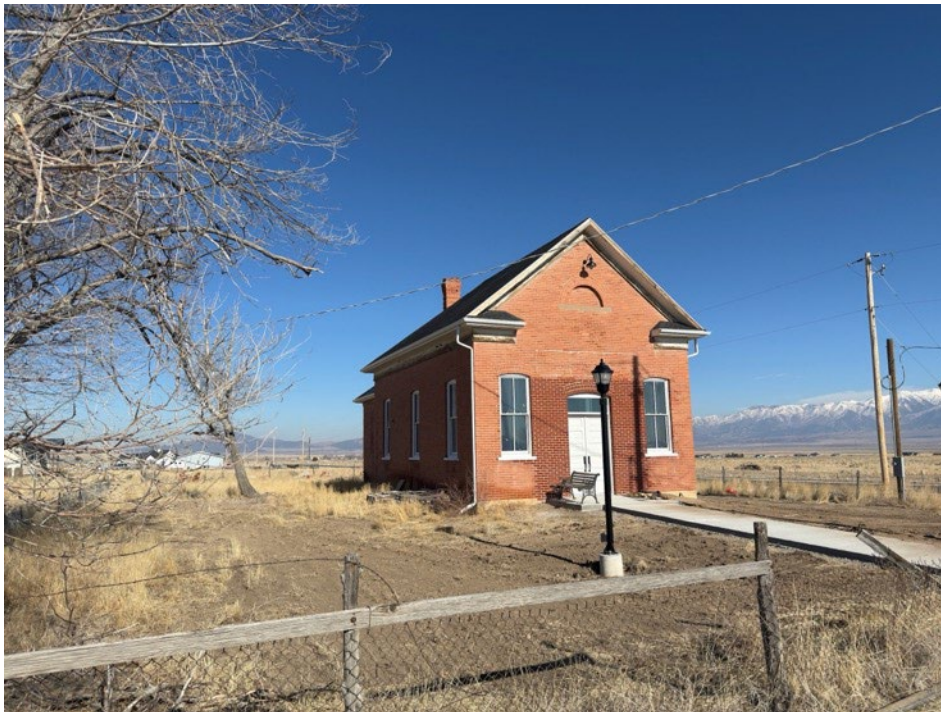
Photograph 2 of 19. Exterior, west and south (main) facades. Camera facing northeast.
