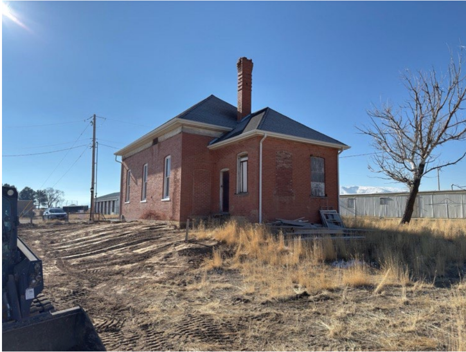
Photograph 9 of 19. Exterior, west and north (rear) facades. Camera facing southwest.
