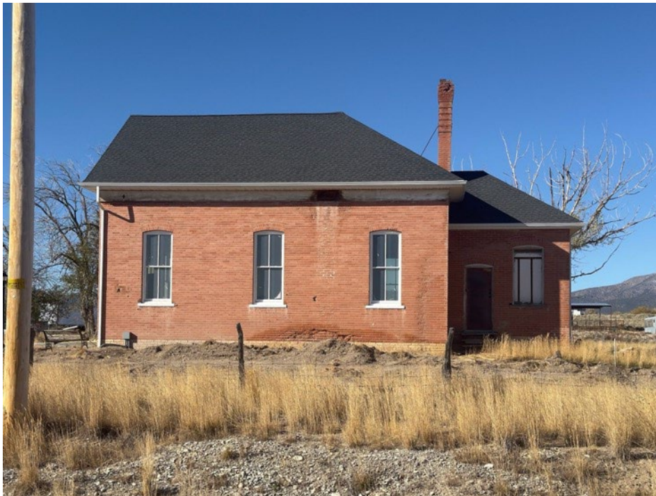
Photograph 10 of 19. Exterior, east facade. Camera facing west.
