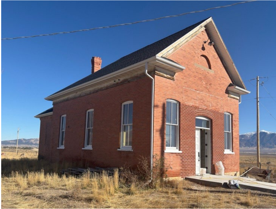
Photograph 5 of 19. Exterior, west and south (main) facades. Camera facing northeast.
