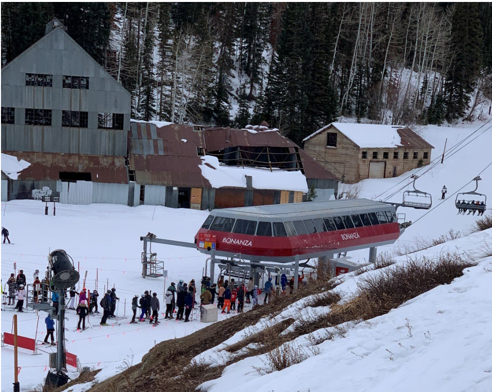
Photo No. 45 South elevation of Bonanza Chairlift with Shaft House and Change House in background. Camera facing south.
