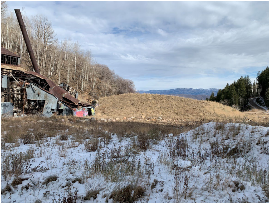
Photo No. 37 West elevation of Dorr Thickener Tank with Silver King Mill on left. Camera facing east.
