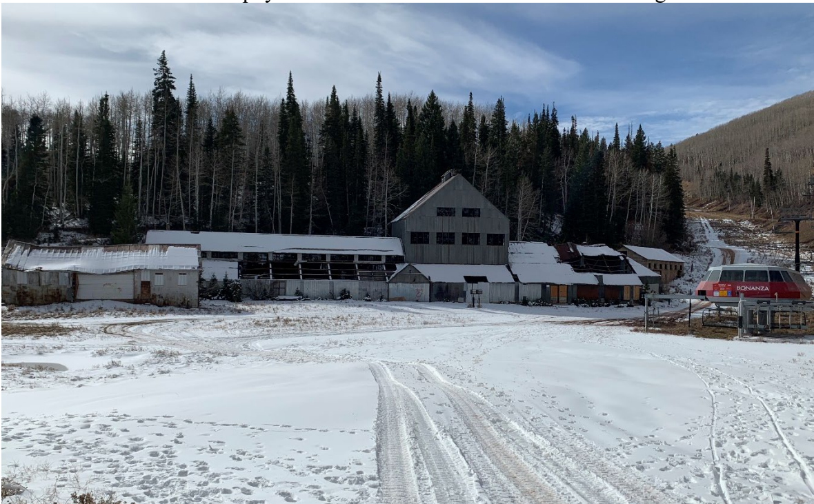
Photo No. 2 Overview and physical environment of the site. Camera facing south
