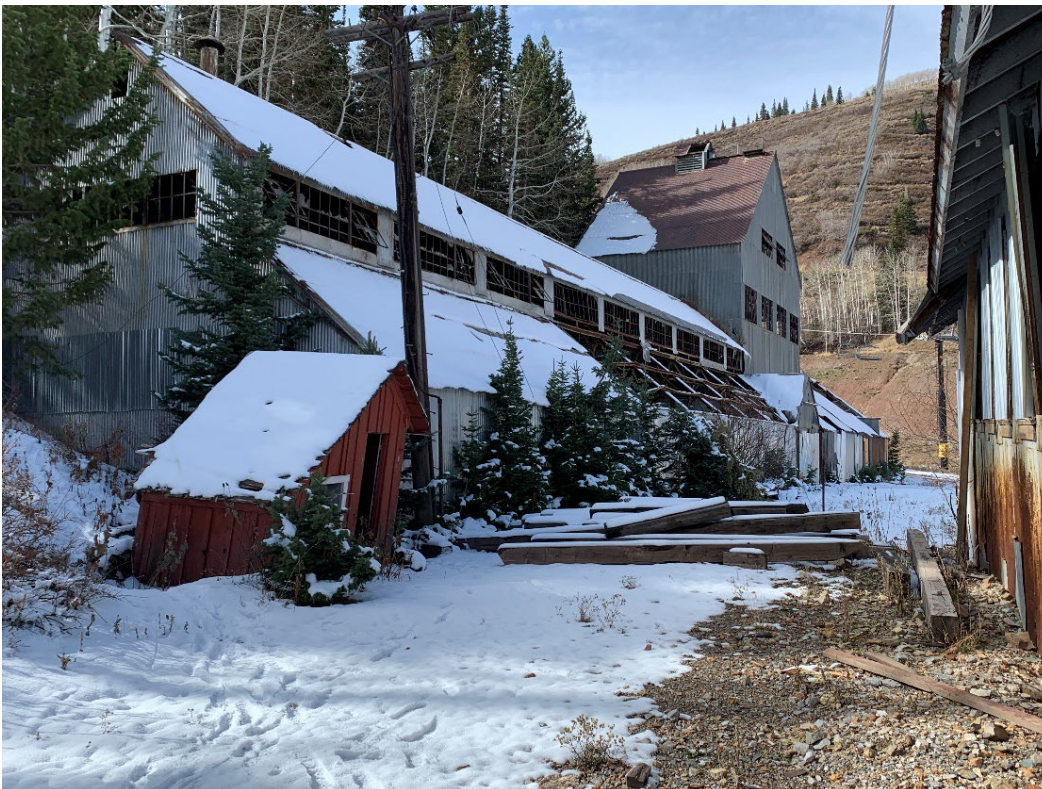
Photo No. 9 East and north elevations of the Silver King Shaft House. Camera facing west
