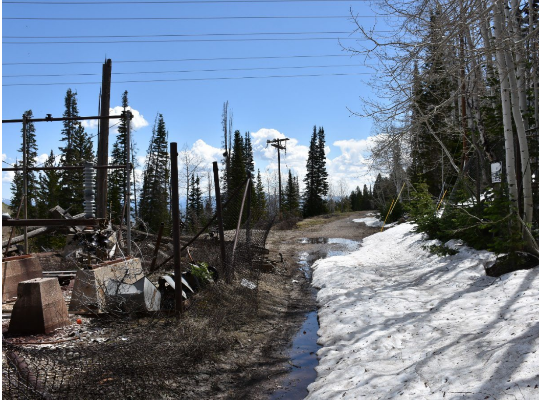
Photo No. 48 Haul Road heading east to waste dump (on the right and beyond the substation). Camera facing east.
