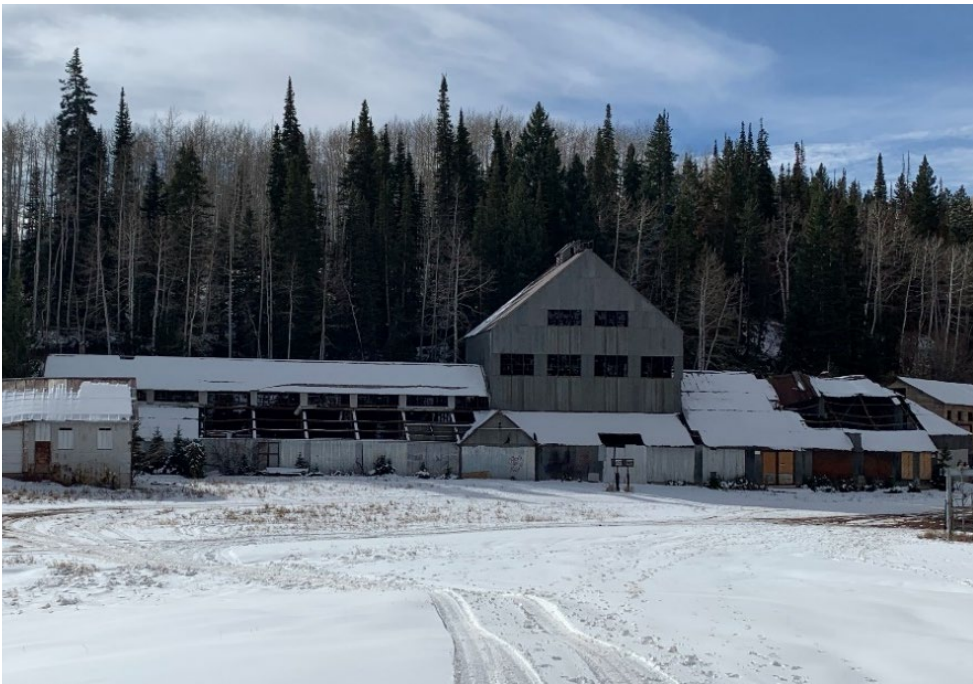
Photo No. 6 North (primary) elevation of the Silver King Shaft House. Camera facing south
