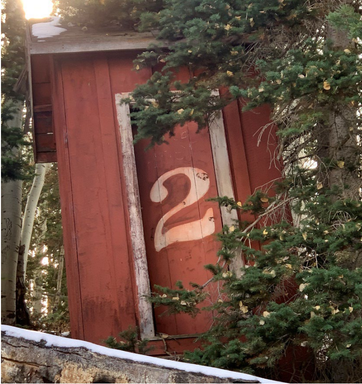
Photo No. 34 North elevation of Fire Hose Shack 2. Camera facing south
