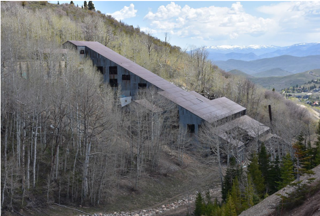
Photo No. 19 West elevation of Silver King Mill. Camera facing east.
