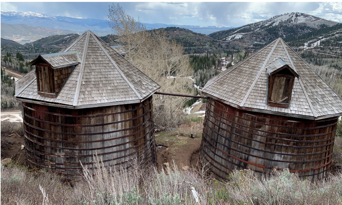
Photo No. 29 West elevation of water Tanks A & B. Camera facing east
