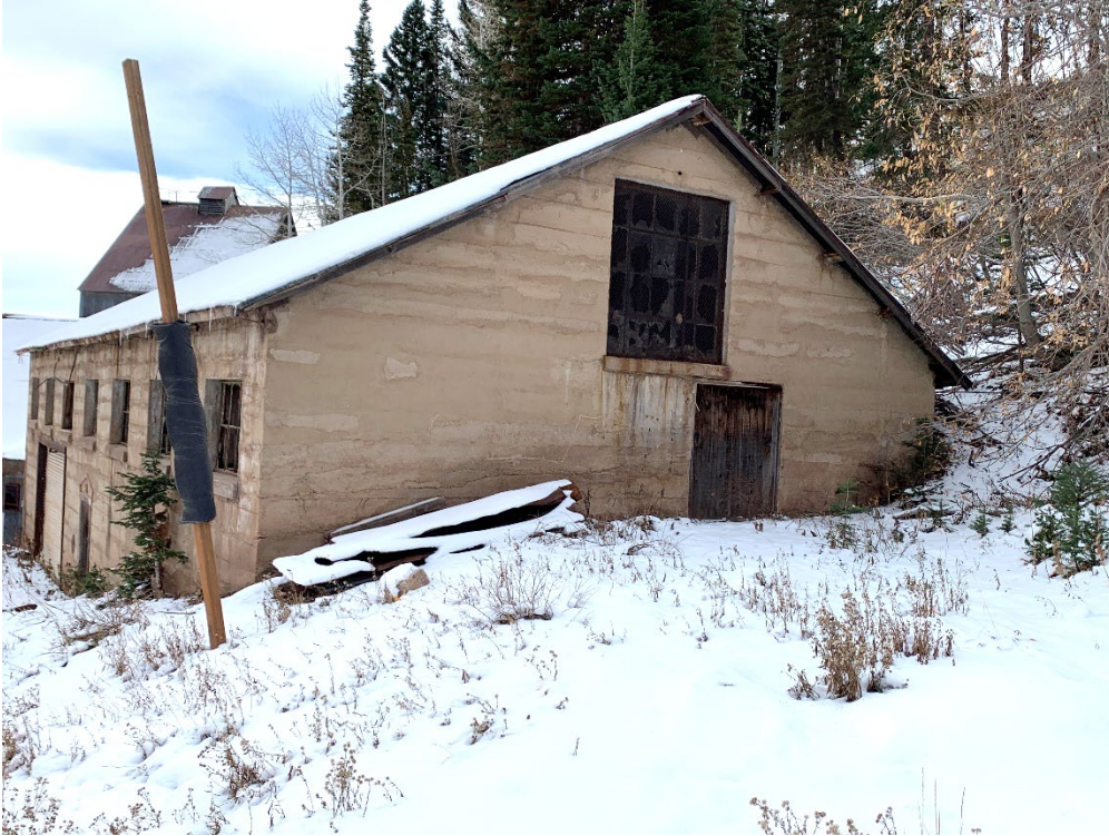
Photo No. 12 West elevation of the Change House. Camera facing north-east
