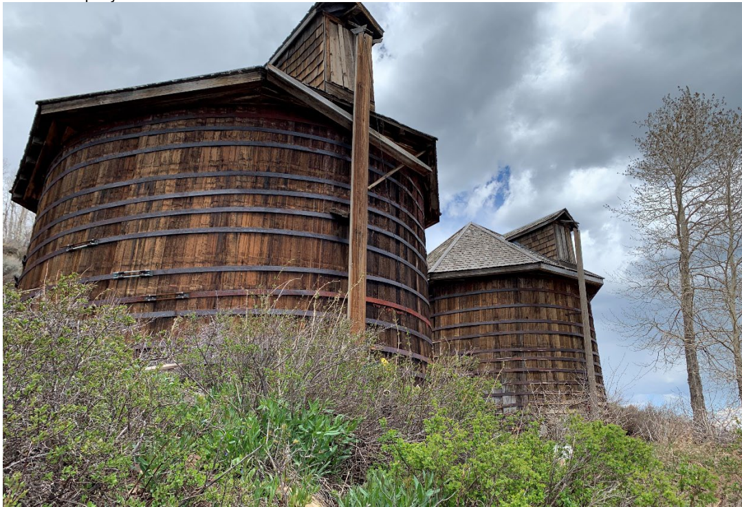
Photo No. 30 East elevation of water Tanks A & B. Camera facing northwest.
