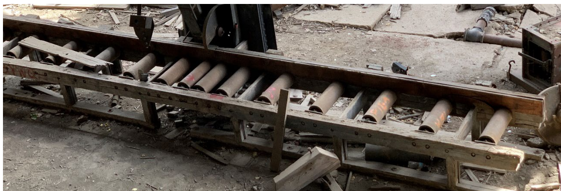
Figure 13. A timber frame holds the rollers of this conveyor, while other conveyors remaining in the mill feature a steel frame. Source: Sandra Morrison, 2023.
