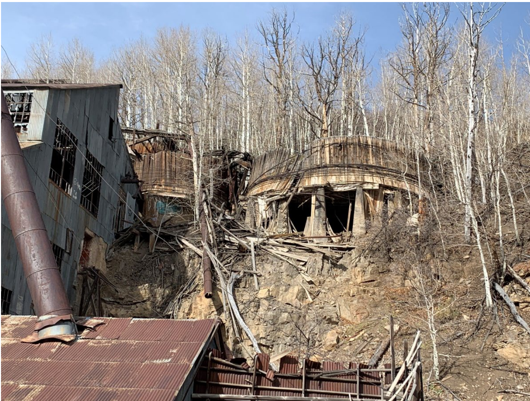
Photo No. 39 South elevation of Silver King Mill Water Tank. Camera facing north
