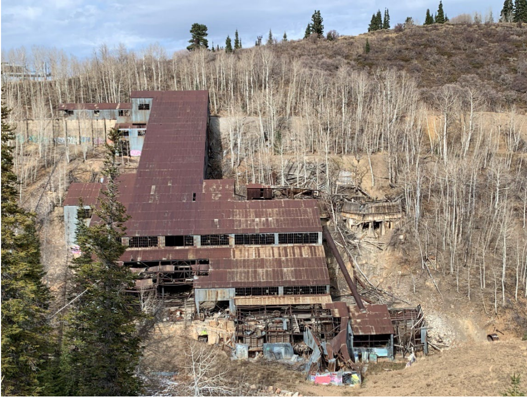
Photo No. 18 South (primary) elevation of the Silver King Mill. Camera facing north
