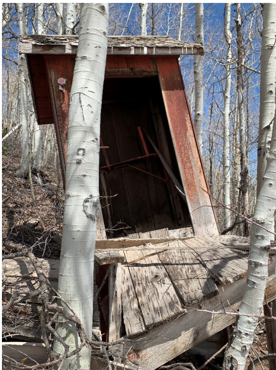
Photo No. 41 South elevation of Mill Fire Hose Shack 2. Camera facing north
