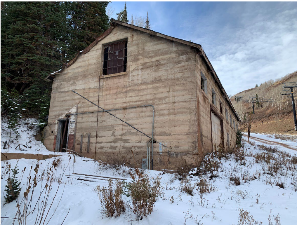
Photo No. 11 East elevation of the Change House. Camera facing south-west
