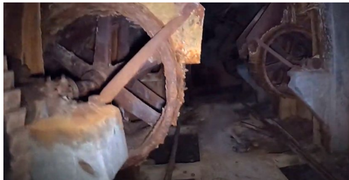
Figure 11: Eight-inch roll-type feeders controlled the passage of ore onto the conveyor belt (visible center). Source: Sandra Morrison 2024.
