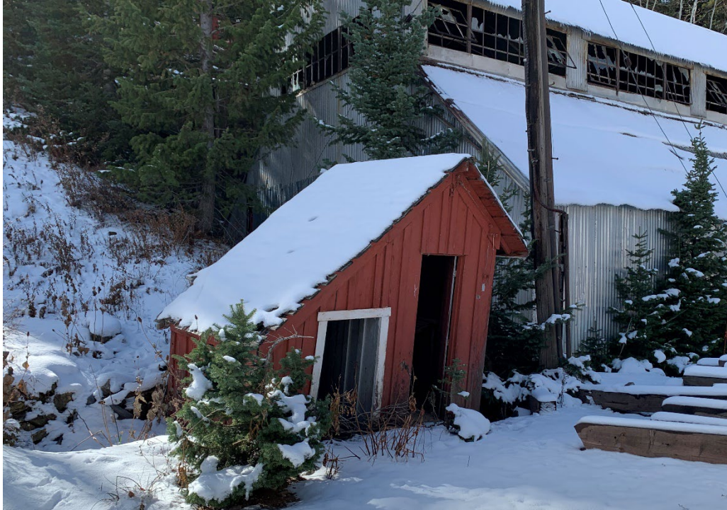
Photo No. 36 North elevation of Fire Hose Shack 4. Camera facing south
