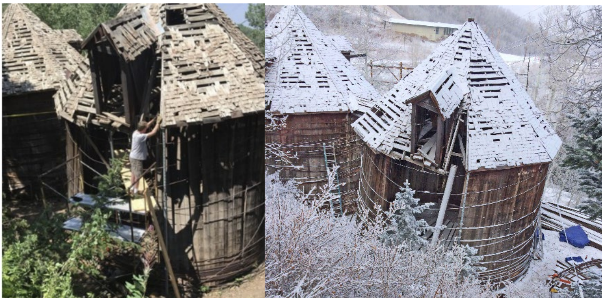
Figures 7 & 8. Two images of Water Tanks D & E before stabilization work. Source: Friends of Ski Mountain Mining History and Lance Kincaid. 2019.
