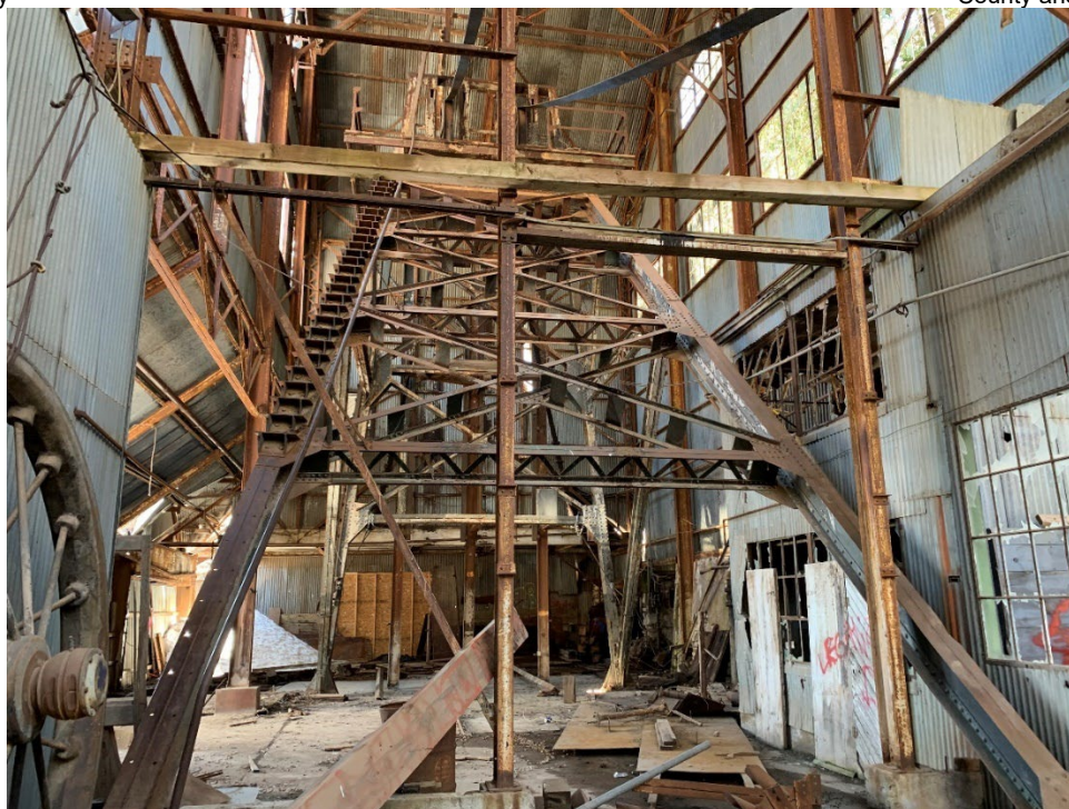
Figure 3. The 62-foot tall headframe located in the middle section of the Shaft House. Source: Sandra Morrison 2024.
