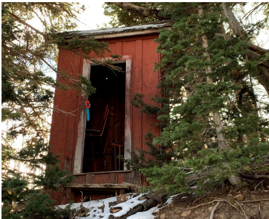
Photo No. 33 North elevation of Fire Hose Shack 1. Camera facing south
