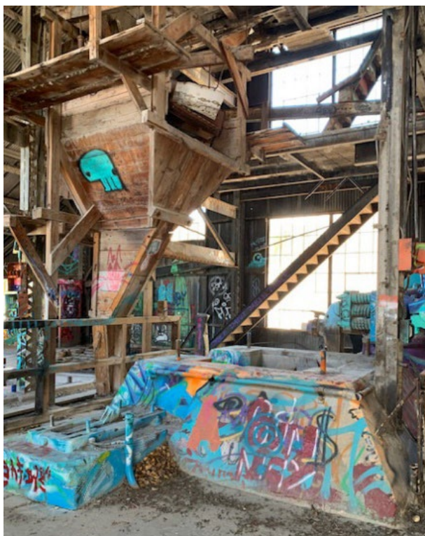
Figure 15. Cone Crusher feeder and foundation. Source: Sandra Morrison, 2024.
