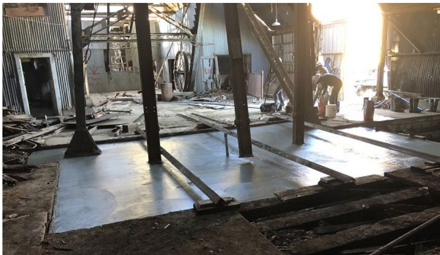
Figure 26. Capping of the Silver King 3-compartment shaft in the summer of 2023. Source: Brian Buck, Friends of Ski Mining Mountain History. 2023
