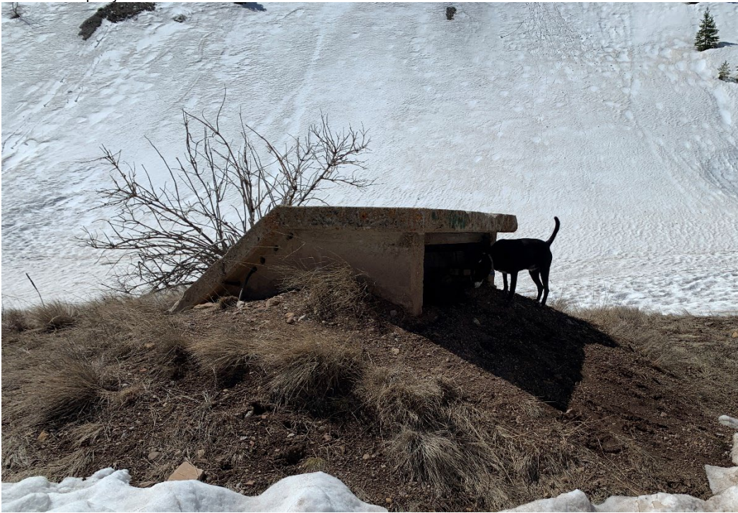
Photo No. 38 North elevation of Dorr Thickener Tank entrance with waste dump in background. Camera facing south.
