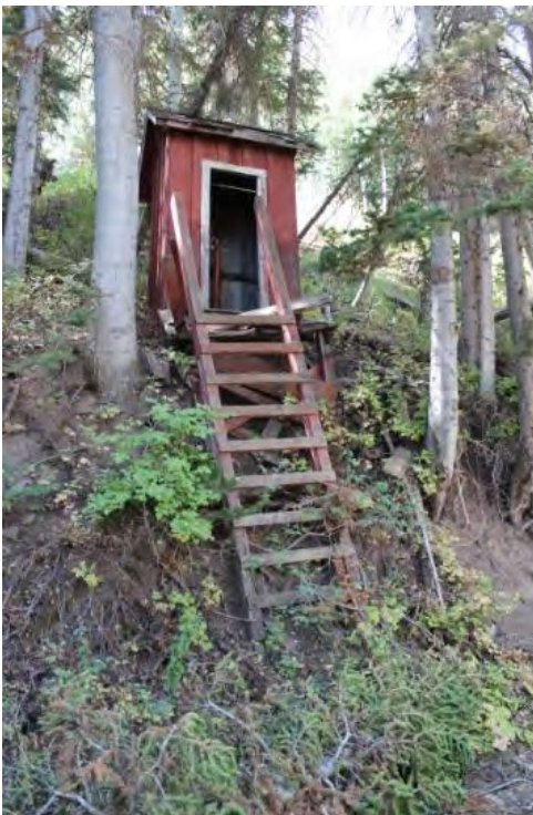
Photo No. 35 North elevation of Fire Hose Shack 3. Camera facing south.
