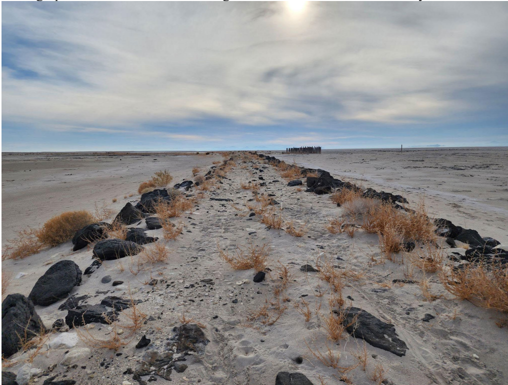
Photograph 19. Rozel Oil Field jetty. Camera view facing west.
