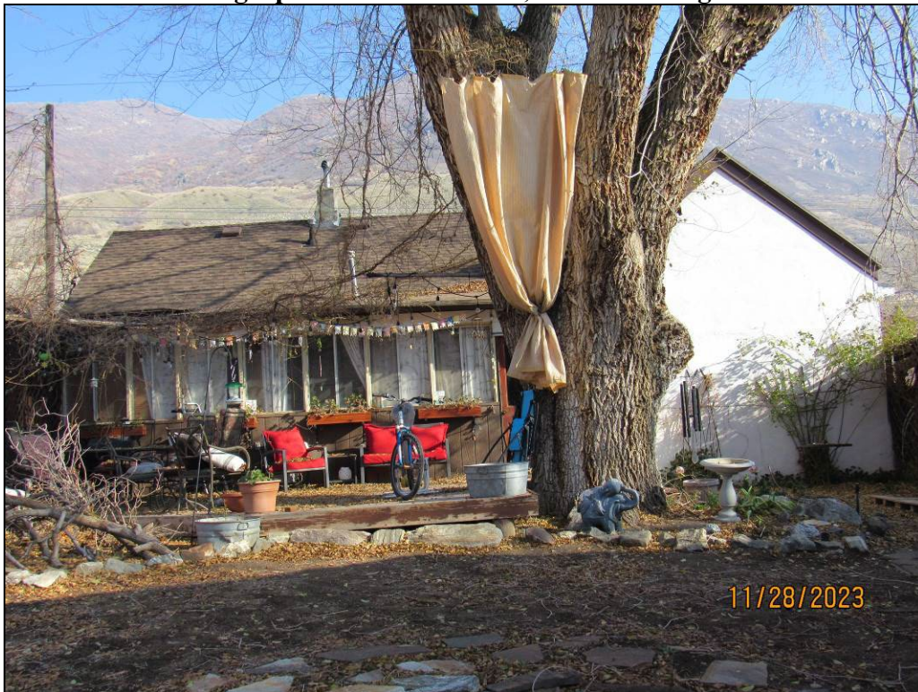
Photograph 8. West elevation; camera facing east
