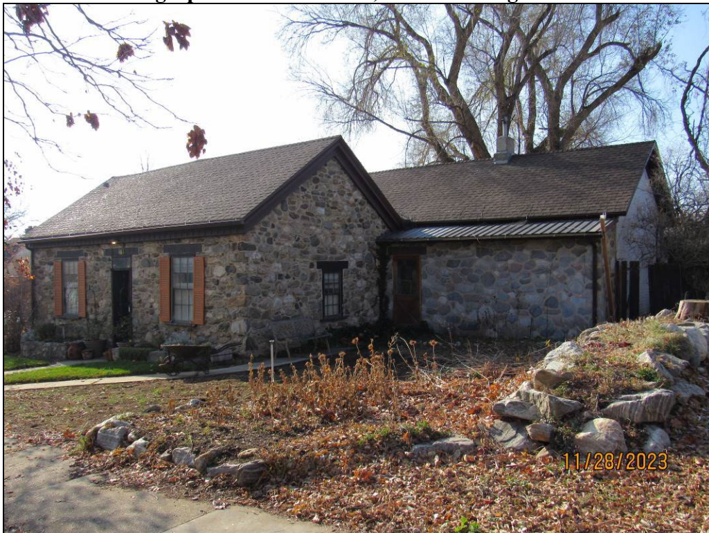
Photograph 4. East elevation; camera facing southwest
