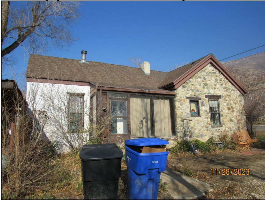
Photograph 7. South elevation; camera facing north-northeast
