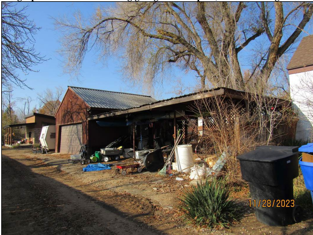
Photograph 11. Non-contributing garage and carport; camera facing northwest
