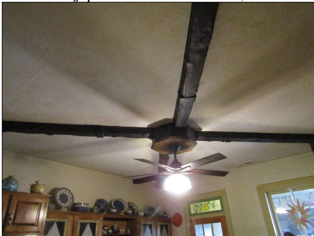
Photograph 14. Faux timber beams in kitchen; detail
