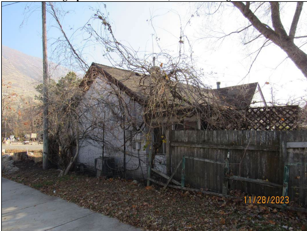
Photograph 10. North elevation; camera facing southeast
