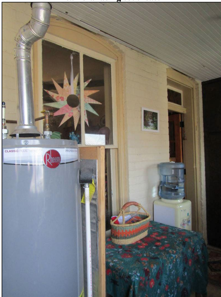
Photograph 15. Original brick wall from rear addition enclosed in second addition; camera facing southeast
