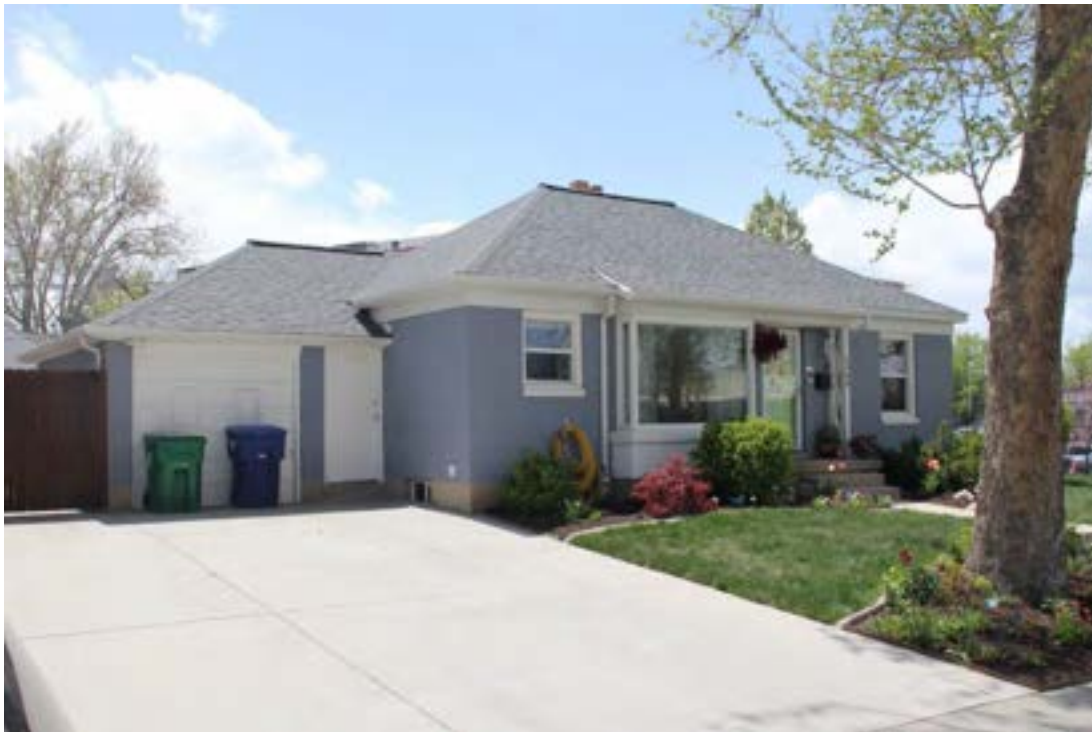
Photo 6. The Montgomery Ward collaboration house at 1368 East 3010 South. Camera facing southwest.
