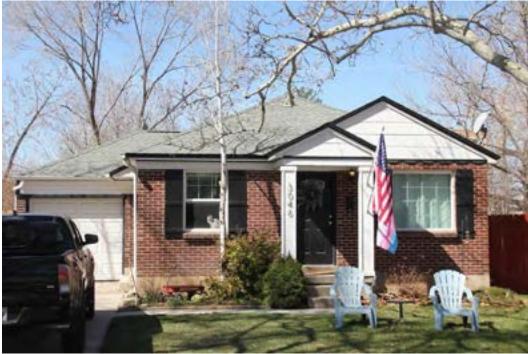
Photo 19. Variation of intersecting hipped roofs with a front gable and attached garage located at 3046 S. Crescent Dr. Camera facing west.
