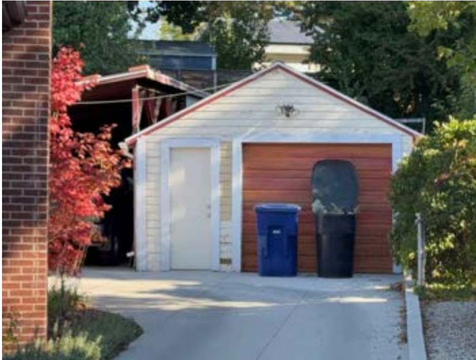
Photo 31. Example of a contributing single bay garage with an attached shed at 1639 East 3010 South. Camera facing east.
