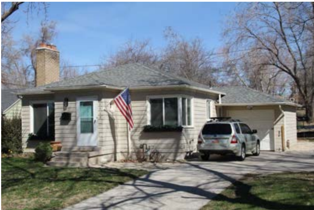
Photo 18. Variation of a hipped roof asymmetrical form with attached garage located at 1415 East 3010 South. Camera facing north.
