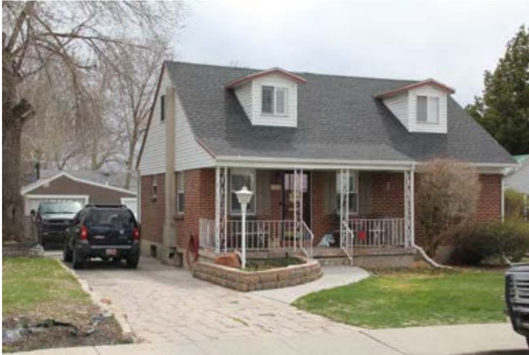
Photo 21. The house at 1602 East 3010 South is the singular example of a rooftop addition in the neighborhood. Camera facing south.
