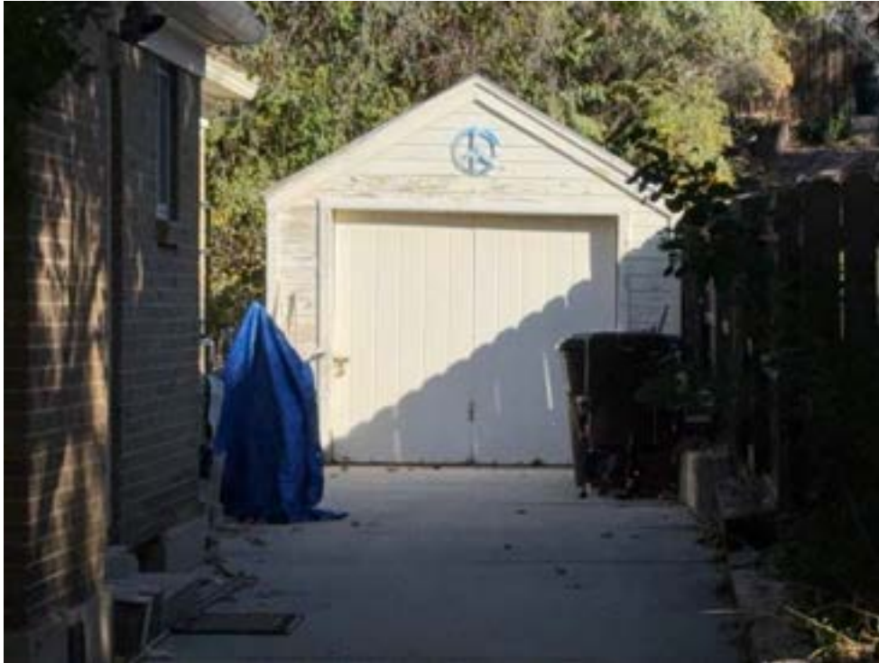
Photo 27. Example of a contributing single bay garage constructed of wood at 1443 East 3010 South. Camera facing north.
