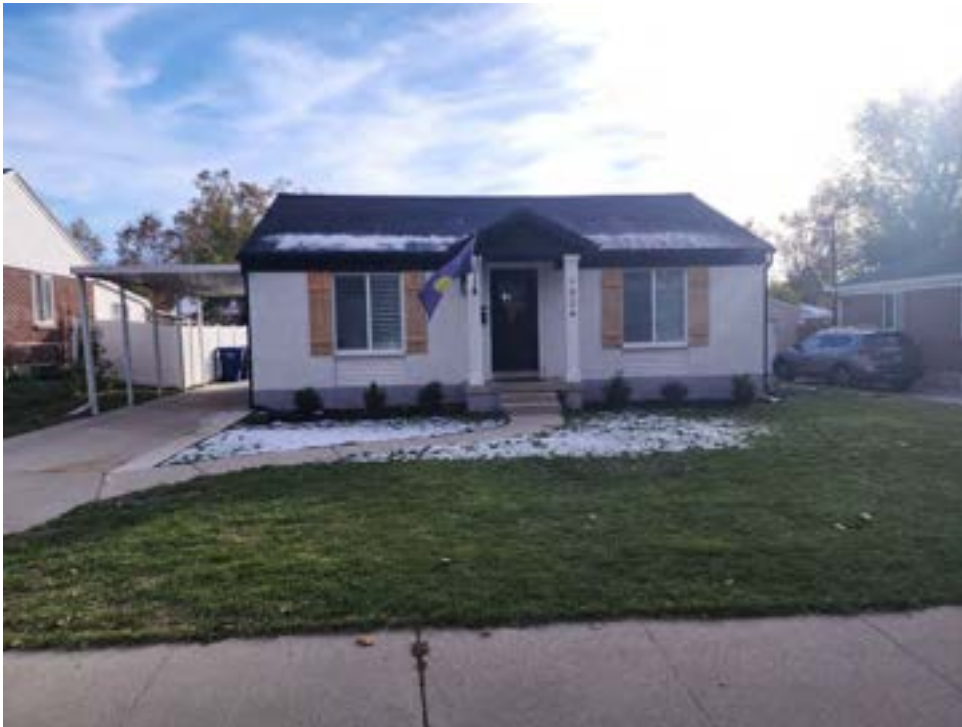
Photo 48. A flat attached carport example at 1524 S. Gregson Ave. Camera facing south.
