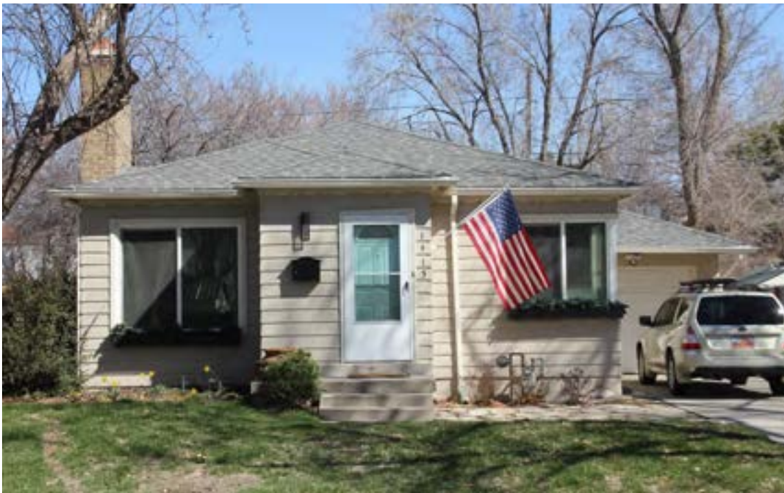
Photo 38. An example of an asymmetrical Ranch with extended front entry under a separate hipped roof at 3010 S. 1415 E. Camera is facing north.
