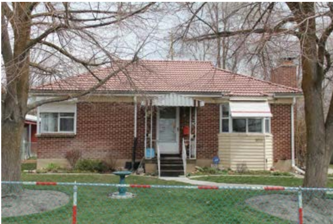
Photo 16. Variation of a hipped roof asymmetrical form located at 3023 South 1640 East. Camera facing east.
