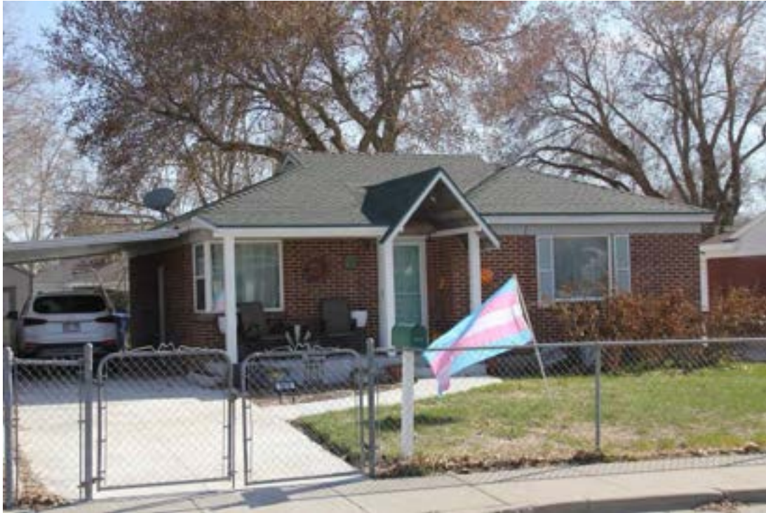
Photo 9. Located at 1612 East 3115 South is the 1949 model house. Camera facing south.
