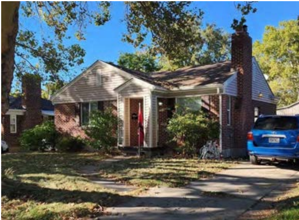
Photo 22. The new siding in the gables and onto the portico and columns has compromised the integrity of the house at 1477 East 3150 South. Camera facing north.
