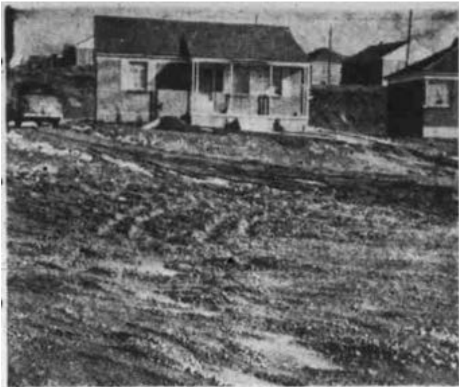
Figure 9. Poor condition of clay roads in Mountair Acres shown in the Deseret News , February 26, 1948.
