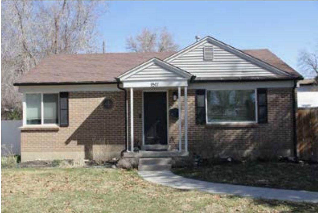
Photo 13. The residence at 1517 East 3010 South, is a Minimal Traditional style example with a double front gable accent, and circular, corner (meeting), and picture windows, along with a small porch as a unique combination of features. Camera facing north.
