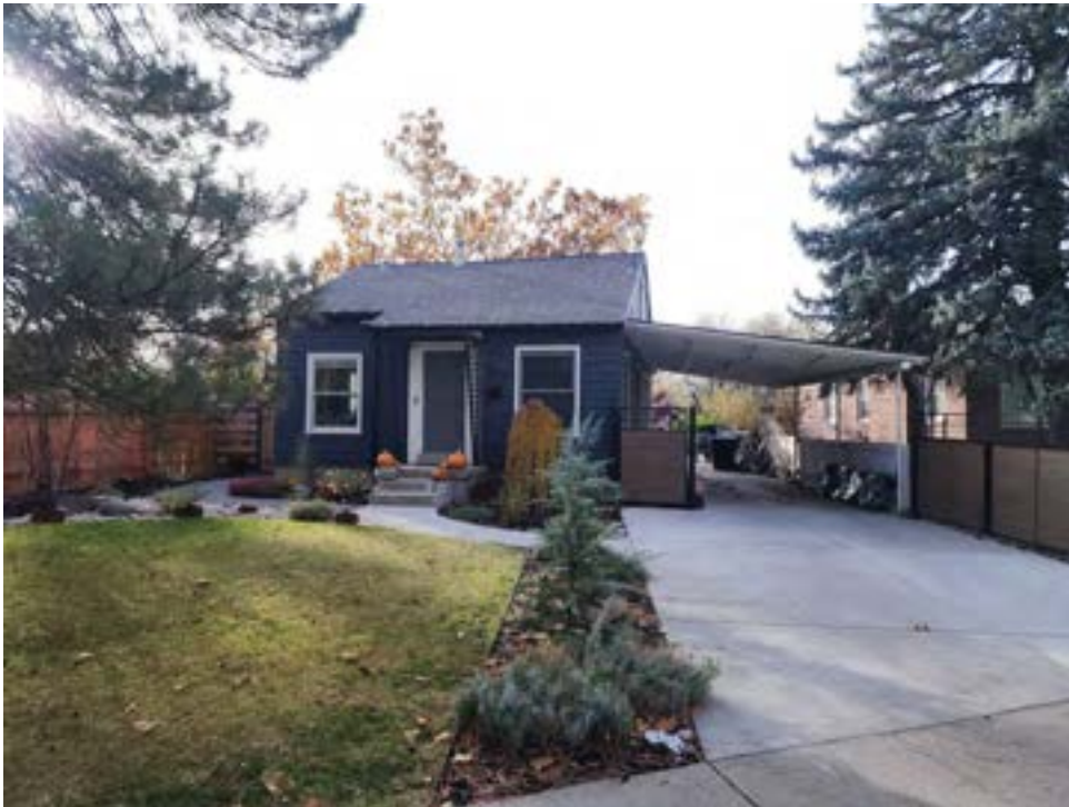
Photo 46. An angled attached carport at 3040 S. Crescent Dr. Camera facing west.
