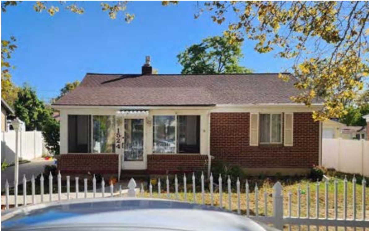
Photo 26. The infilled porch at 1524 East 3045 South is the primary alteration that made this building non-contributing. Camera facing south.
