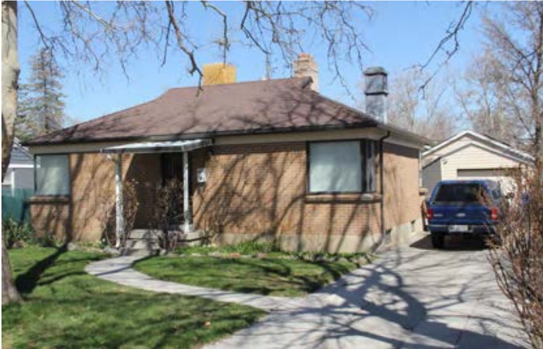
Photo 39. An example of an asymmetrical form Ranch with a hipped roof and pop at the top to allow for ridge vents at 1517 E 3045 S. Camera facing north.
