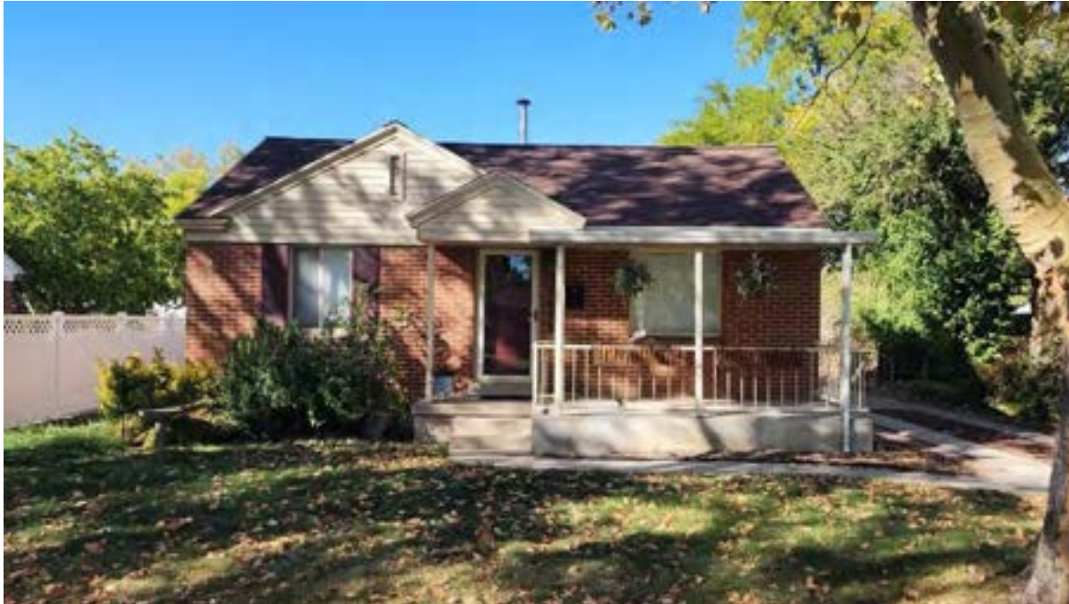
Photo 25. The house at 1525 E. Gregson Ave. has had a concrete porch addition to the front of the house, creating a non-contributing evaluation. Camera facing north.
