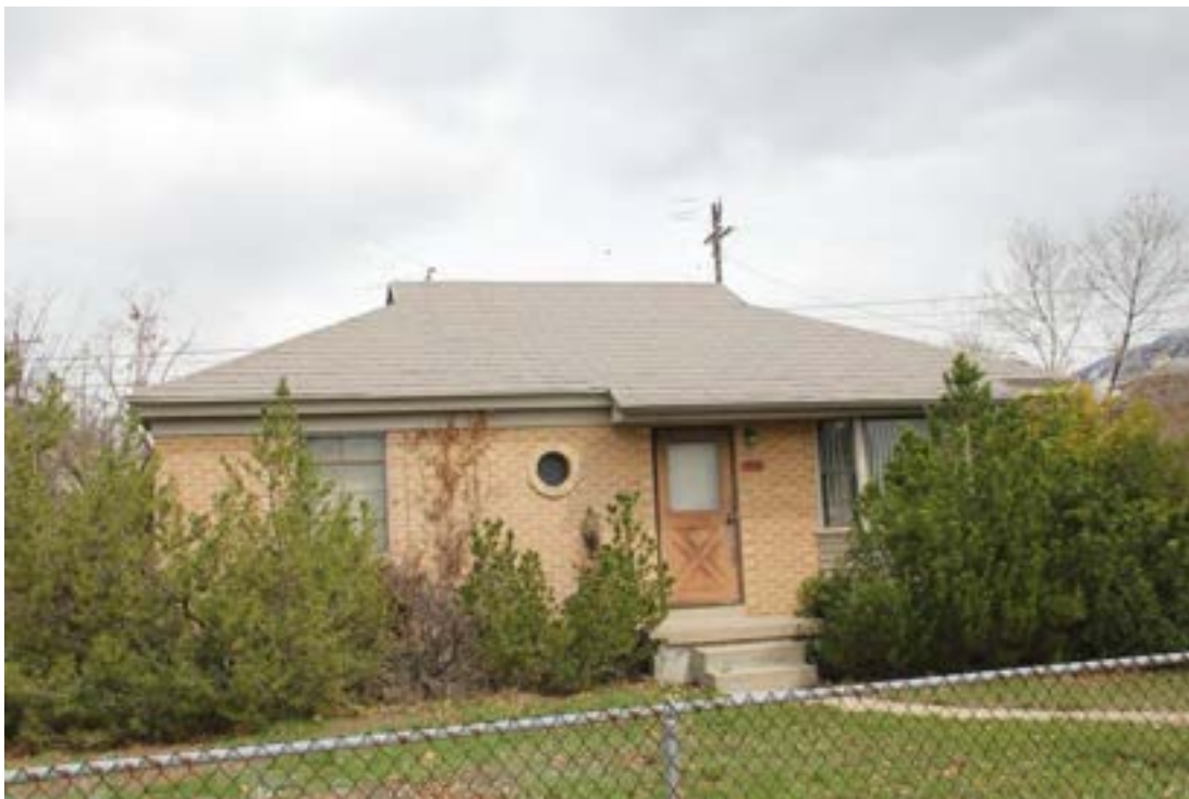
Photo 10. The residence at 3009 South 1640 East, an Early Ranch style house, displays a bay window and circular window with the discernable hipped roof popped at the top with side ridge vents. Camera facing east.
