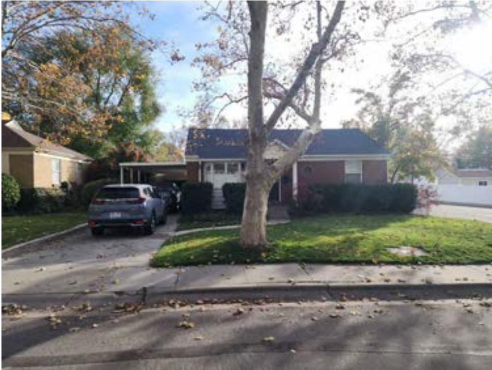
Photo 45. A flat attached carport at 1526 E. Gregson Ave. Camera facing south.
