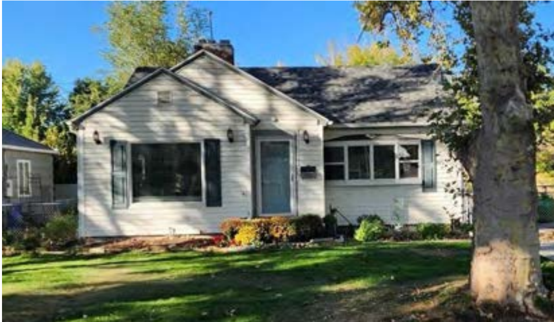
Photo 23. The major window alteration to install the bay window rendered this building at 1427 East 3010 South non-contributing. Camera facing north.
