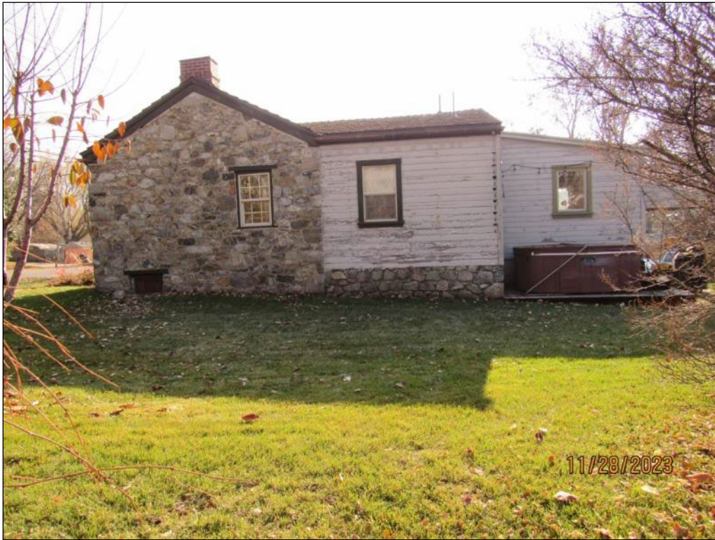
Photograph 7. North elevation; camera facing south
