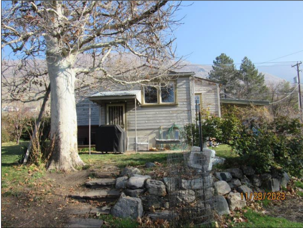
Photograph 5. West elevation; camera facing east
