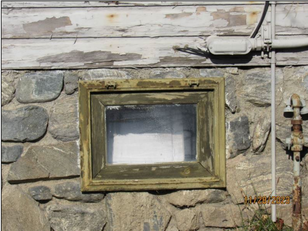
Photograph 10. Basement window detail in rear addition; camera facing east
