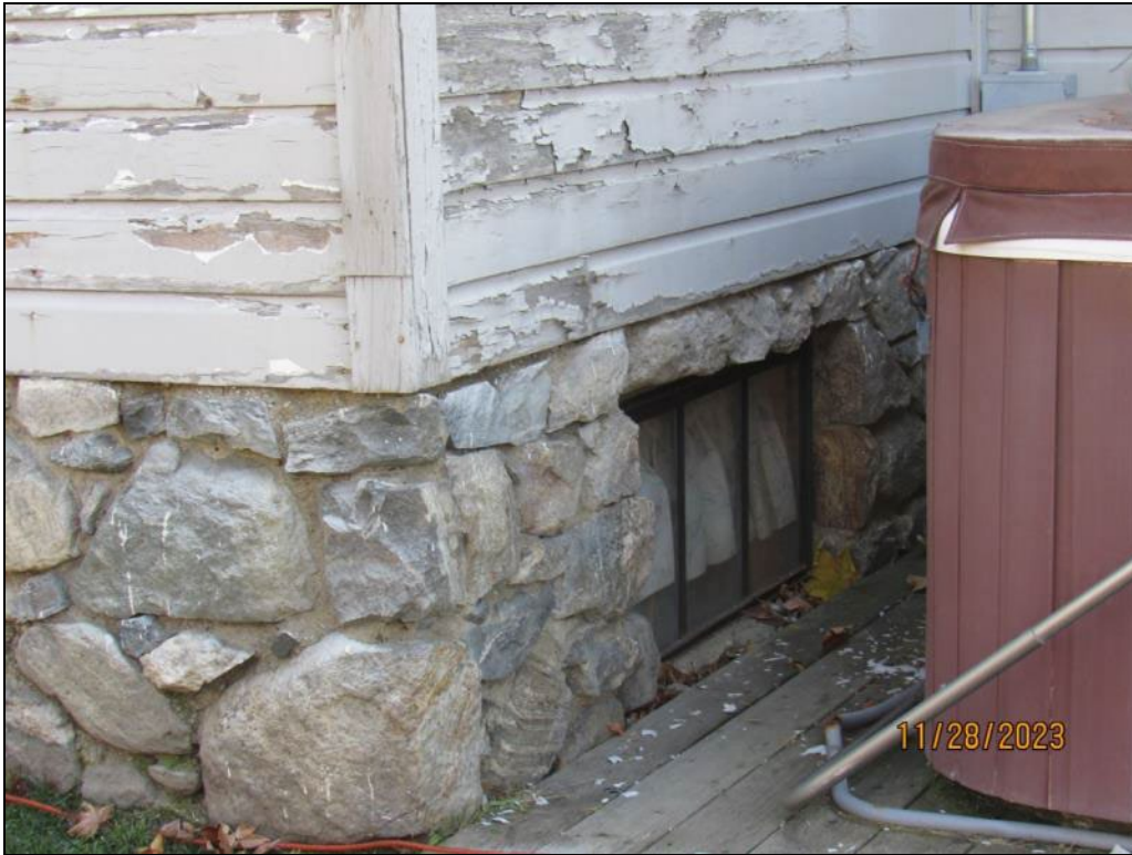
Photograph 9. Foundation detail for rear addition; camera facing east-northeast
