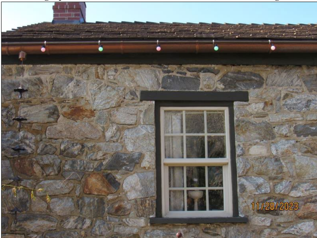
Photograph 8. Window detail in east elevation; camera facing west
