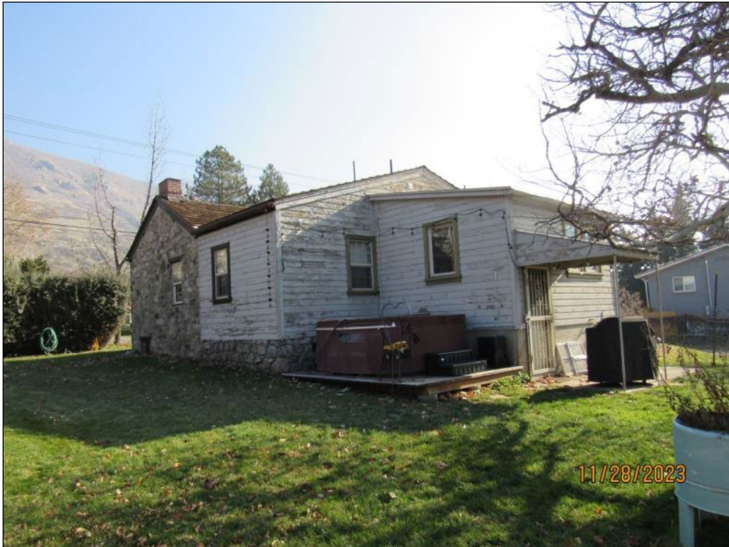
Photograph 6. North (at left) and west (at center) elevations; camera facing southeast
