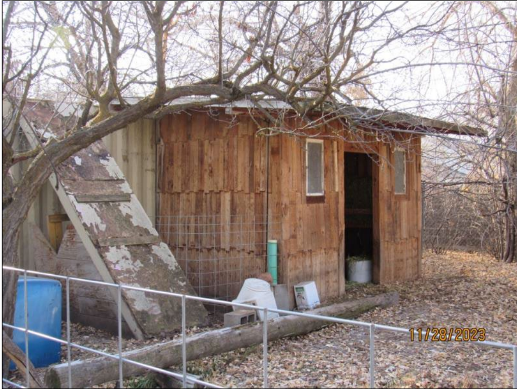
Photograph 19. Non-contributing animal sheds/shelters; camera facing southwest
