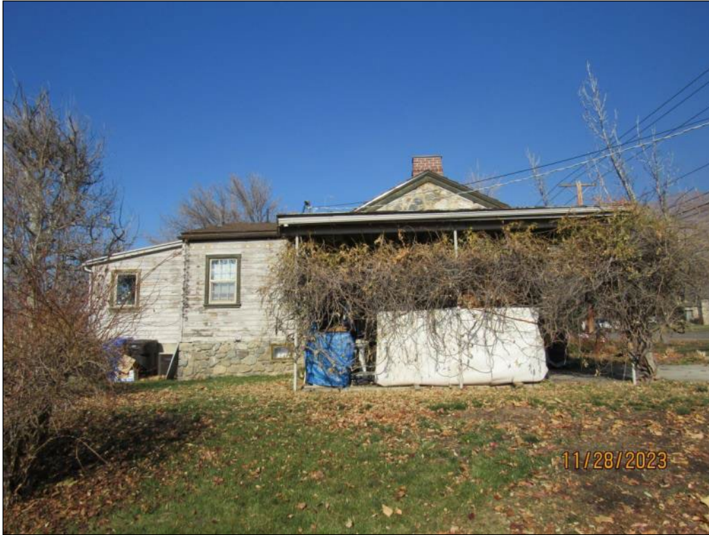
Photograph 3. South elevation; camera facing north
