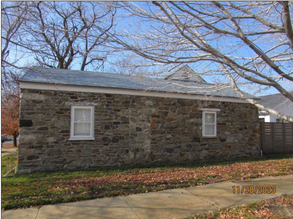
Photograph 2. East elevation (primary façade); camera facing west
