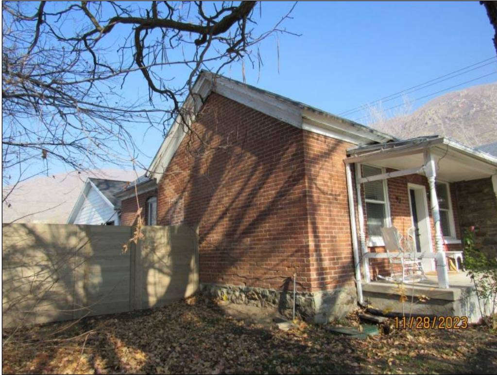
Photograph 5. West elevation; camera facing northeast
