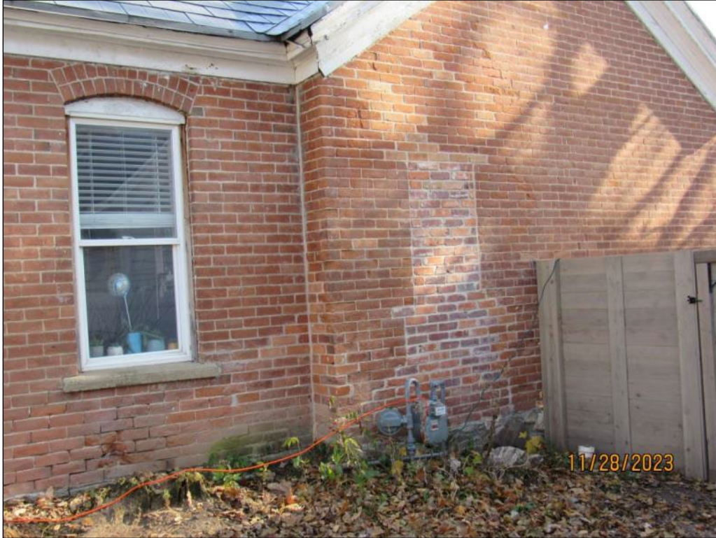
Photograph 9. Exempted doorway or window opening in brick addition; camera facing southeast
