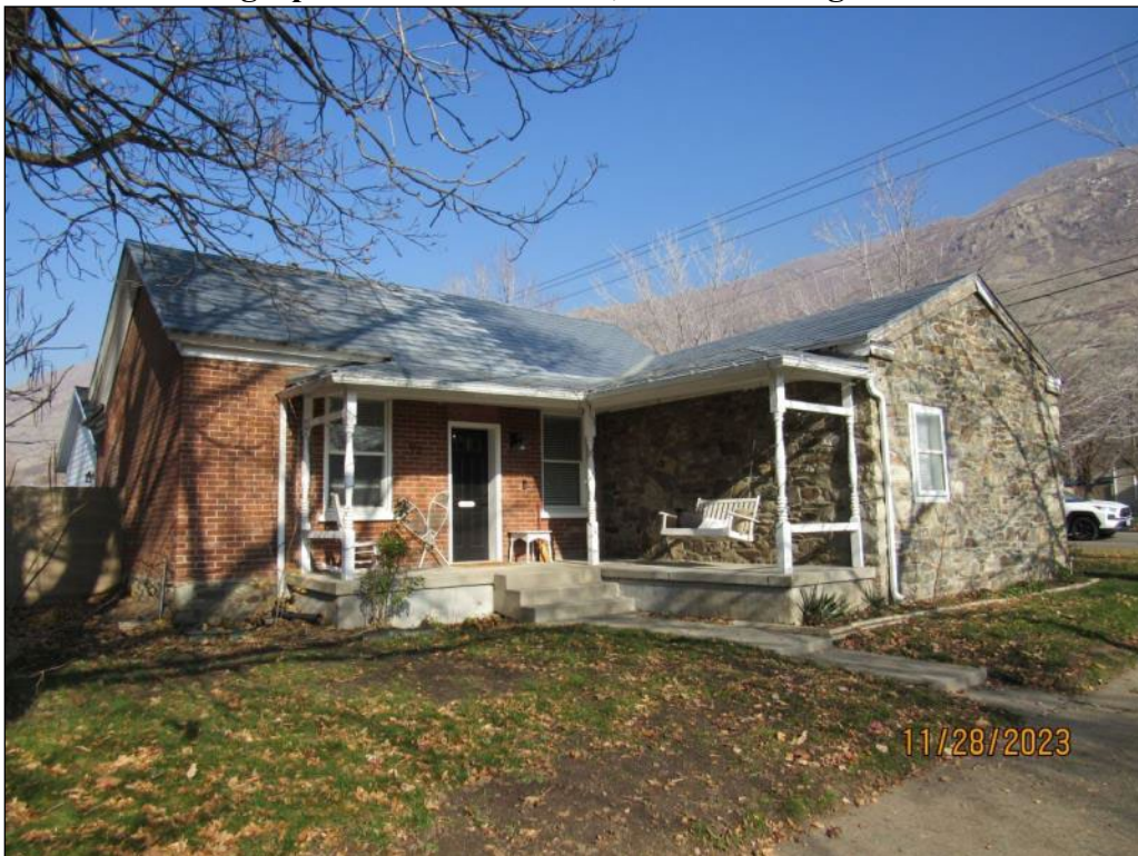
Photograph 4. South elevation; camera facing northeast
