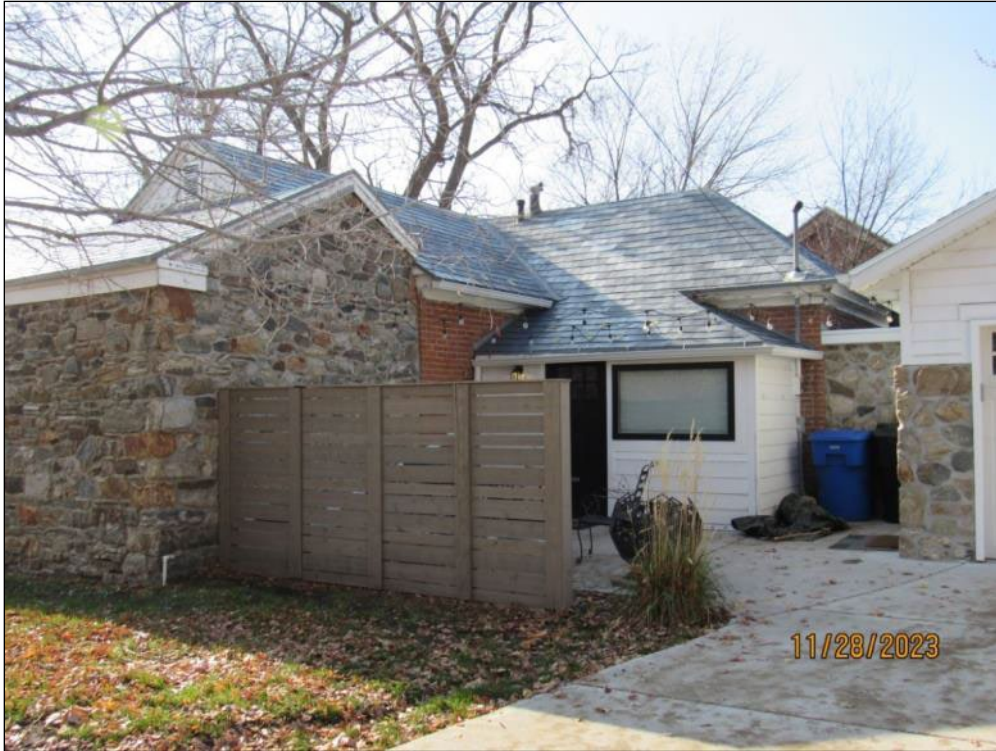
Photograph 7. North elevation; camera facing southwest
