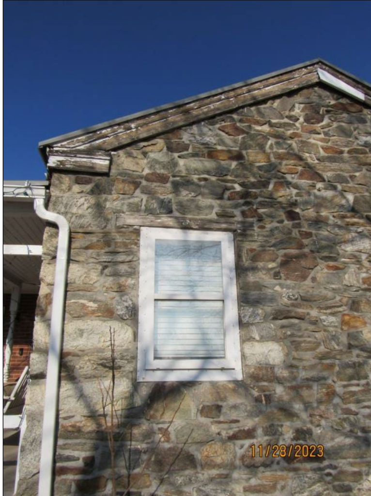
Photograph 10. Window and raking molding detail on south elevation of stone section; camera facing north
