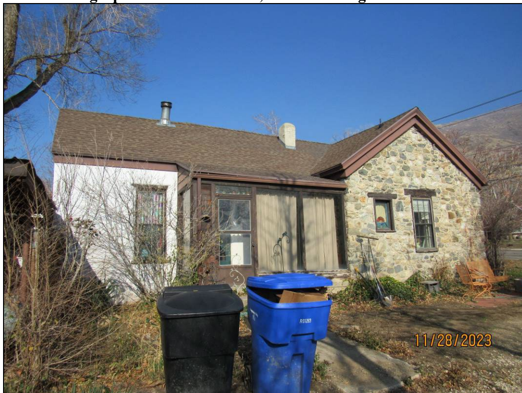
Photograph 7. South elevation; camera facing north-northeast
