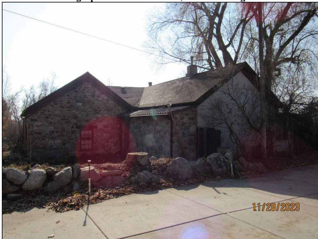
Photograph 5. North elevation; camera facing south
