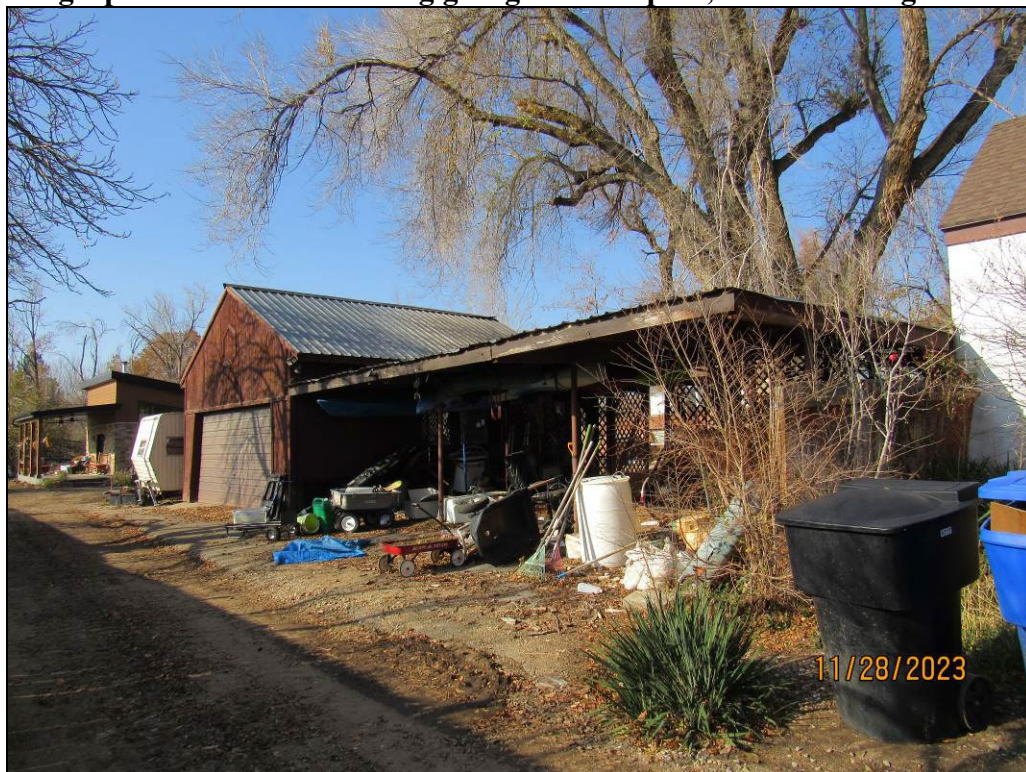
Photograph 11. Non-contributing garage and carport; camera facing northwest
