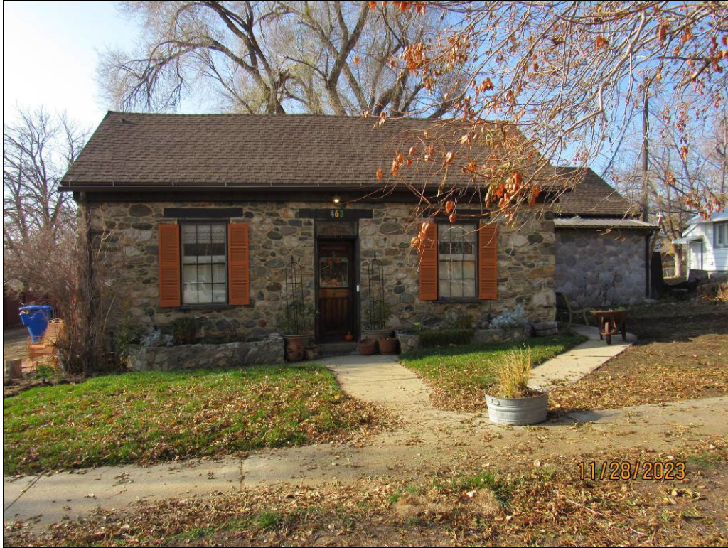
Photograph 3. East elevation; camera facing west
