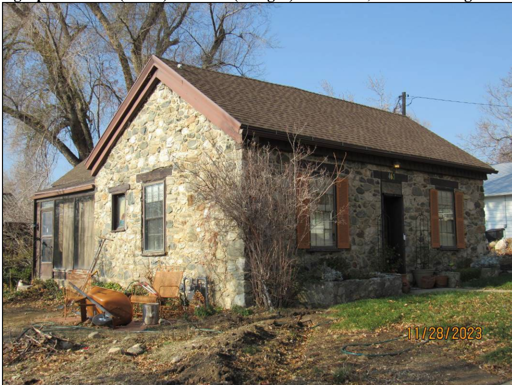
Photograph 2. South (at left) and east (at right) elevations; camera facing northwest
