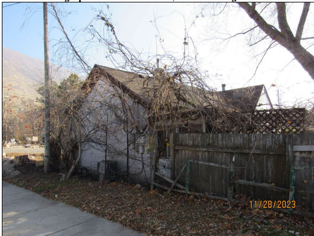
Photograph 10. North elevation; camera facing southeast
