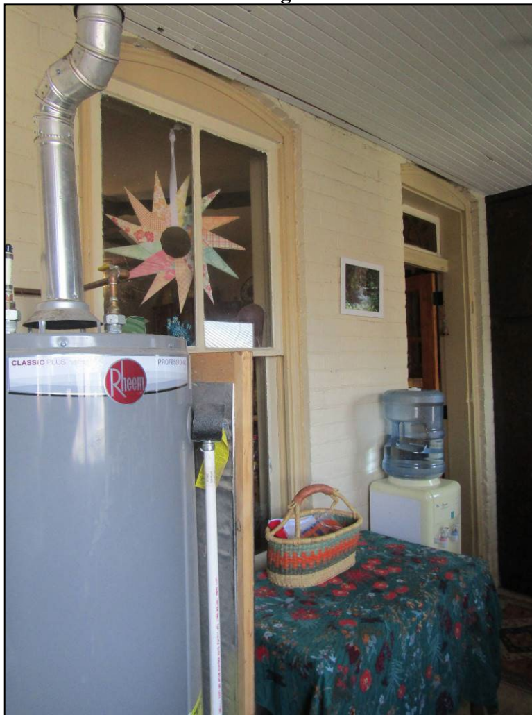
Photograph 15. Original brick wall from rear addition enclosed in second addition; camera facing southeast
