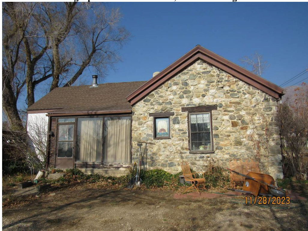
Photograph 6. South elevation; camera facing north
