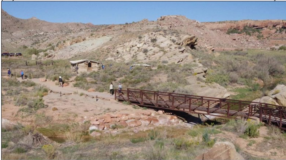
Fig. 20. The same location and angle in 2021 (Steely) show how Salt Wash changed the drainage channel again in 2006 farther west toward the buildings, requiring a new segment of the Pedestrian Bridge in 2007, including stone rip-rap beneath, to carry Delicate Arch Trail across the wash.
