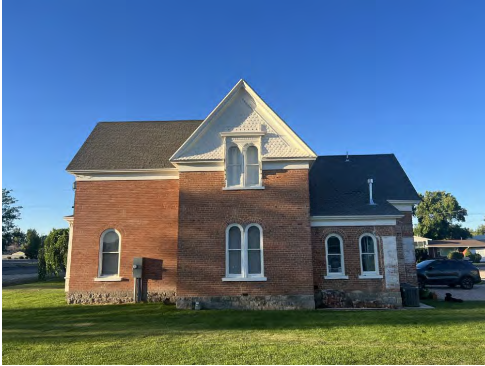
Photo 3 of 16. North elevation. Camera facing south.
