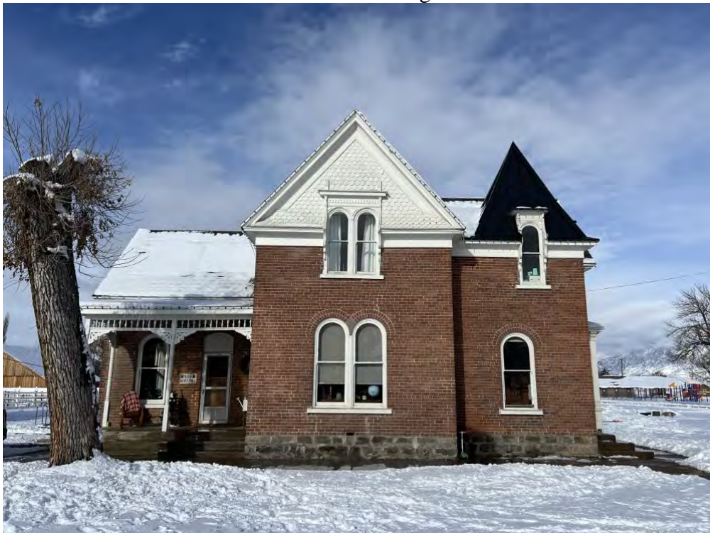
Photo 2 of 16. South elevation. Camera facing north.
