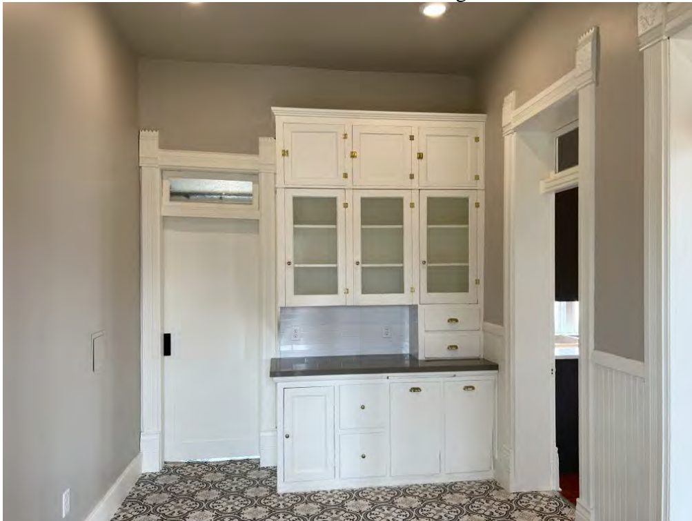
Photo 6 of 16. Main floor mudroom. Camera facing north.
