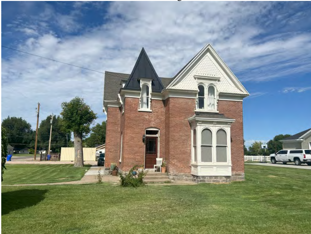
Photo 4 of 16. East elevation. Camera facing west.
