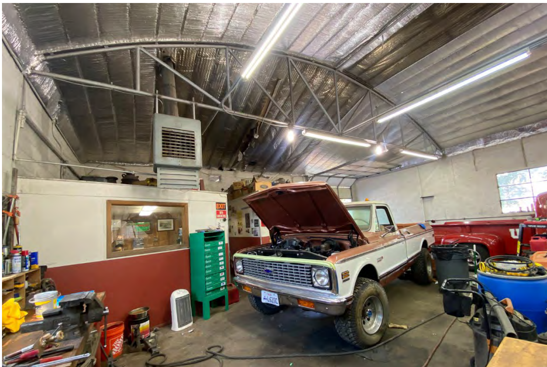
Photograph 17 Interior, workshop office and trusswork. Camera facing northwest.
