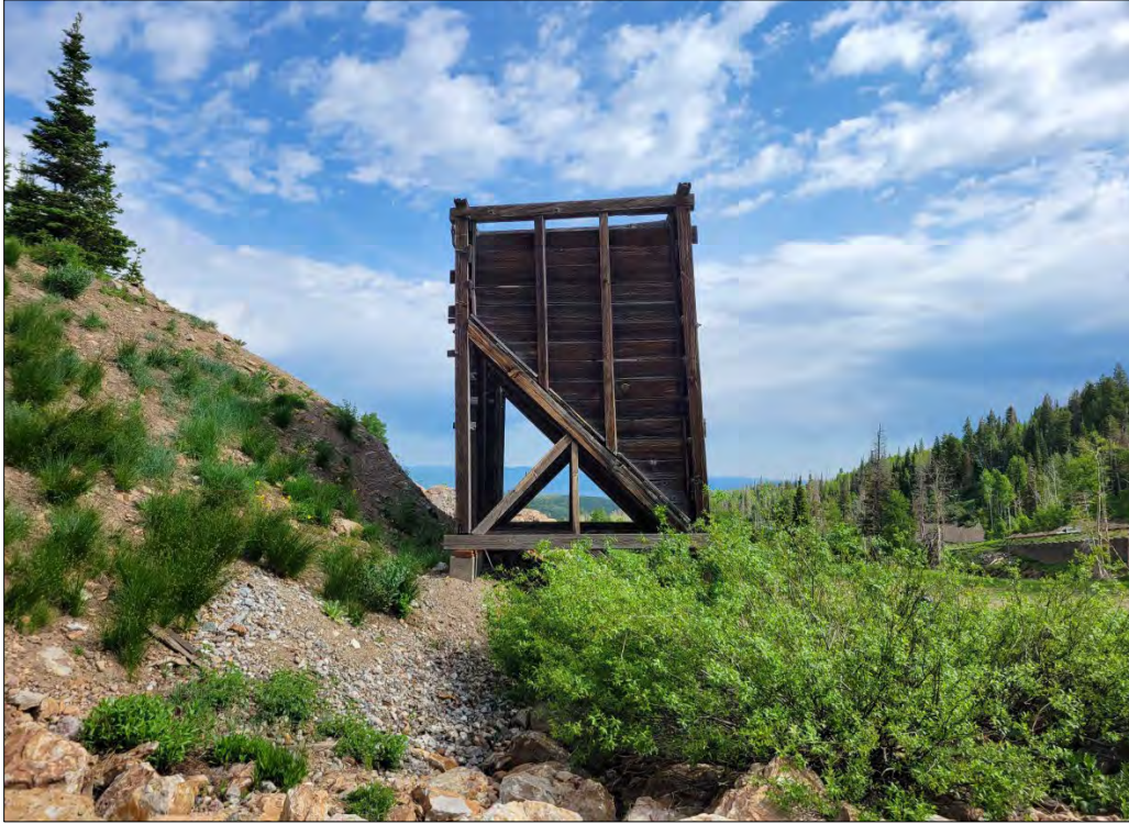
Photo No. 6 South elevation of ore bin. Camera facing north.
