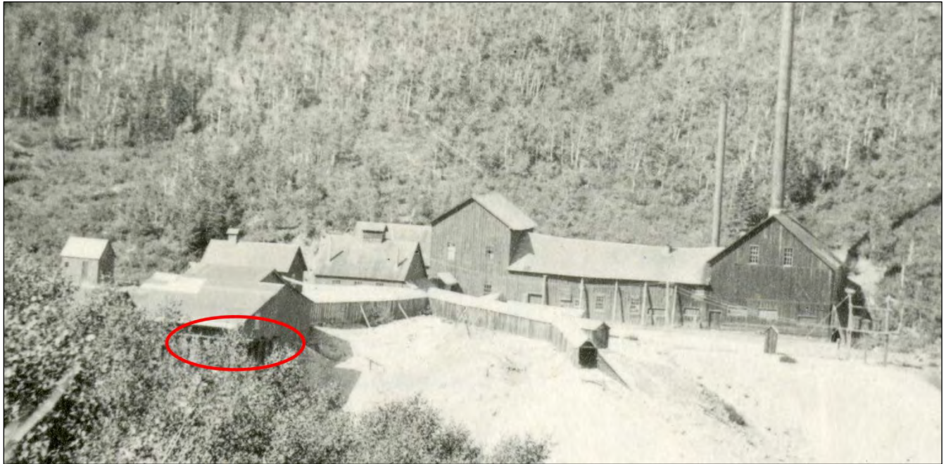
Figure 2. Little Bell surface plant c.1907. (Top of ore bin circled.) Image courtesy Park City Historical Society.
