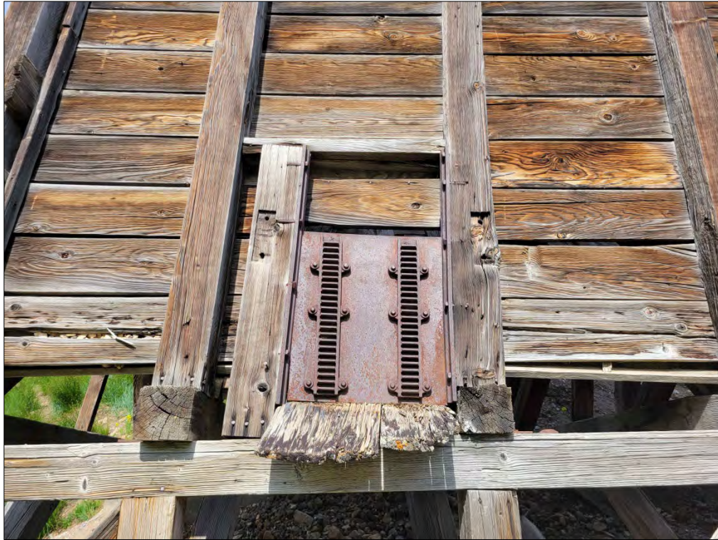
Photo No. 4 Detail of cast-iron chute (gate) doors. Camera facing west.
