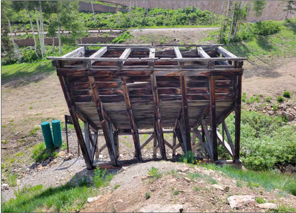
Photo No. 10 West (rear) elevation. Camera facing east.
