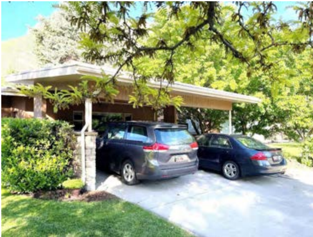
Photo 6 of 25, Carport, Facing Southeast
