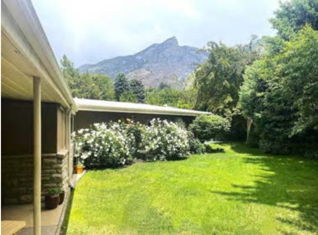
Photo 9 of 25, Rear/south and east elevations, Facing northeast
