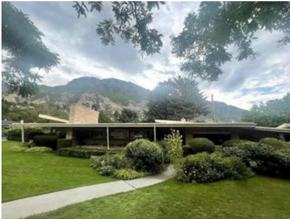
Photo 2 of 25, Façade/west elevation, Facing Northeast
