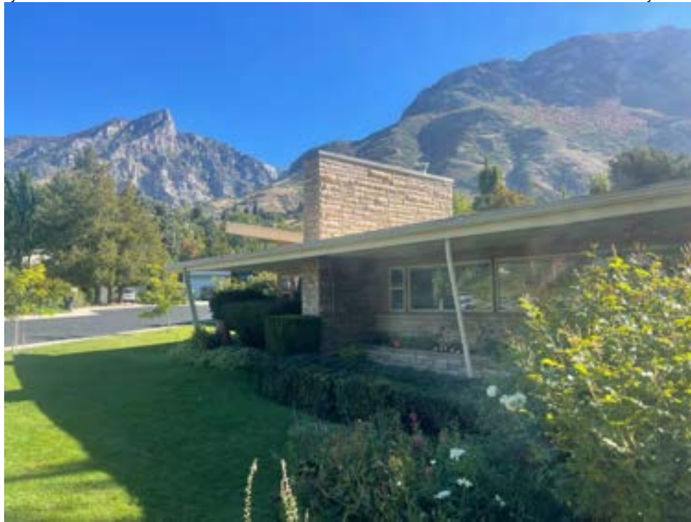
Photo 3 of 25, Chimney and west elevation, June 2023, Facing Northeast
