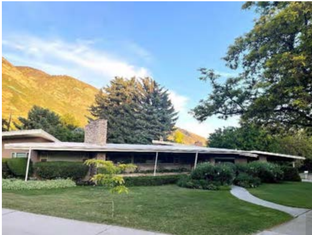
Photo 4 of 25, Façade/west elevation, Facing Southeast
