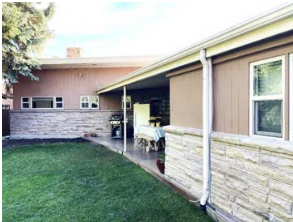
Photo 8 of 25, Rear/south and east elevations, Facing West
