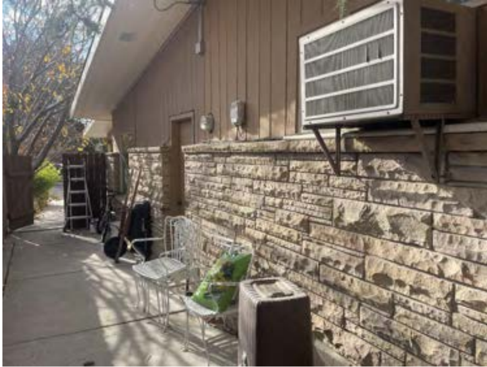
Photo 7 of 25, South Elevation, Facing Southwest
