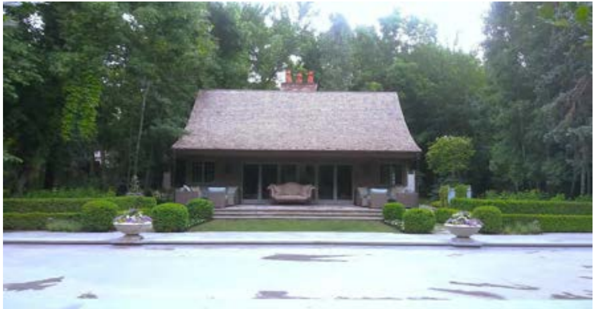
Photo 42 of 46. Pool and Guest House, 2023. Camera facing south.
