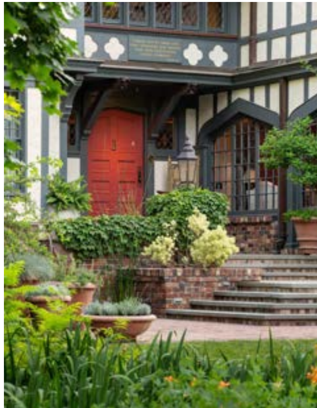
Photo 4 of 46. Entryway on Primary / Northeast Façade, 2013. Camera facing southwest.
