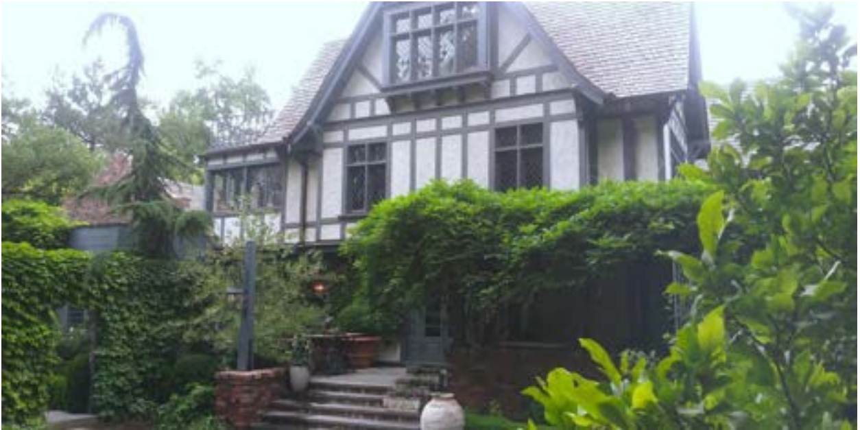
Photo 11 of 46. Northeast Façade (Historic House and Kitchen Addition), 2023. Camera facing southwest.
