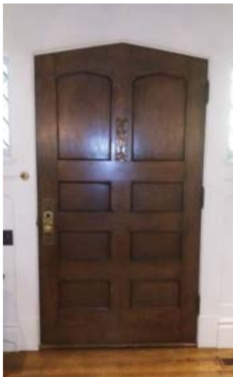
Photo 12 of 46. Primary Entrance Door, c. 2023. Camera facing north.
