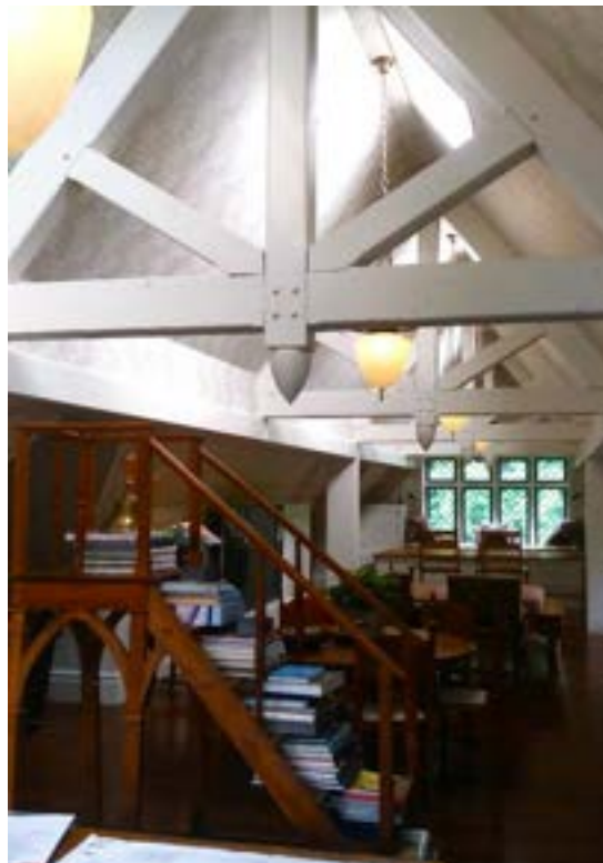
Photo 38 of 46. Third Floor c. 2023. Camer facing southeast.
