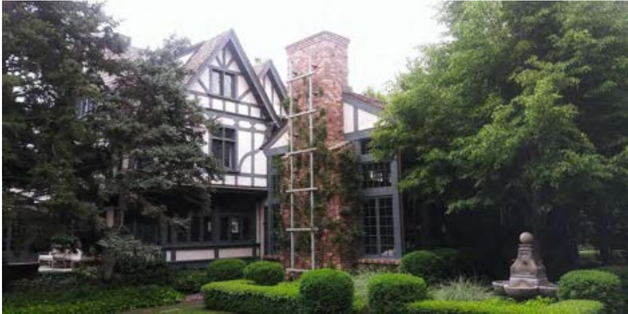
Photo 9 of 46. Southwest Façade (Historic House and Later Kitchen Addition), 2023. Camera facing northeast.
