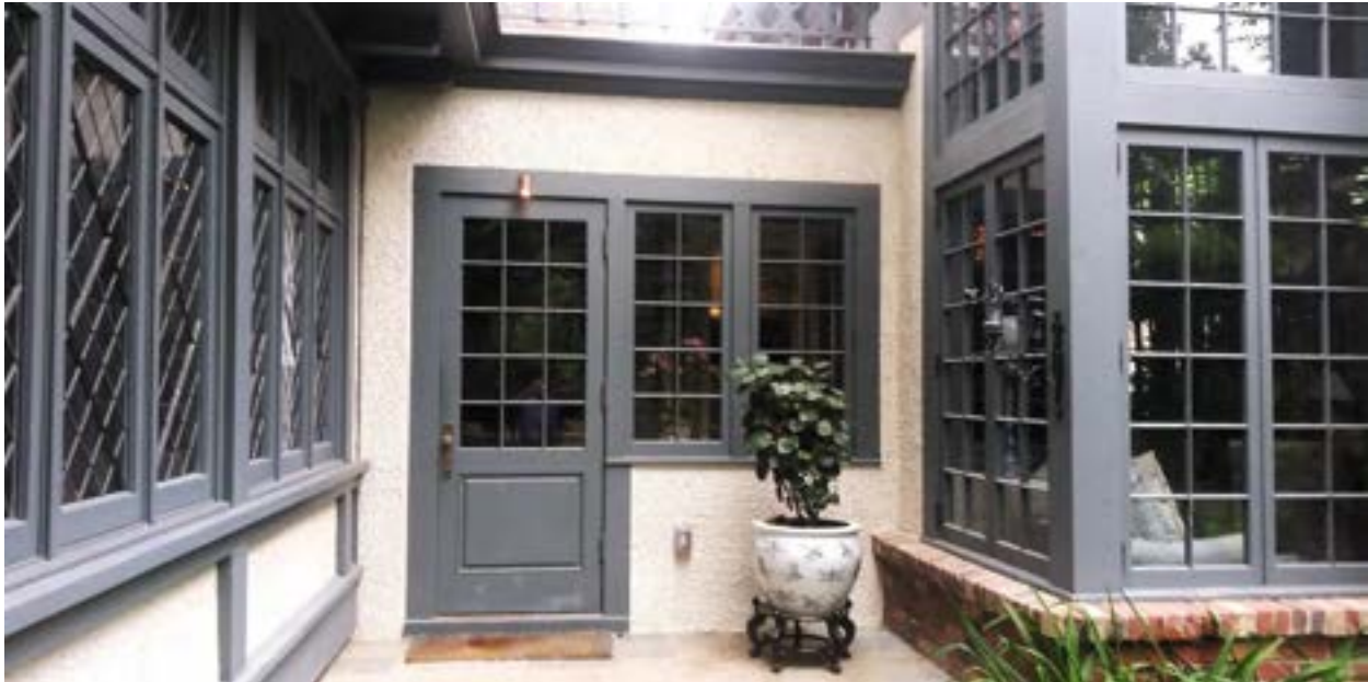
Photo 8 of 46. Southeast Façade (Passage Between Historic House and Kitchen Addition), 2023. Camera facing northeast.
