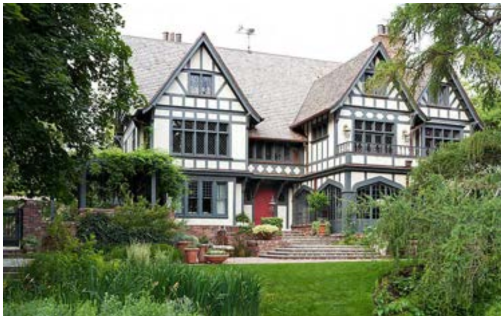
Photo 2 of 46. Primary / Northeast Façade, c. 2015. Camera facing southwest.
