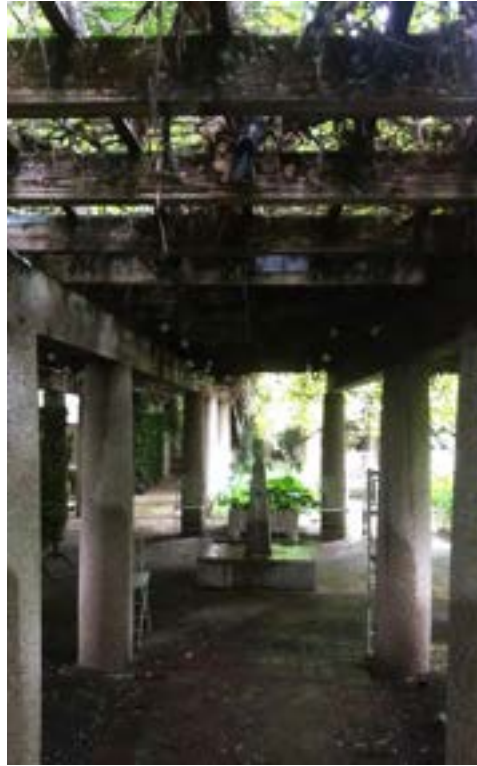
Photo 45 of 46. Pergola and Fountain, 2023. Camera facing east.
