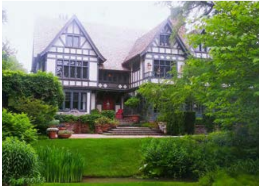
Photo 1 of 46. Northeast Façade, 2023. Camera facing southwest.
