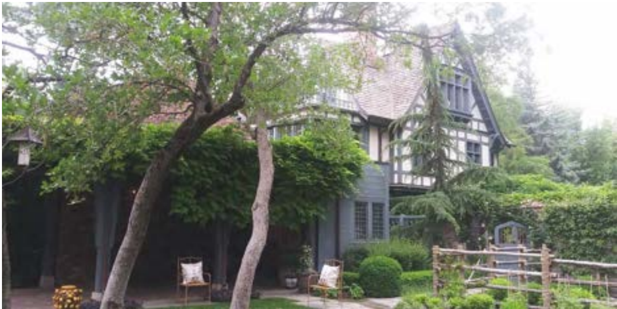
Photo 10 of 46. Northeast Façade (Historic House and Later Kitchen Addition), 2023. Camera facing northwest.
