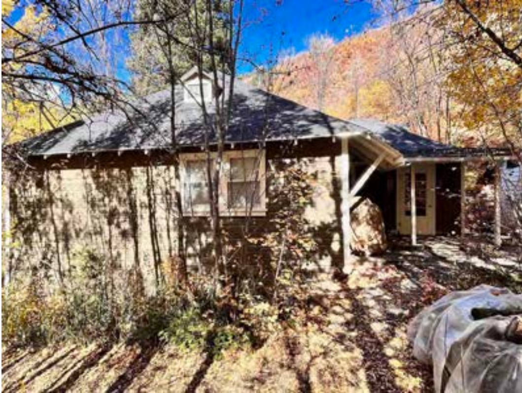
Photograph 33. View of cabin 90 (Contributing). Camera view north.
