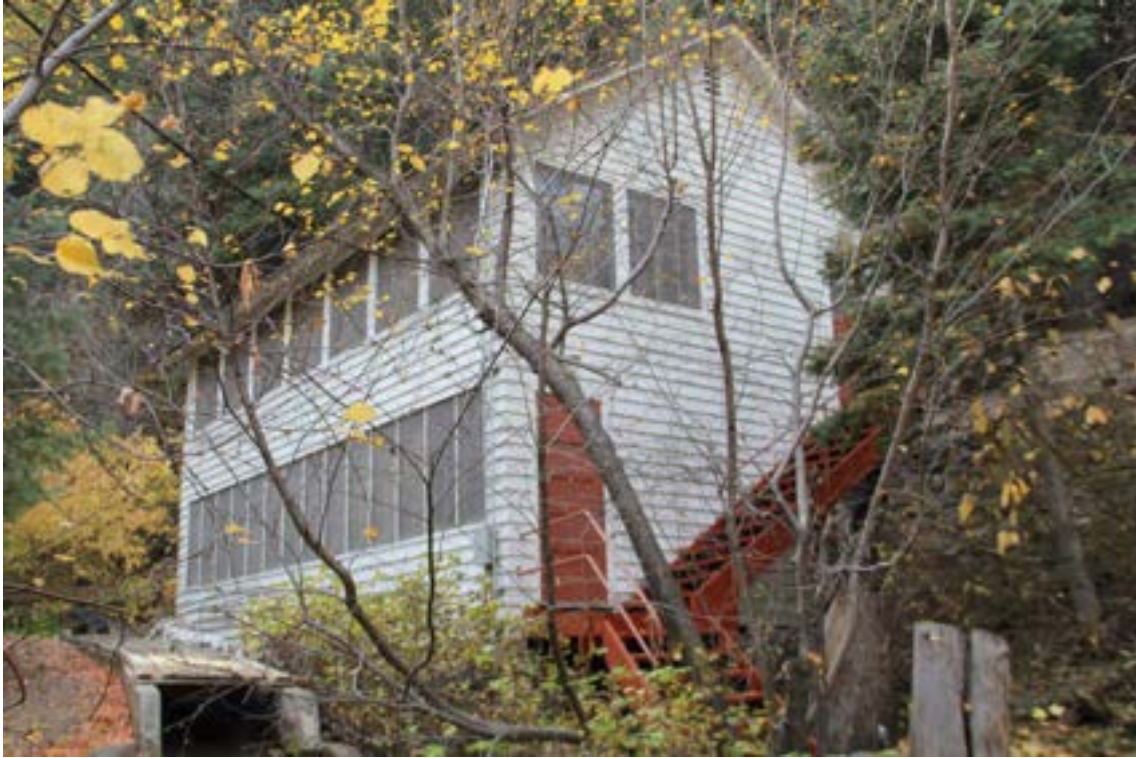
Photograph 21. View of cabin 52 (Contributing). Camera facing southeast.
