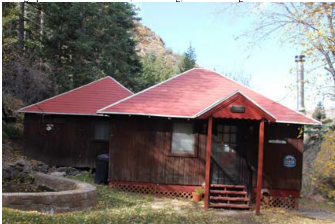
Photograph 20. View of cabin 50 (Contributing). Camera facing northwest.
