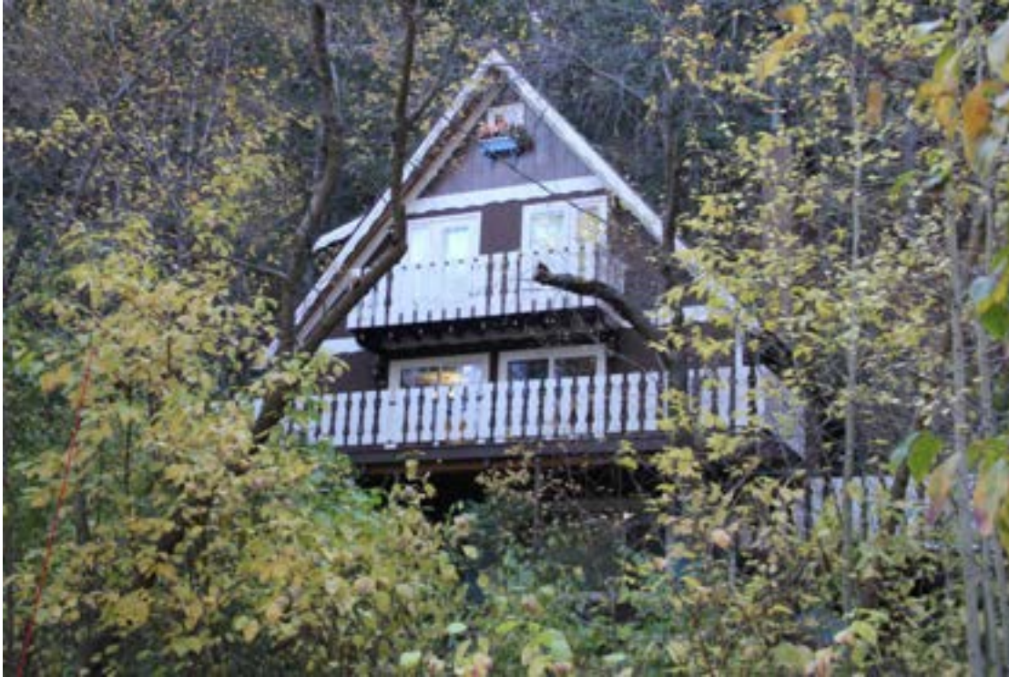
Photograph 31. View of cabin 84 (Contributing). Camera view south.
