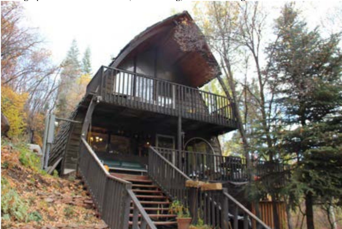
Photograph 8. View of cabin 22 (Contributing). Camera facing northwest.
