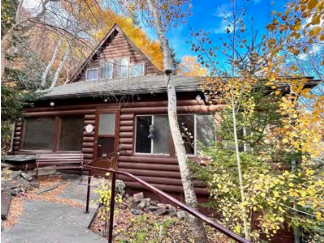
Photograph 13. View of cabin 37 (Contributing). Camera facing northwest.
