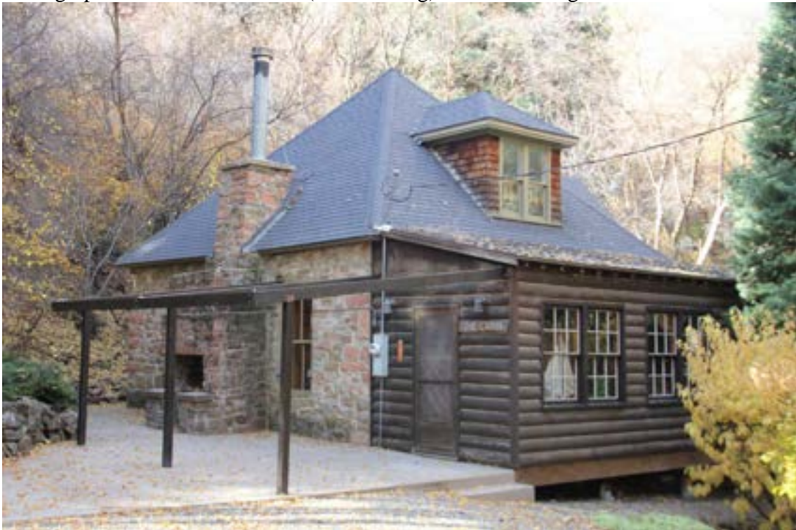
Photograph 16. View of cabin 42 (Contributing). Camera facing northwest.
