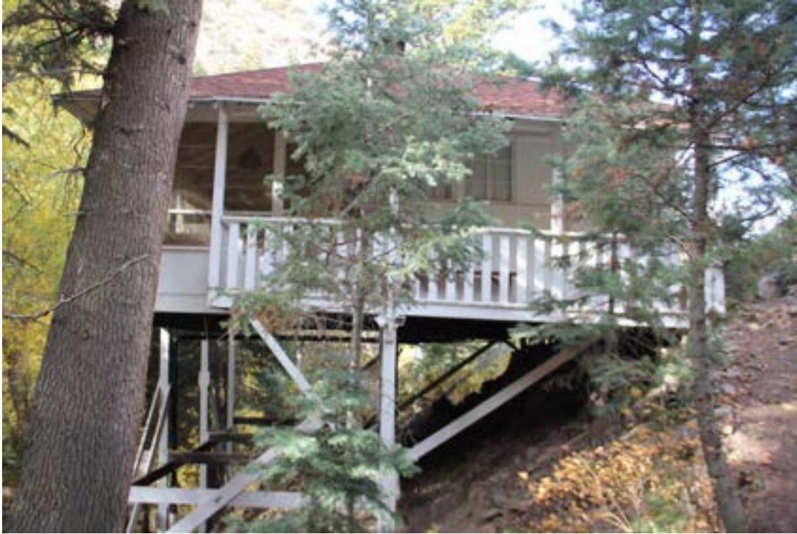
Photograph 23. View of cabin 55 (Contributing) side façade. Camera view northwest.
