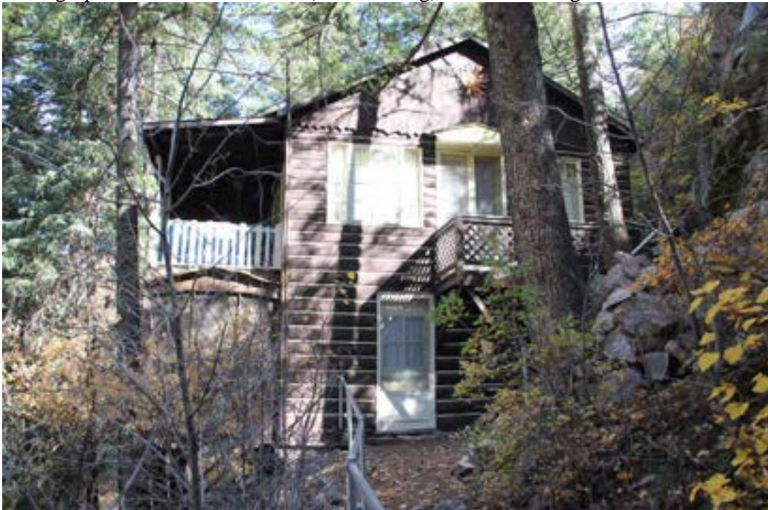
Photograph 28. View of cabin 76 (Contributing). Camera facing west.
