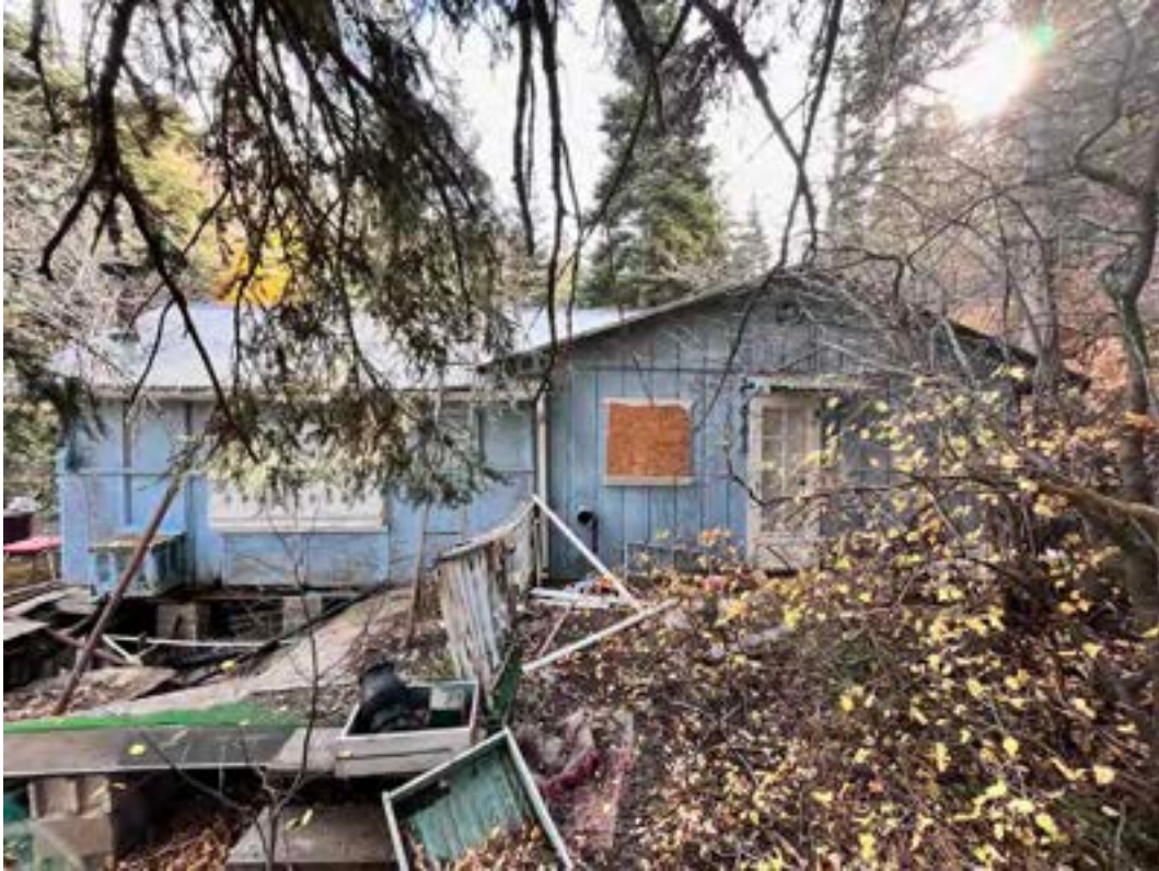
Photograph 17. View of cabin 43 (Contributing). Camera facing
