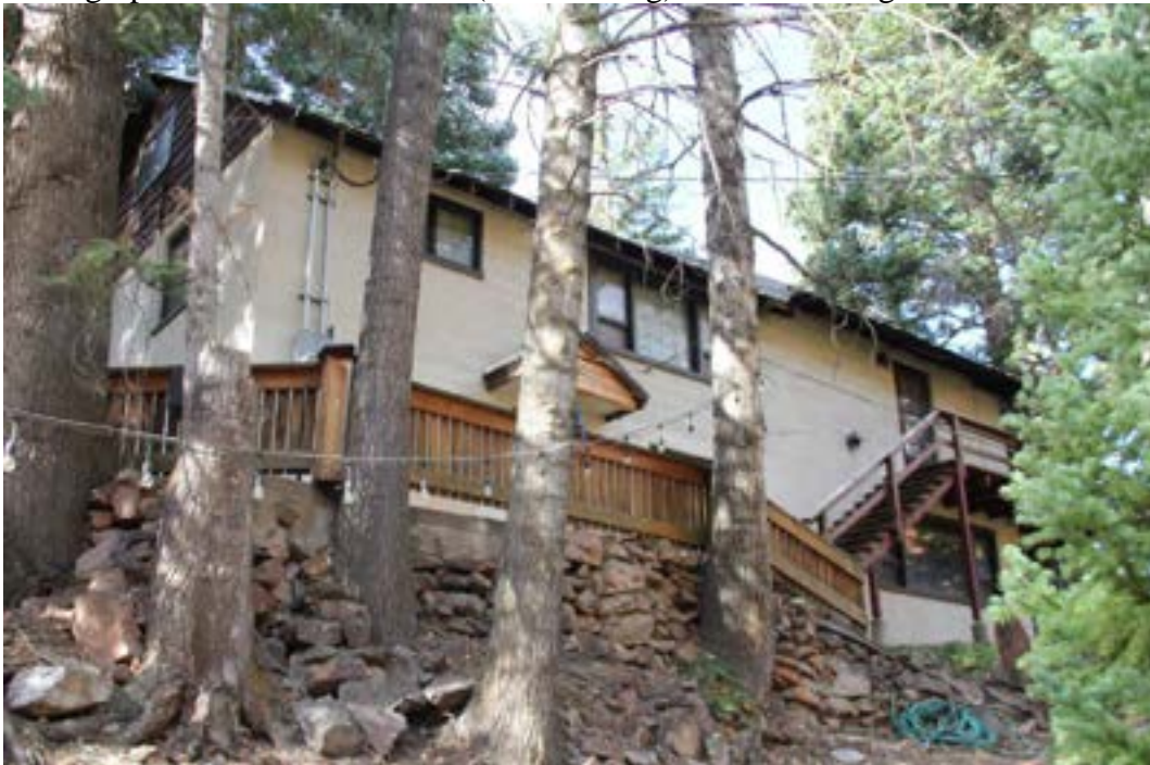
Photograph 18. View of cabin 44 (Contributing). Camera facing northwest.
