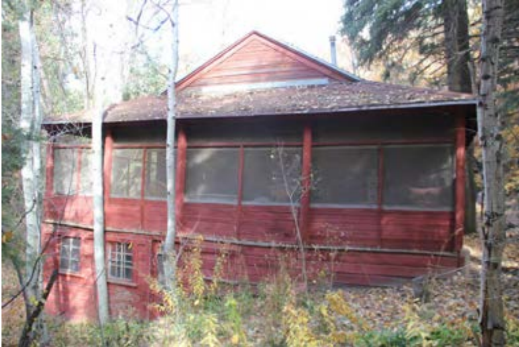
Photograph 25. View of cabin 57 (Contributing). Camera facing northeast.
