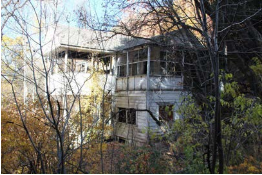
Photograph 27. View of cabin 62 (Contributing). Camera facing northwest.
