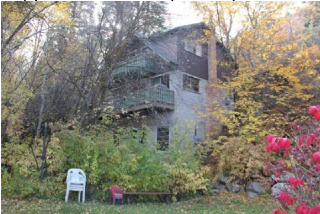
Photograph 12. View of cabin 33 (Contributing). Camera facing southwest.
