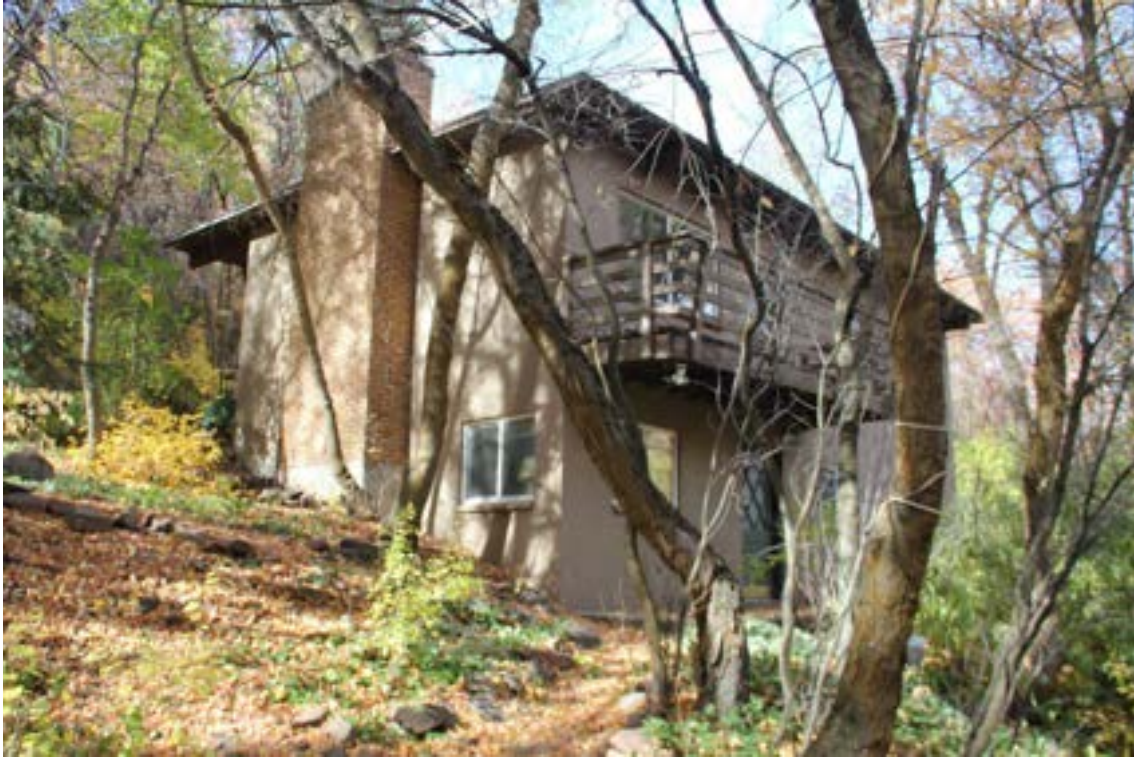
Photograph 15. View of cabin 41 (Contributing). Camera facing northwest.
