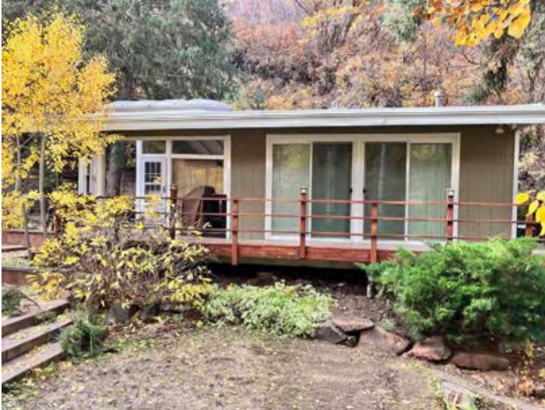
Photograph 9. View of cabin 27 (Contributing). Camera facing southwest.
