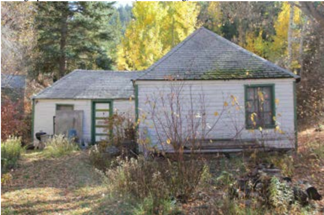
Photograph 34. View of cabin 92 (Contributing). Camera view east.
