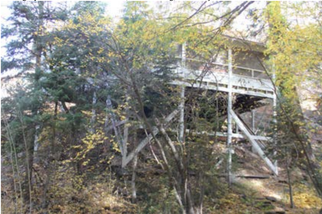
Photograph 22. View of cabin 55 (Contributing) main façade. Camera view northeast.
