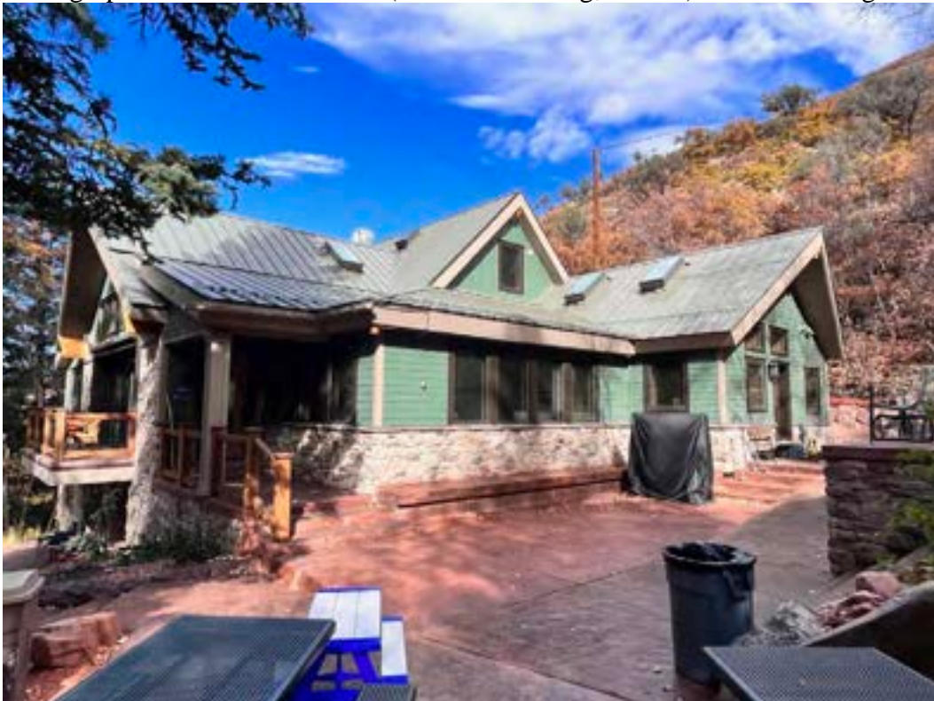
Photograph 26. View of cabin 60 (Non-contributing; altered). Camera facing northwest.
