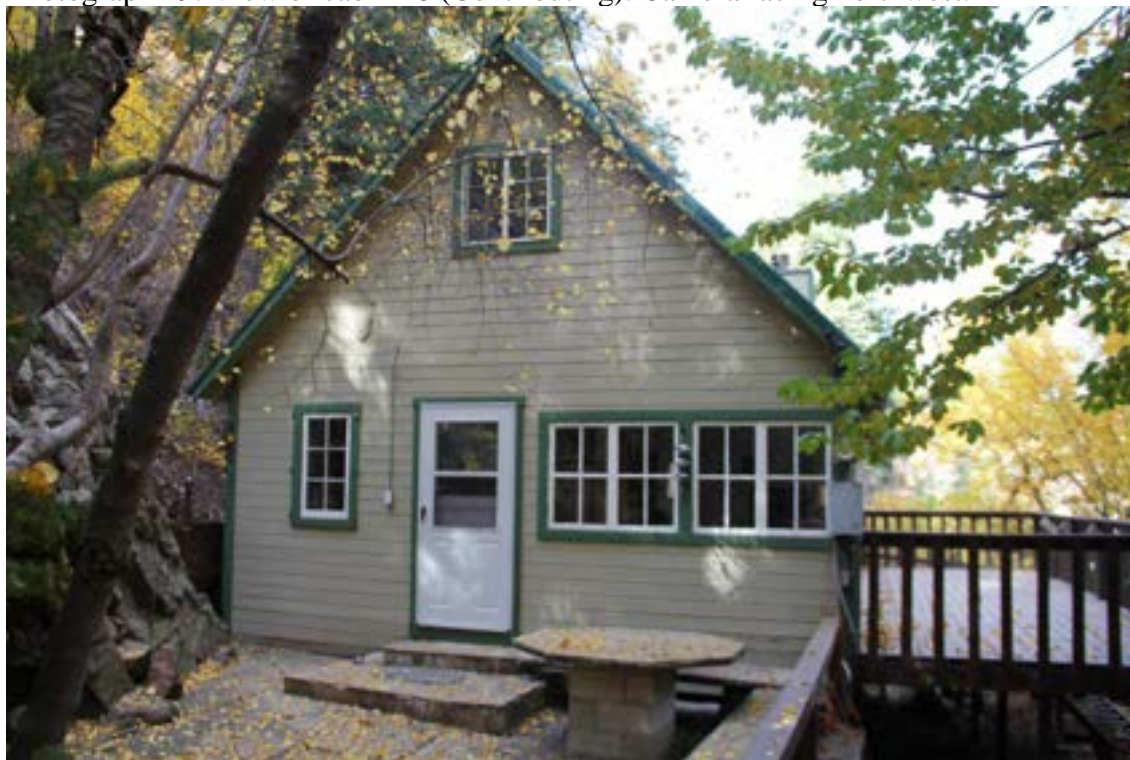
Photograph 19. View of cabin 48 (Contributing). Camera facing northwest.
