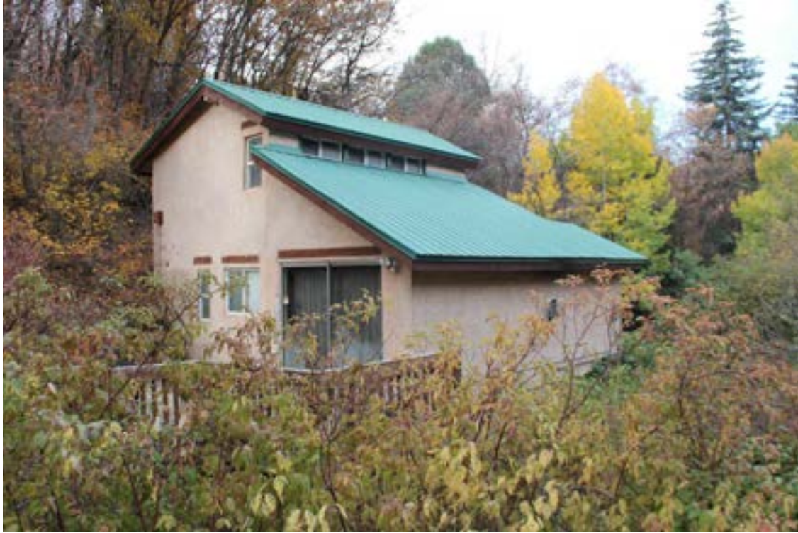
Photograph 7. View of cabin 19 (Non-contributing; altered). Camera facing northwest.
