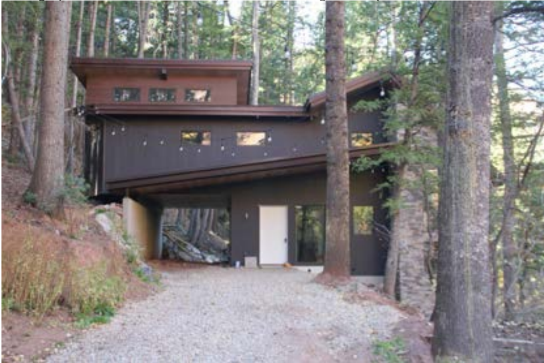
Photograph 32. View of cabin 86 (Non-contributing; out of period). Camera view west.
