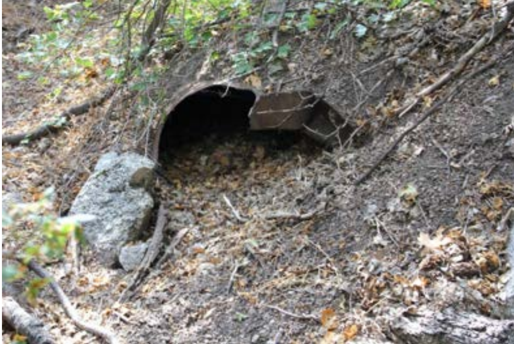
Photograph 9. Remnant of metal pipe adjacent to Pipeline Trail. Camera view west.
