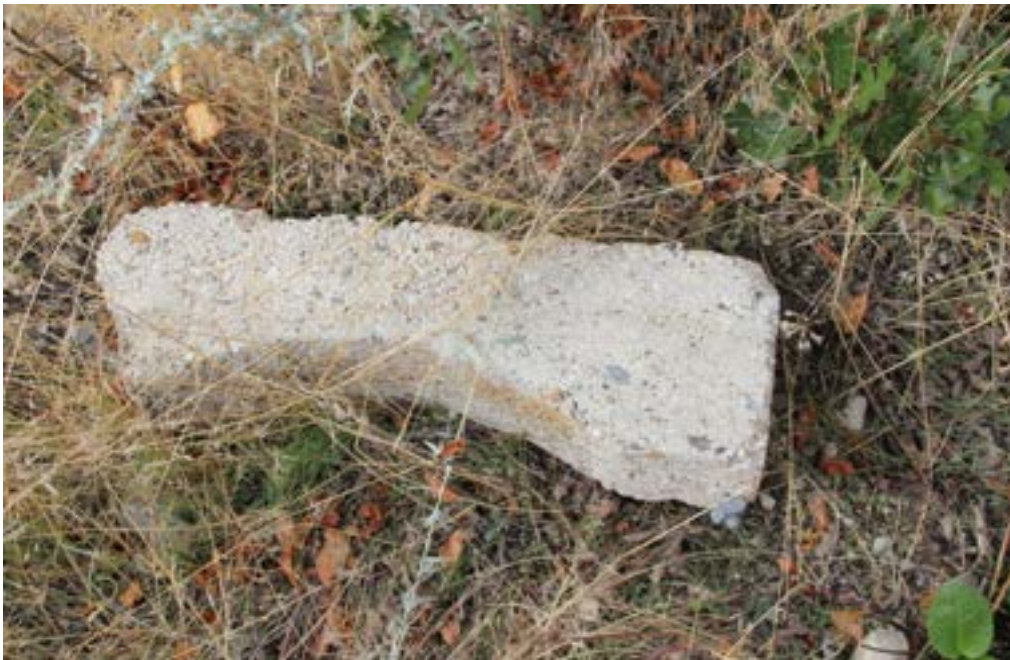
Photograph 8. Concrete block for supporting a pipeline adjacent to the Pipeline Trail. Camera view down.
