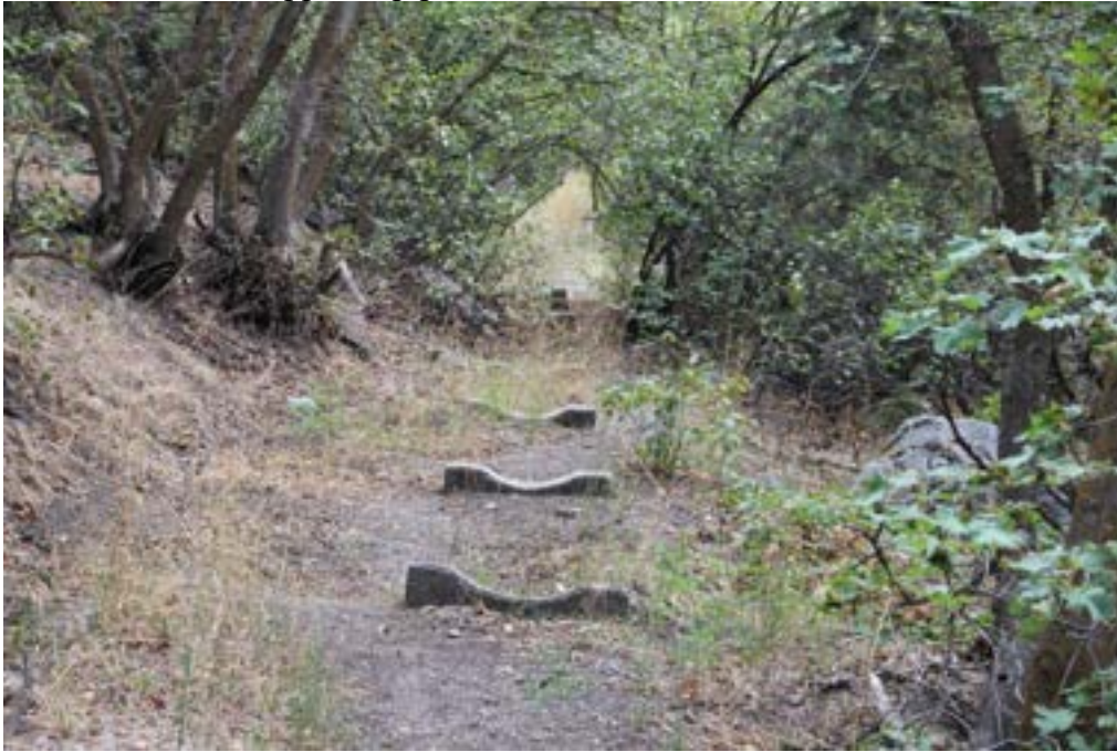
Photograph 7. Alpenbock Loop's Pipeline Trail section near Secret Garden showing concrete blocks formed to support a pipeline. Camera view east.
