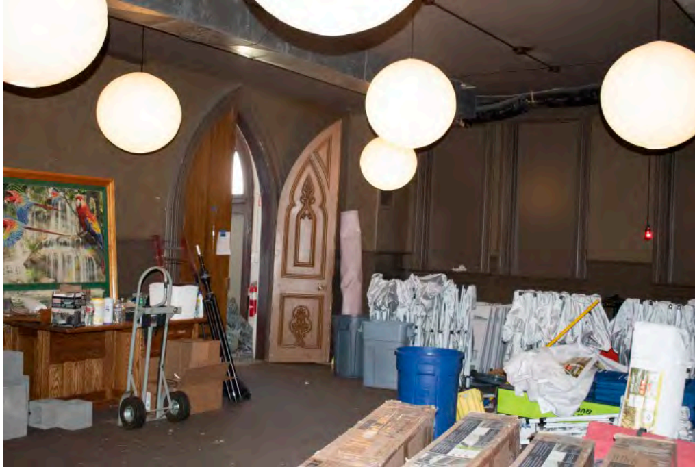
Photograph 17 of 35. Interior, Relief Society Room now used for storage. Camera facing northeast.
