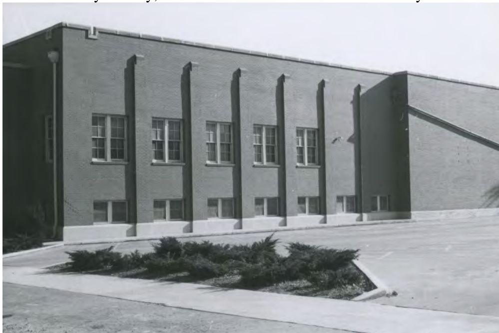
Figure 4 of 5. The 1949 addition as it appeared in the southwest corner after completion. Credit: Church History Library, The Church of Jesus Christ of Latter-day Saints.
