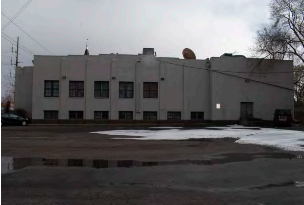
Photograph 10 of 35. Exterior, west elevation of Phase II & III. Camera facing east.
