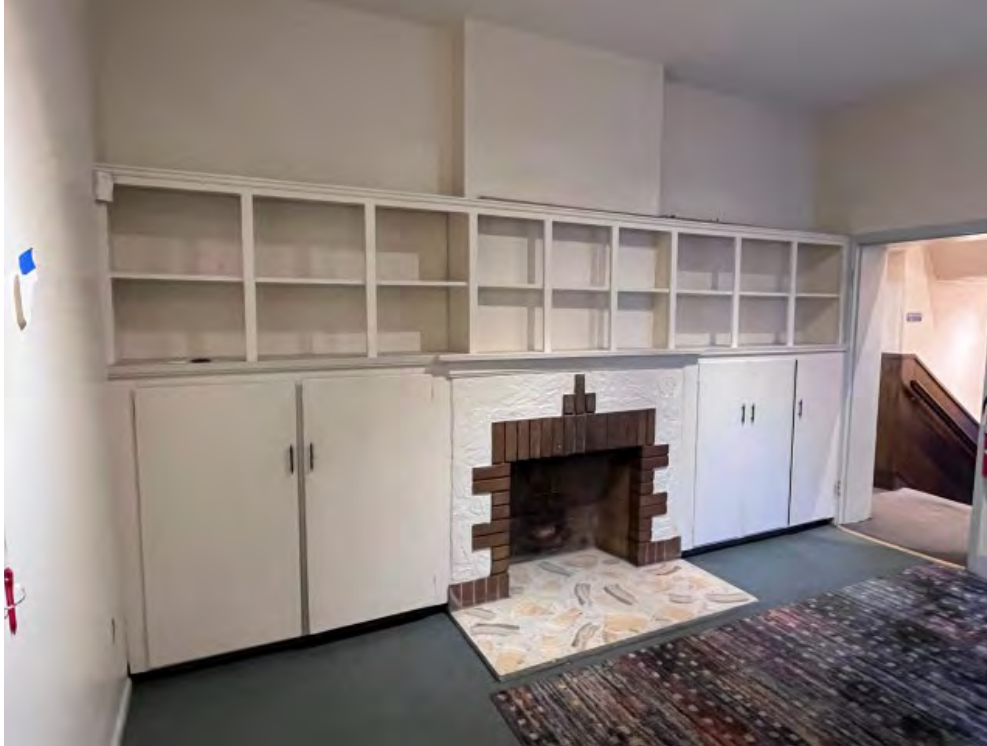
Photograph 25 of 35. Interior, Phase II library and office showing fireplace. Camera facing southwest.
