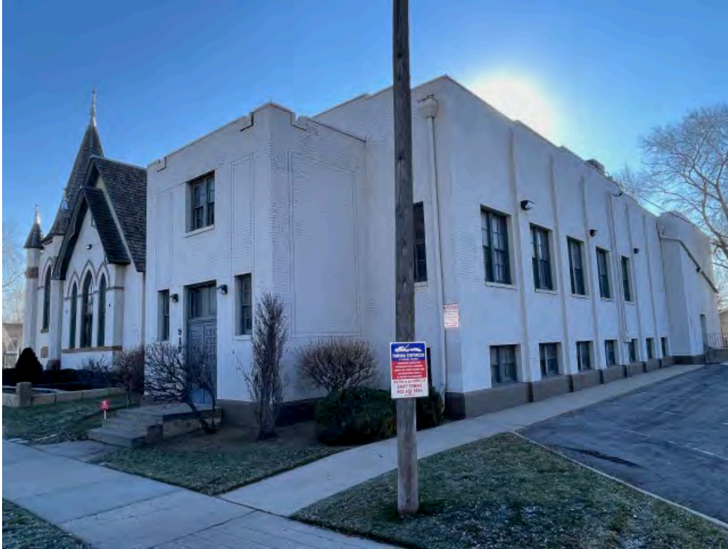
Photograph 3 of 35. Exterior, north elevation (main façade) of Phase I & II and west elevation of Phase II & III. Camera facing southeast.
