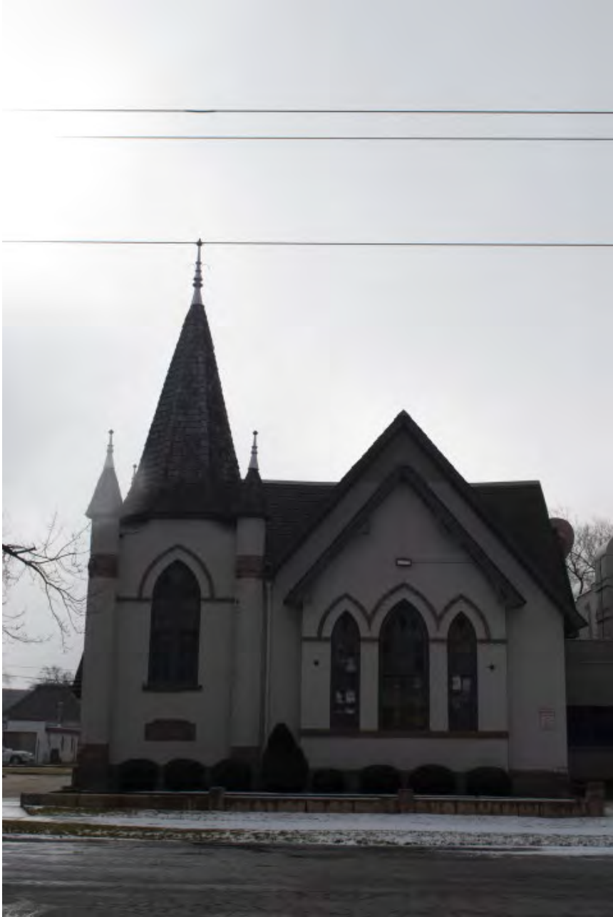
Photograph 7 of 35. Exterior, north elevation of Phase I. Camera facing south.
