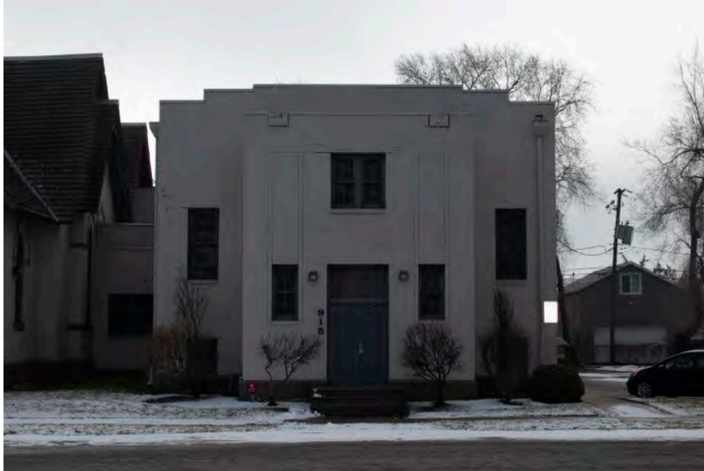
Photograph 9 of 35. Exterior, north elevation of Phase II. Camera facing south.
