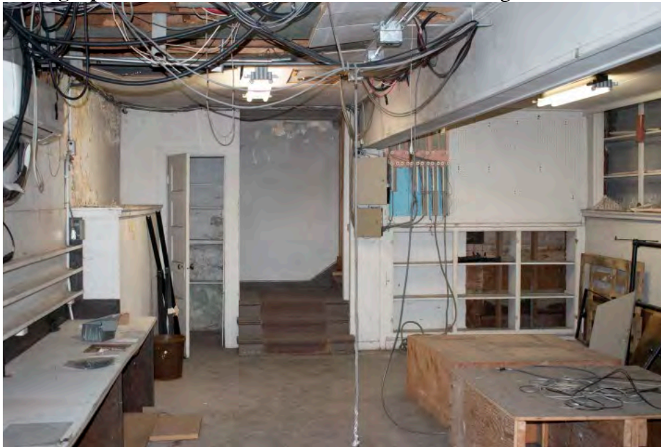
Photograph 34 of 35. Interior, Phase III basement storage room. Camera facing east.
