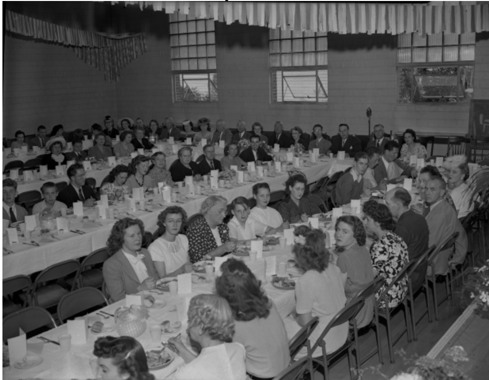
Figure 3 of 5. Banquet for Bishop Quayle in 1946 taking place inside the early gymnasium. Credit: Utah State Historical Society/Utah State Archives.
