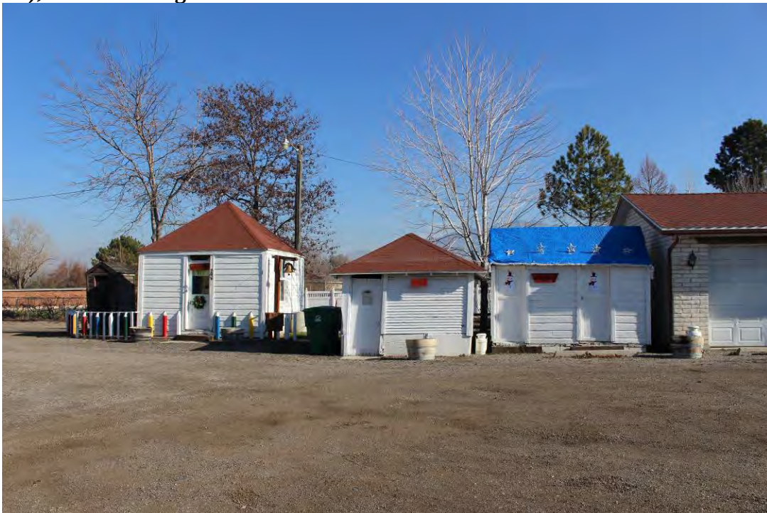
Photograph 14 of 19. Example of non-contributing relocated buildings (except pump house at center); camera facing east
