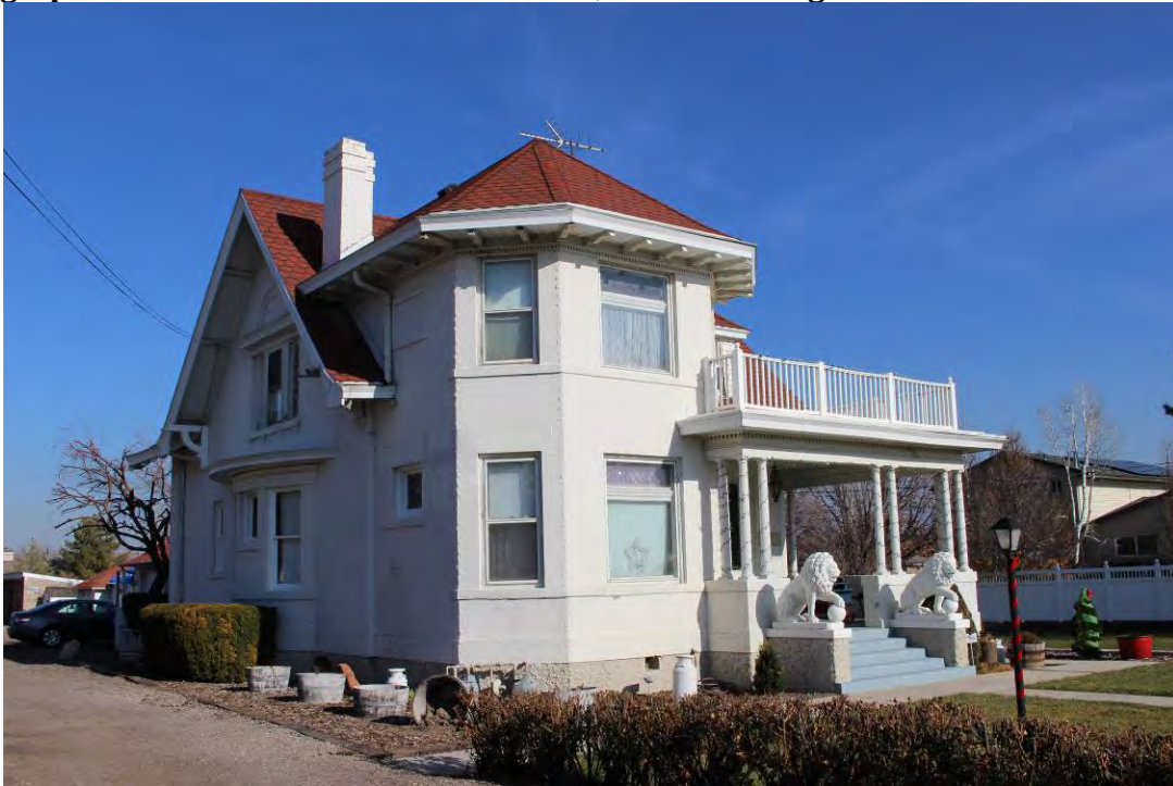
Photograph 3 of 19. South and west elevations; camera facing northeast
