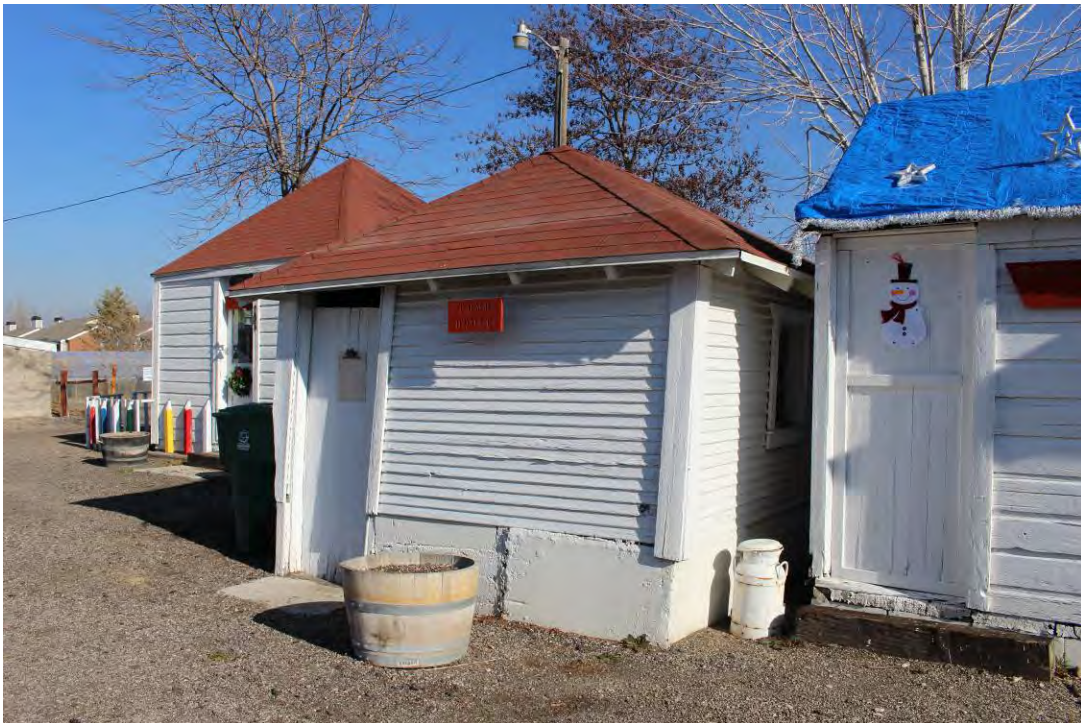
Photograph 12 of 19. Pump house, west and partial south elevations; camera facing northeast
