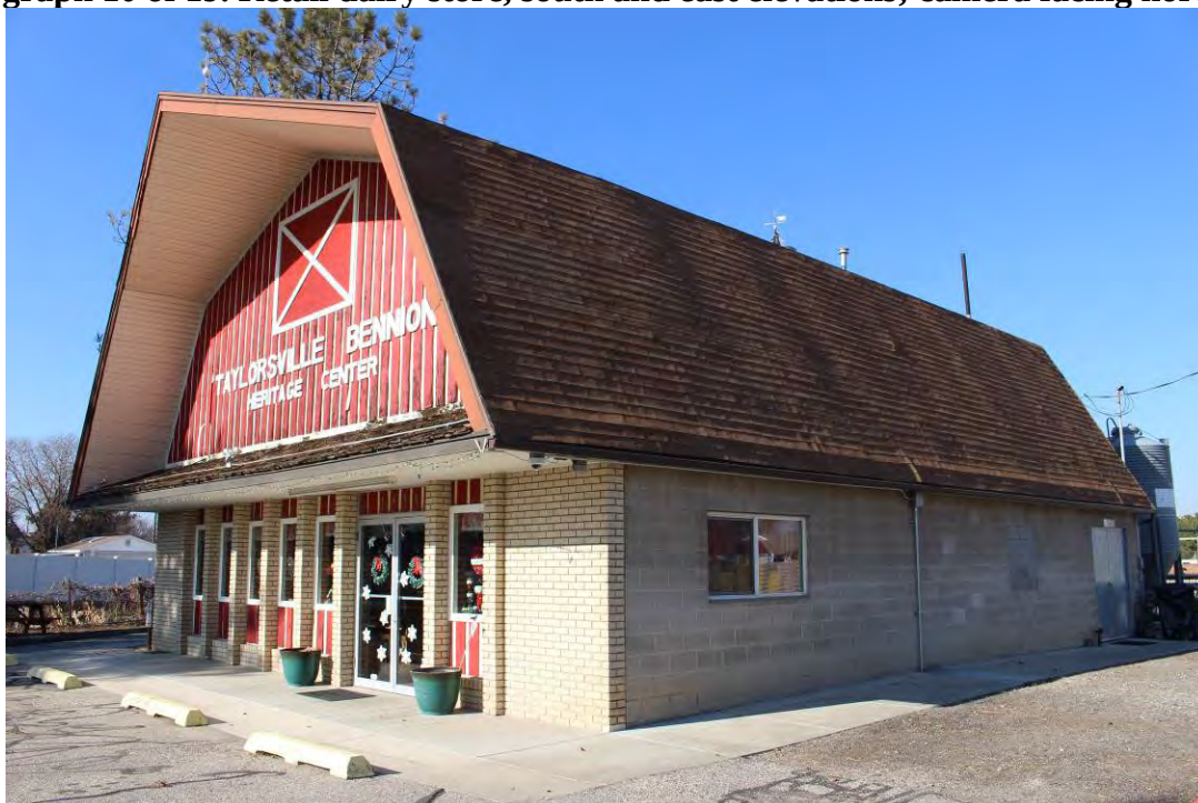
Photograph 10 of 19. Retail dairy store, south and east elevations; camera facing northwest
