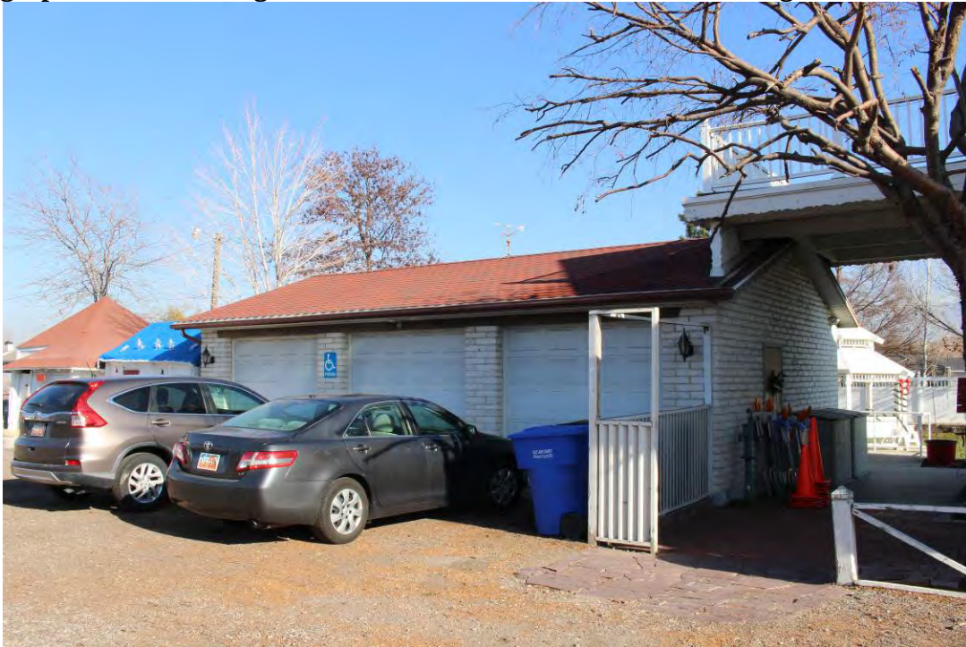
Photograph 15 of 19. Garage, west and south elevations; camera facing northeast
