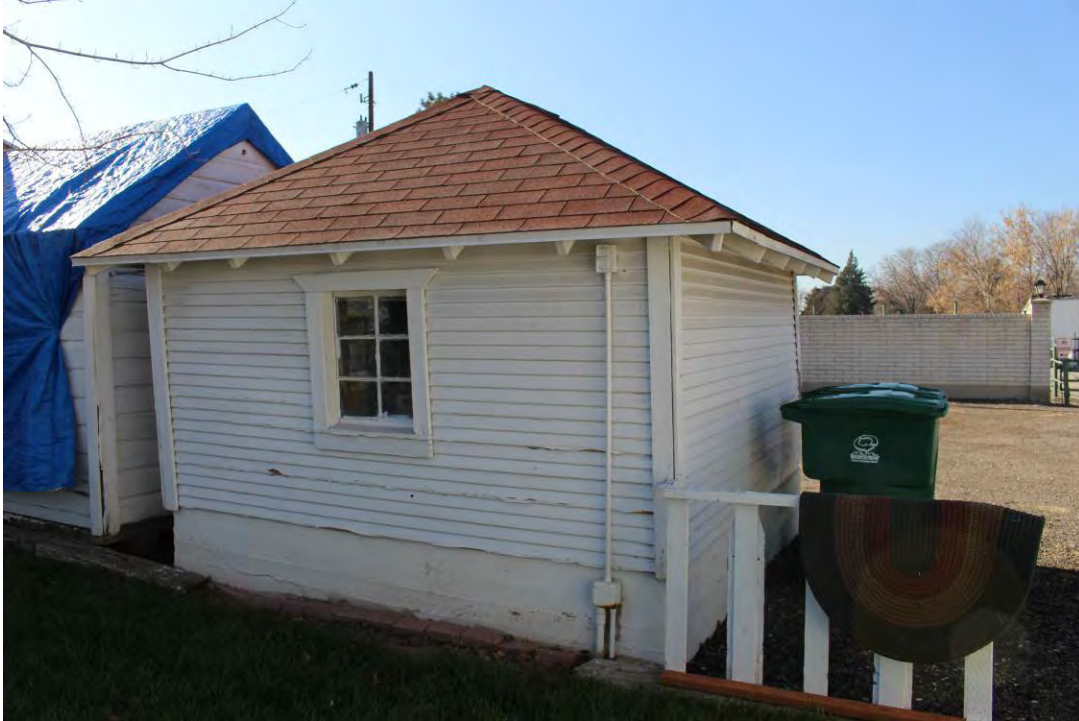
Photograph 13 of 19. Pump house, north and east; camera facing southwest
