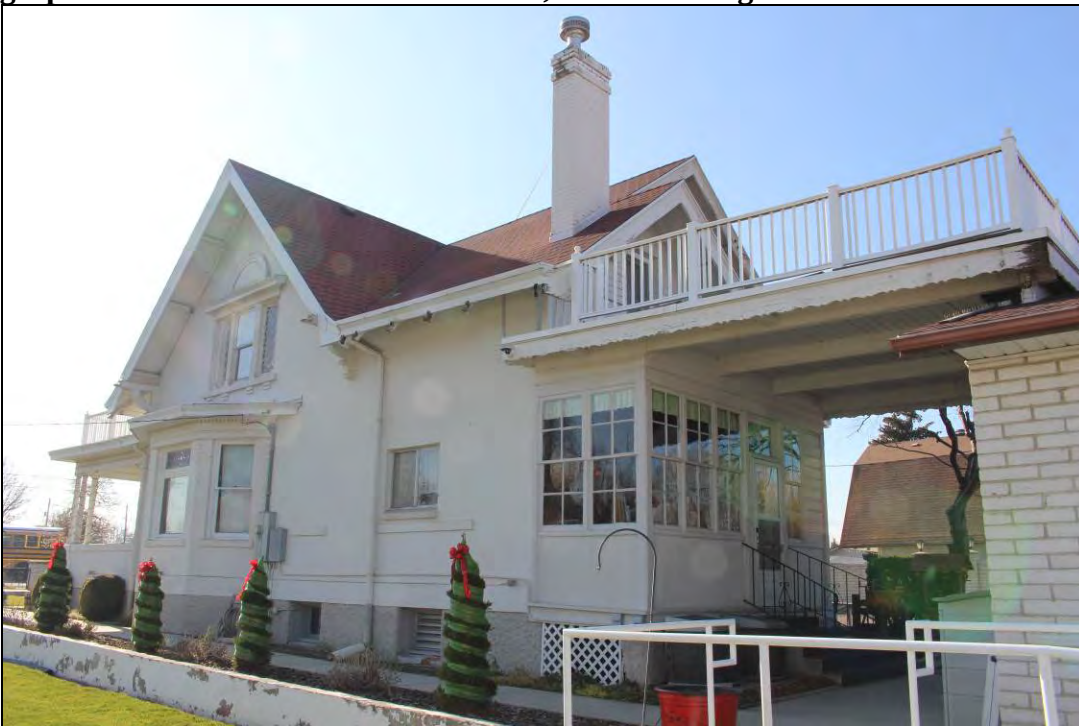
Photograph 4 of 19. North and east elevations; camera facing southwest
