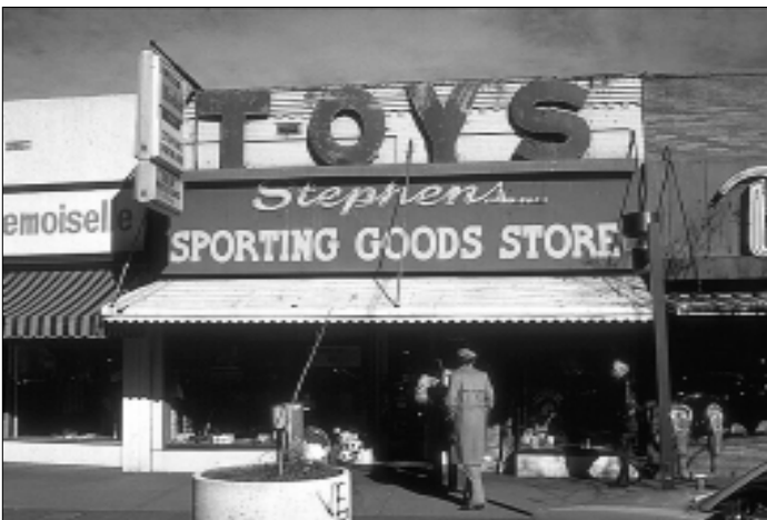
Signs that are out of scale with the facade.
