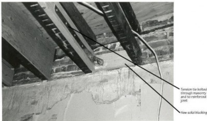
Reinforced Joist/Masonry Wall Connection
